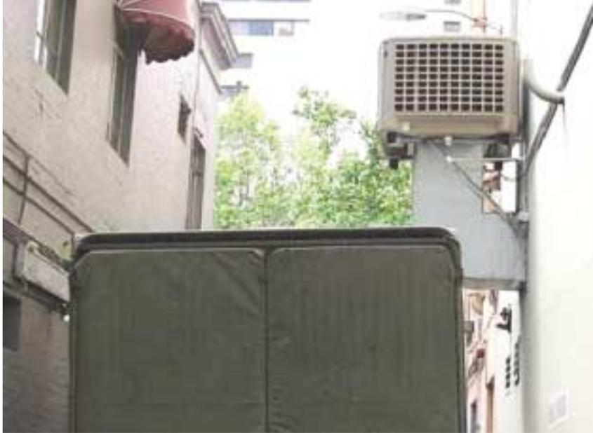
Unplanned, unsightly and unsafe service installations encroaching into the road space. Other problems include noise and dripping water from these installations.
