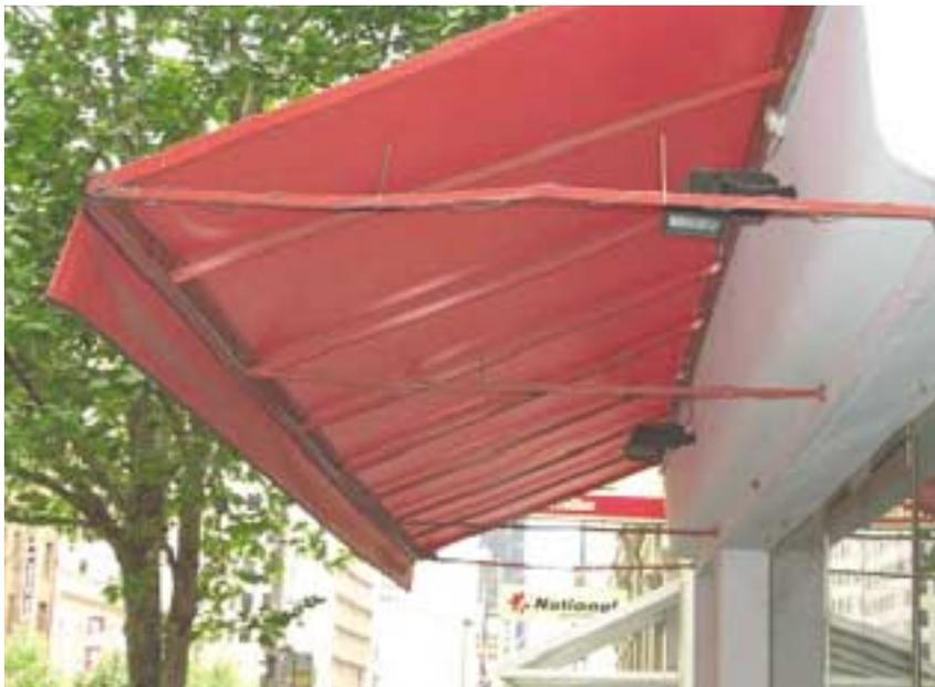
Barbed wire treatment to protect an inadequately designed awning strut.
