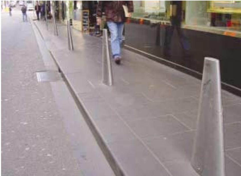
Bollards used to delineate between pedestrian and vehicle zones where parking on the kerb can be an issue.
