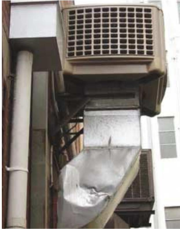
Damaged ductwork due to inadequate vehicular clearance.
