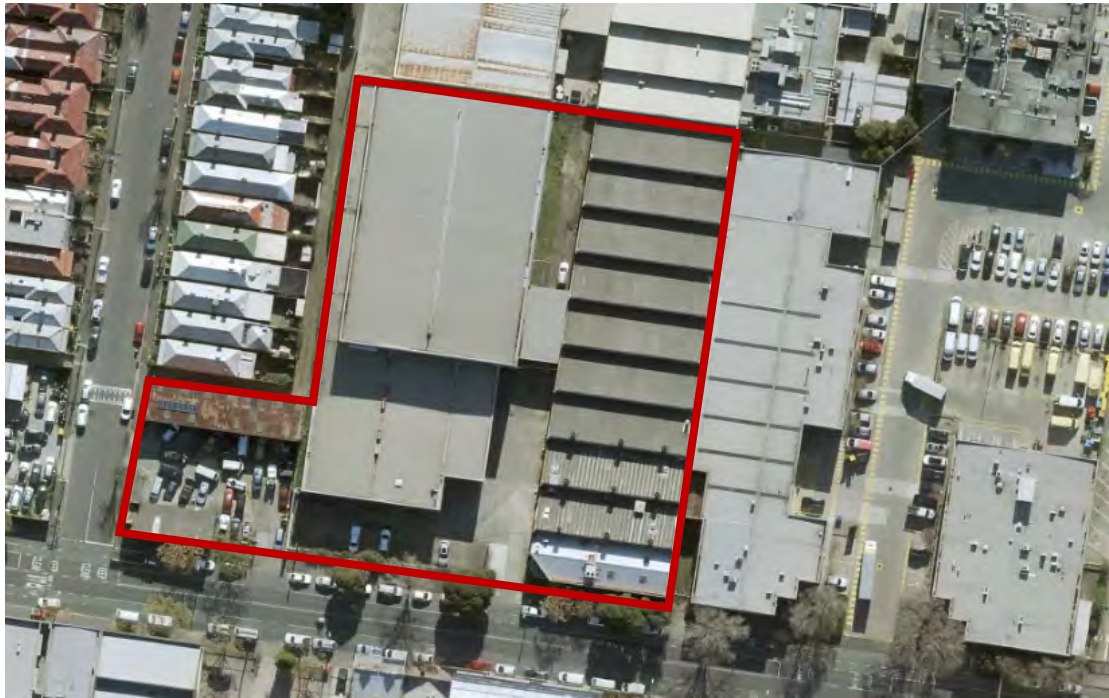
Figure 2 - MetroMap Aerial Photo of site. Captured on 20 July 2022
