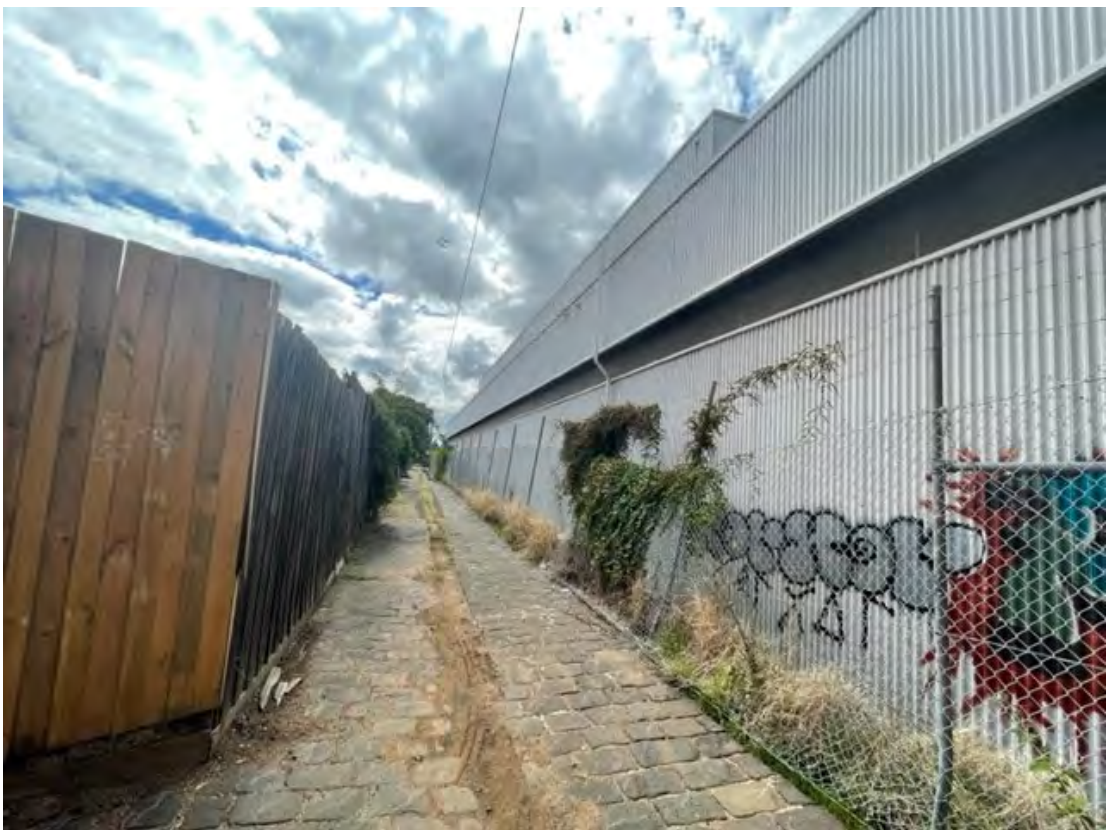
Figure 5 - View north along Council Laneway 167 with subject site on right. Captured on 28 March 2022
