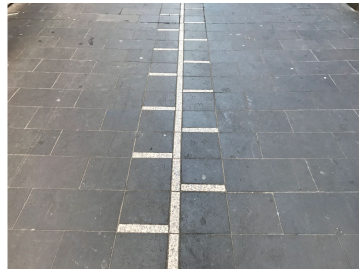
Example of customised bluestone paving with granite inlay
