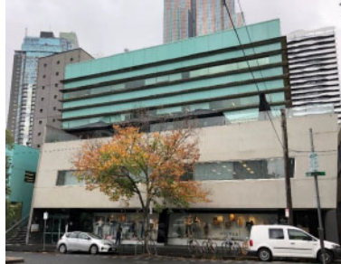
Building 94 (23-37 Cardigan Street, Carlton)
