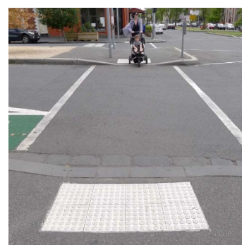
Examples of kerb access ramps
