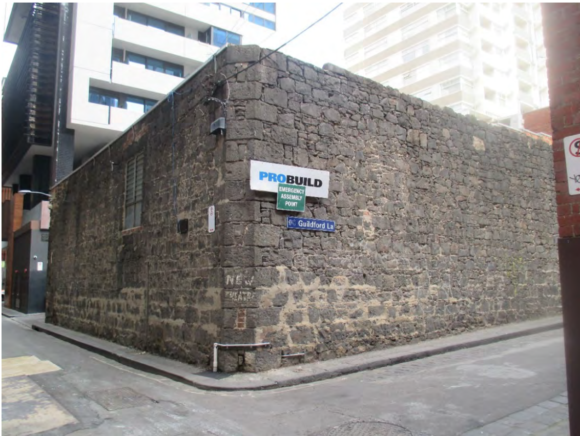
Figure 38 Former Bucks Head Hotel stables, 15 Sutherland Street
