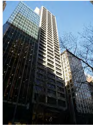
Former Commonwealth Banking Corporation Building, 359-373 Collins Street (Bates Smart & McCutcheon, c1972-75)
