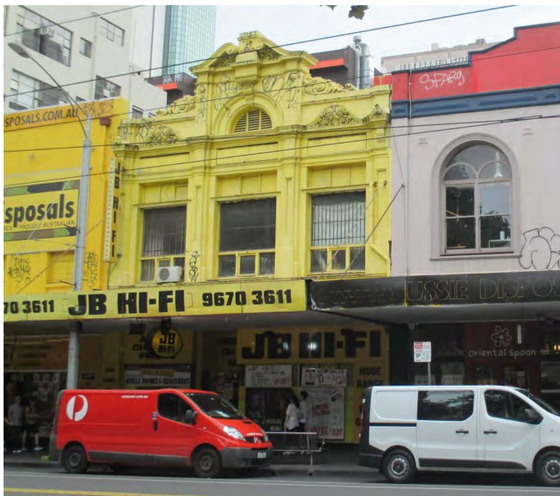
Figure 28 The former John Cooper and Co premises at 287 Elizabeth Street
