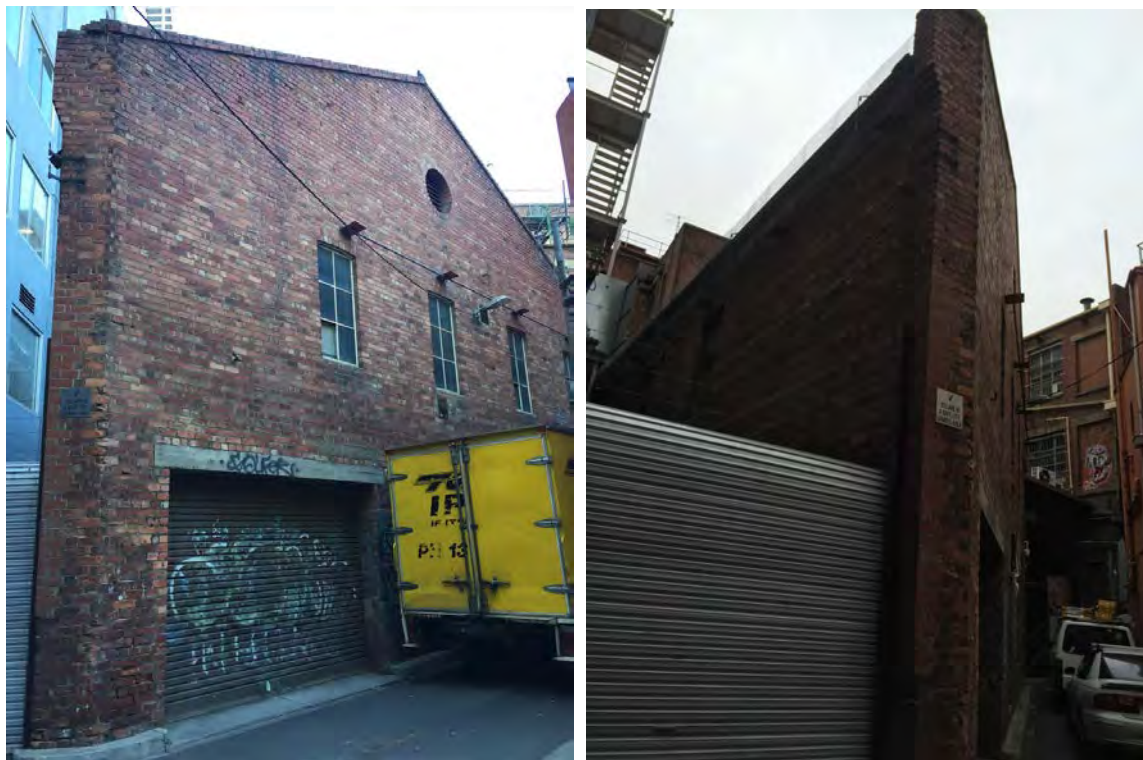
Figure 1 Subject building, east elevation (at left) and side (south) elevation (at right)
