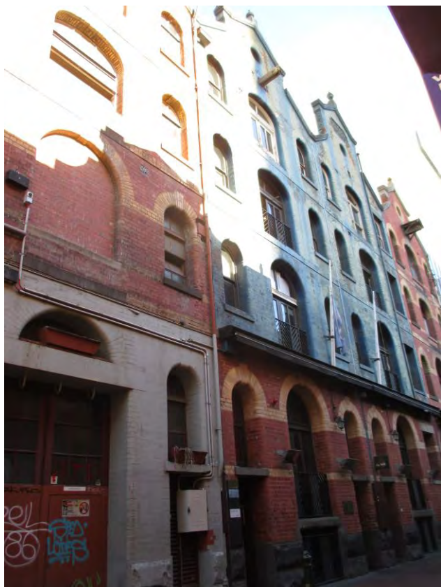
Figure 1 Subject warehouse row (four buildings)
