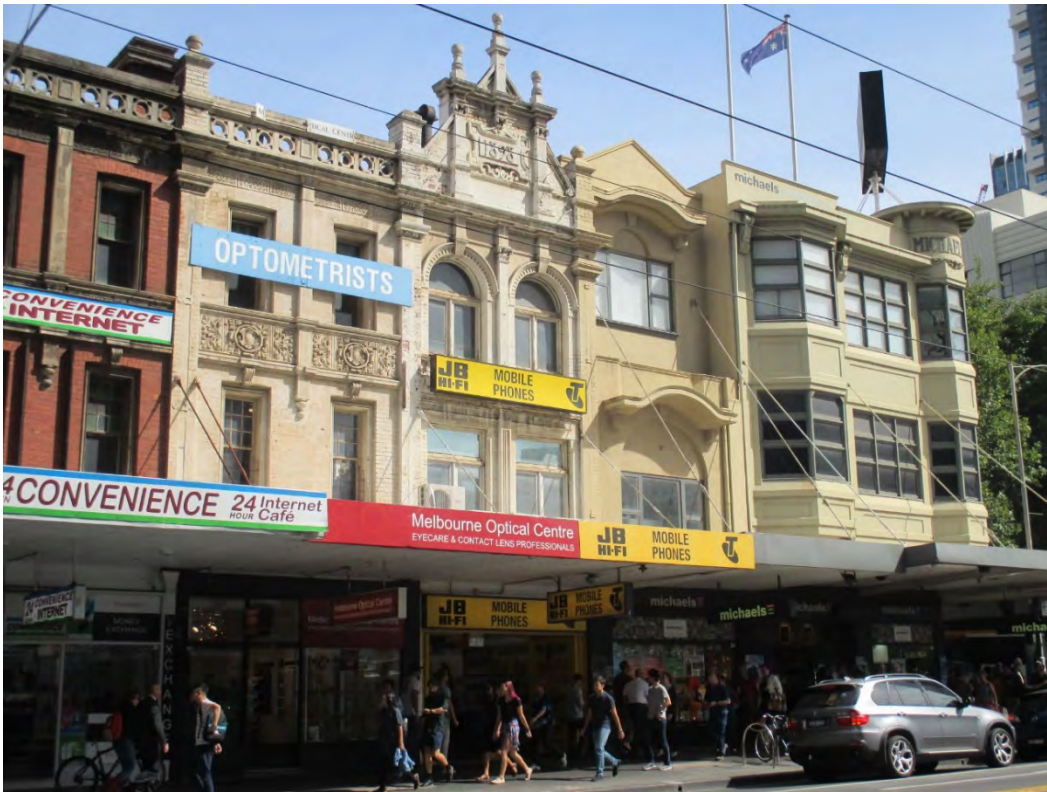
Figure 14 Development at nos. 259-269 on the west side of Elizabeth Street, northern section of precinct; Michaels Building at the corner of Lonsdale Street is visible at right
