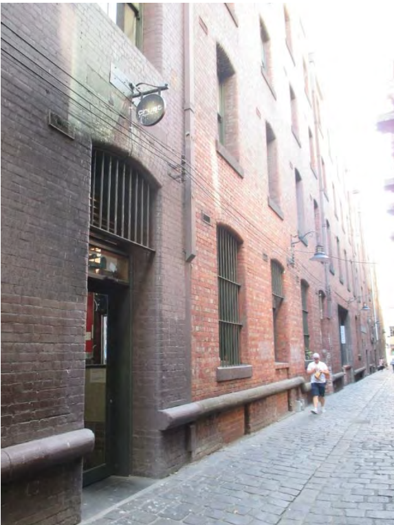
Figure 2 West elevation of subject building (to Niagara Lane)
