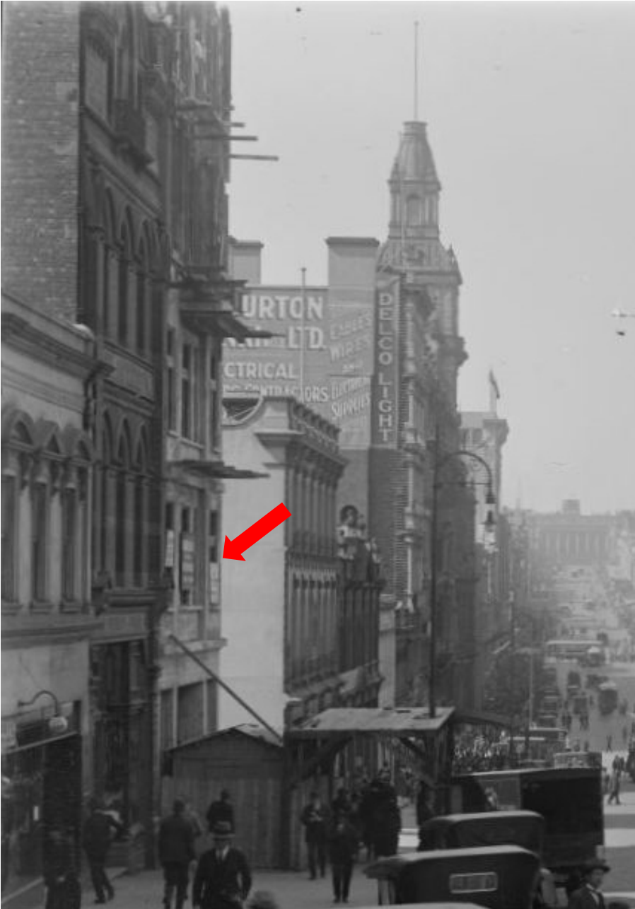
Figure 8 Detail, Bourke Street, looking to Parliament House, Rose stereograph co, c1920-1954 [sic] shows 414-416 Bourke Street under construction (indicated) Source: State Library of Victoria
