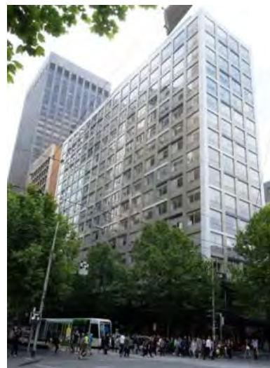
MLA Building, 308-336 Collins Street (Stephenson & Turner, 1963)
