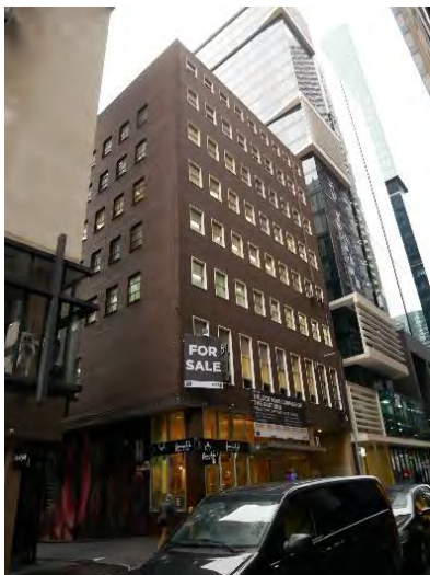
Former Methodist Church Centre, 130-134 Little Collins Street (Bates Smart & McCutcheon, 1966-67)
