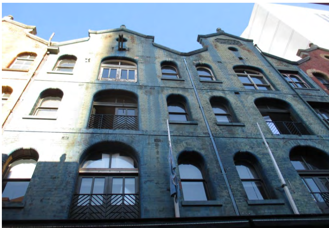
Figure 2 View of upper level facades
