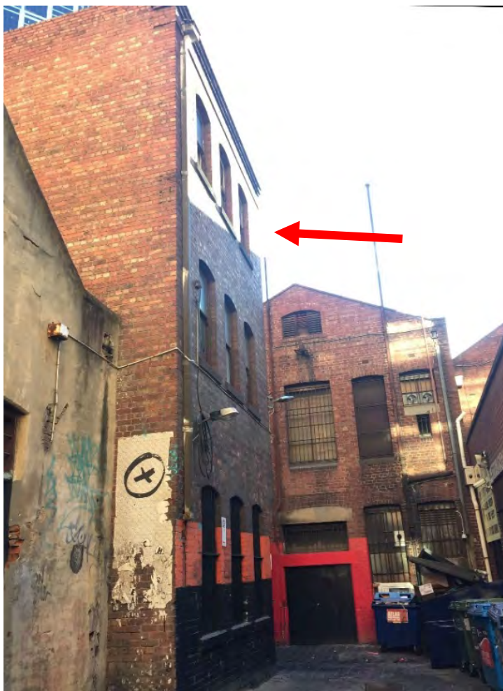
Figure 25 South elevation of the subject three-storey brick building at left (indicated); the rear of the building at 291-3 Elizabeth Street is visible in the distance
