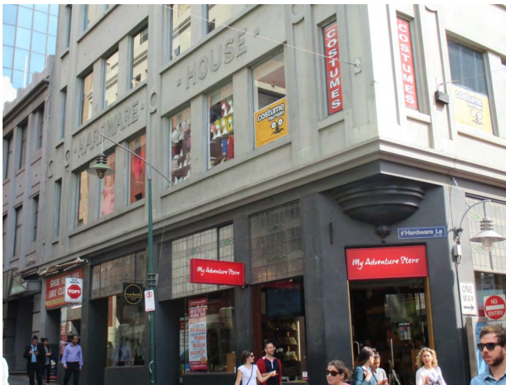
Figure 45 Ground floor façade, Hardware House
