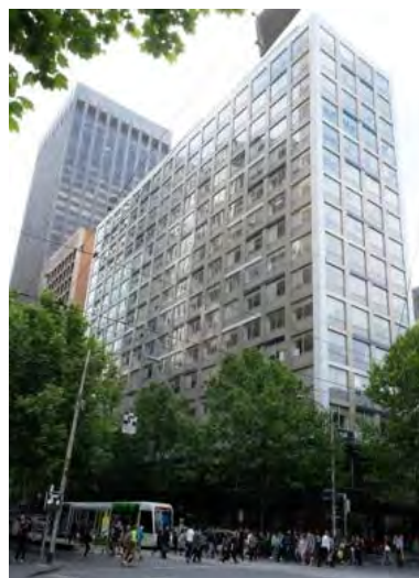
MLA Building, 308-336 Collins Street (Stephenson & Turner, 1963)
