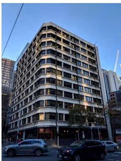
Office Building, 589-603 Bourke Street (Peddle Thorp de Preu, 1973-75)
