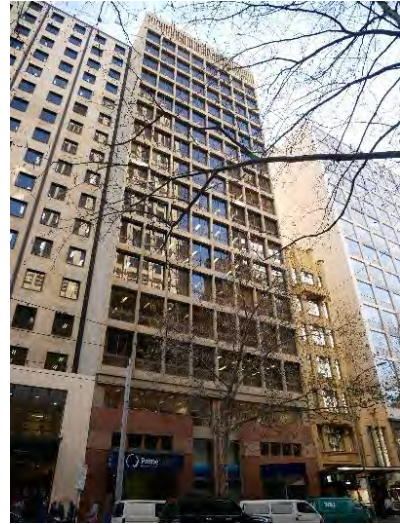
Former AMP Building, 344-350 Collins Street (Godfrey & Spowers, Hughes Mewton and Lobb, 1966-68)
