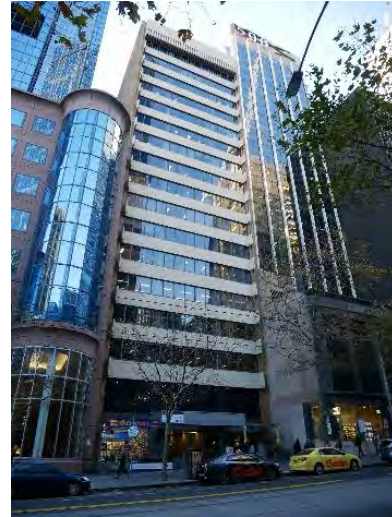
Office Building, 516-520 Collins Street (architect unknown, c1974)
