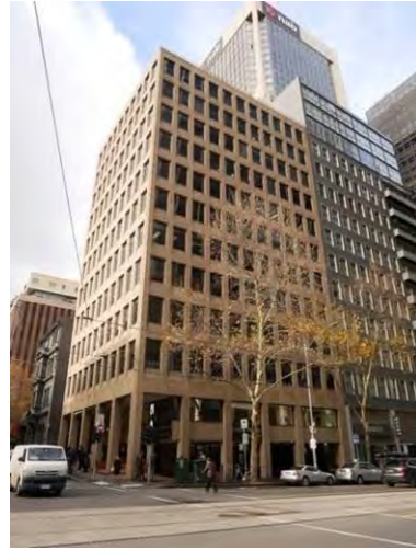
Office Building, 178-188 William Street (McIntyre McIntyre & Partners, 1972-72)
