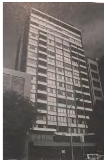
Figure 2. Park Tower soon after completion (Source: Edquist 2002: 19)
