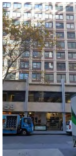
Cowan House, 457-469 Little Collins Street (E & G Kolve, 1969)
