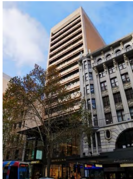
Former Commercial Banking Company of Sydney Building, 251-257 Collins Street, (Bates Smart & McCutcheon, 1974-73) included in HO502 The Block Precinct (fronting Collins Street) & HO506 (fronting Flinders Lane) (Non-contributory).
