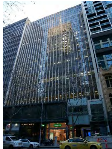
Former Australia-Netherlands House, 468-478 Collins Street (Meldrum & Partners with Peddle Thorp Walker, 1968-70)
