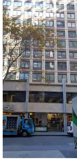
Cowan House, 457-469 Little Collins Street (E & G Kolle, 1969)
