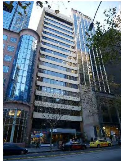
Office Building, 516-520 Collins Street (architect unknown, c1974)
