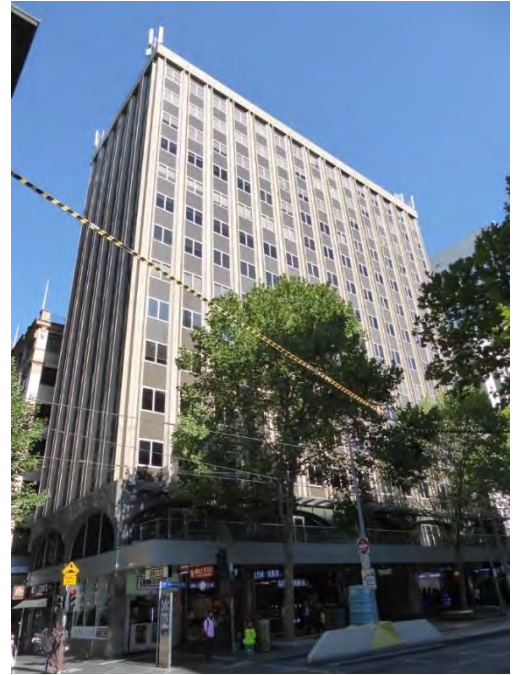
Former State Savings Bank of Victoria, 45-63 Swanston Street, (Buchan Laird & Buchan, 1974) included in HO505 Flinders Gate Precinct (Non-contributory).
