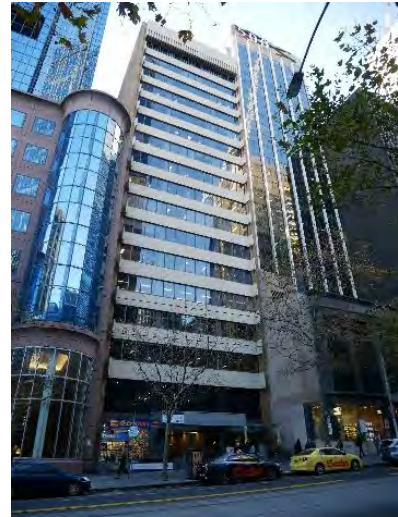
Office Building, 516-520 Collins Street (architect unknown, c1974)
