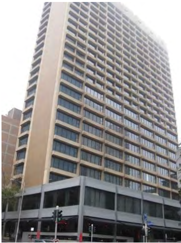
Former Bryson Centre, 174-192 Exhibition Street (Perrot Lyon Timlock & Kesa, 1970-72)
