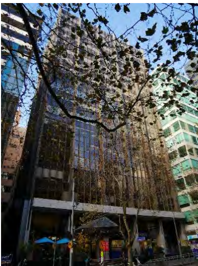
Former Dalgety House, 457-471 Bourke Street (Peddle Thorp & Walker, 1966-68)
