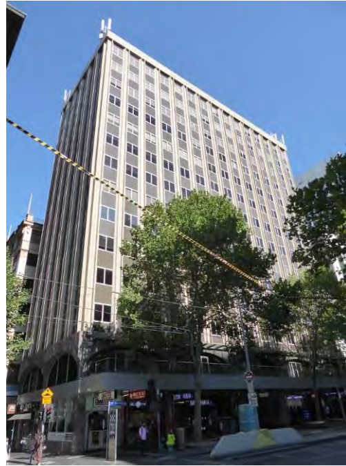
Former State Savings Bank of Victoria, 45-63 Swanston Street, (Buchan Laird & Buchan, 1974) included in HO505 Flinders Gate Precinct (Non-contributory).
