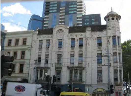
Figure 2. 2-8 Spencer Street, built in 1913.
