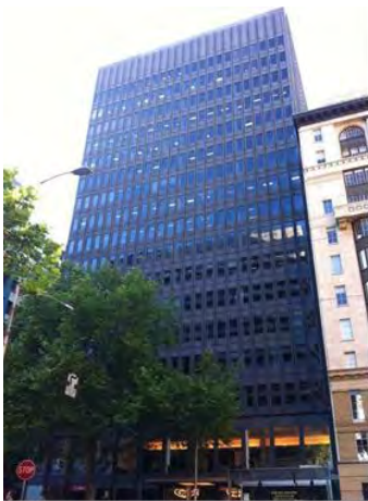
Royal Insurance Group Building, 430-442 Collins Street (Yunken Freeman, 1966)
