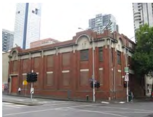
Figure 2. Substation at 651-669 Lonsdale Street constructed 1915.
