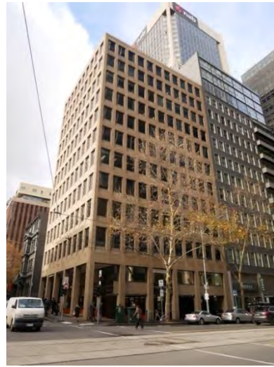
Office Building, 178-188 William Street (McIntyre McIntyre & Partners, 1972-73)
