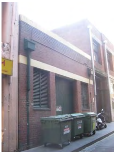
Figure 5. Substation at 28 Crossley Street, unknown build date.
