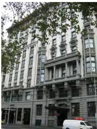
Figure 7. 318-324 Flinders Street, built in 1913.
