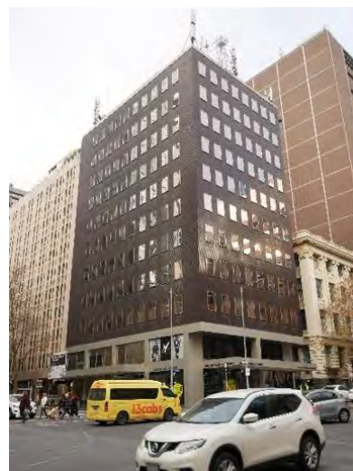
Former State Saving Bank of Victoria, 233-243 Queen Street (Godfrey & Spowers, Hughes Mewton and Lobb, 1967-68)
