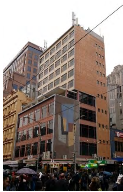
Former Hosie's Hotel, 1-5 Elizabeth Street & 288-290 Flinders Street (Mussen McKay & Potter, 1954-55), included in HO505 Flinders Gate Precinct as a Significant place.
