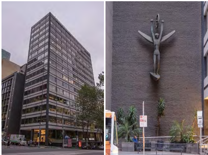
158-164 Queen Street and 'Transformation', built in 1964. (Source: Context 2019)
