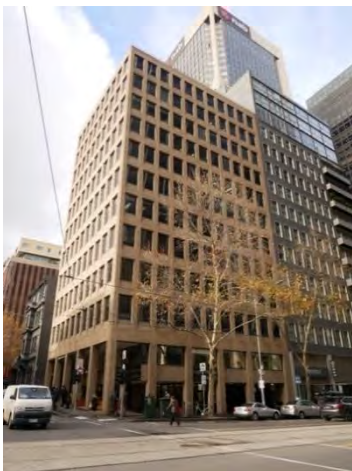
Office Building, 178-188 William Street (McIntyre McIntyre & Partners, 1972-73)
