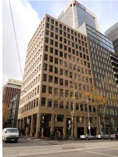
Office Building, 178-188 William Street (McIntyre McIntyre & Partners, 1972-73)
