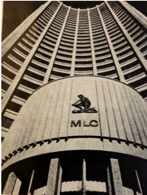
Figure 4. Photo of the building published in the May/June edition of Architecture in Australia (AIA, May/June 1973:8).
