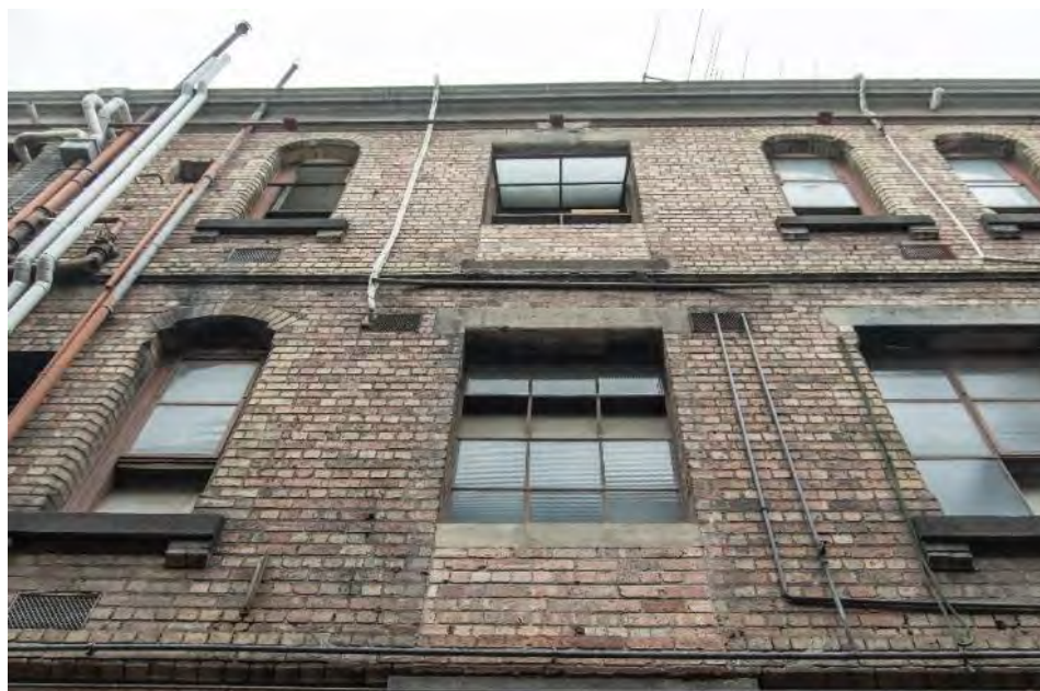
Figure 8. Side elevation of 365-367 Little Bourke Street fronting Warburton Lane. Later rectangular openings with concrete lintels and sills, and the original window openings with cement sills with brackets and splayed edges on the either side of the later openings. (Source: Context, January 2020)
