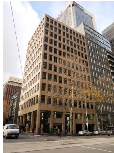
Office Building, 178-188 William Street (McIntyre McIntyre & Partners, 1972-73)
