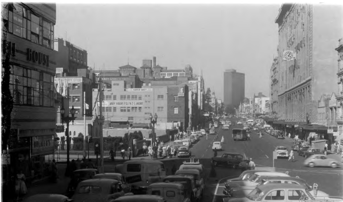
Figure 5. Lonsdale Street showing ICI building, Melbourne, Vic. Rose Stereograph Co, 1955 (State Library of Victoria)
