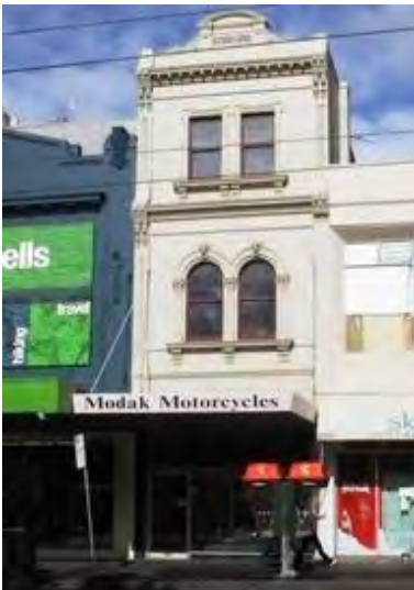
Figure 22. 299 Elizabeth Street, constructed 1885. (Source: CoMMaps)
