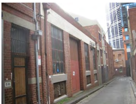
Figure 6. 12-14 Guildford Lane, substation constructed c1920.
