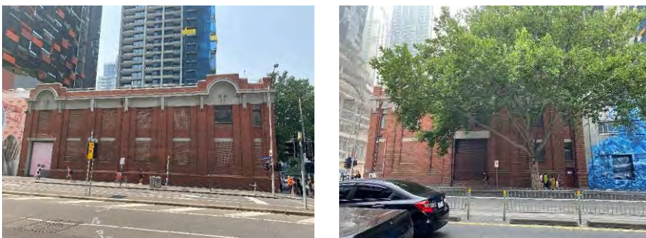
Figure 10. Elevations of the CitiPower 'Substation J' at Lonsdale Street (left) and Spencer Street (right). (Source: Context, January 2020)
