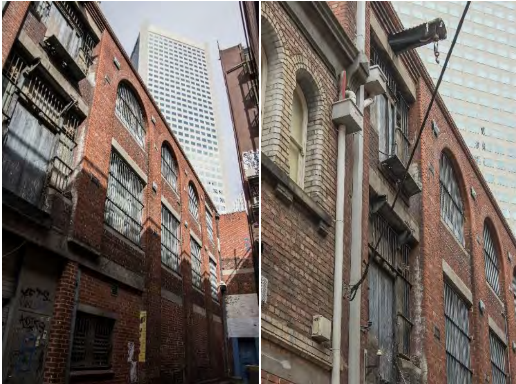
Figure 9. The 1912 warehouse fronting Warburton Lane, at the rear of 384-386 Bourke Street (left). Note the upper-level detailing of the Warburton Lane warehouse, including the corbel heads detailing above each end bay, timber loading doors and a hoist (right). (Source: Context, March 2019)
