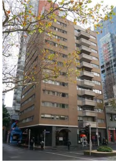
Exhibition Towers, 287-293 Exhibition Street (Kenneth McDonald & Associates, 1969-71)
