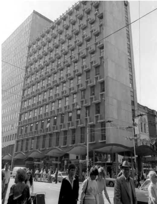
Figure 10. Royal Mail House in the early 1980s (City of Melbourne Libraries online Heritage Collection, Reference no. Butler16291; photo dated 1982-1985).
