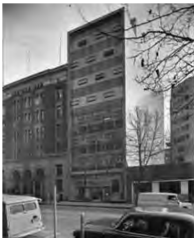
Figure 1. 468-470 Bourke Street in 1959. (Source: Sievers 1959, SLV H2003.100/219 copyright )
