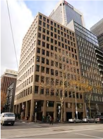
Office Building, 178-188 William Street (McIntyre McIntyre & Partners, 1972-73)
