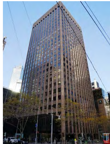
AMP Tower and St James Building Complex, 527-555 Bourke Street (Skidmore Owings & Merrill in association with Bates Smart & McCutcheon, 1965-69)
