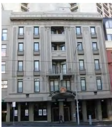
Figure 4. 66-70 Spencer Street, built in 1926-28.
