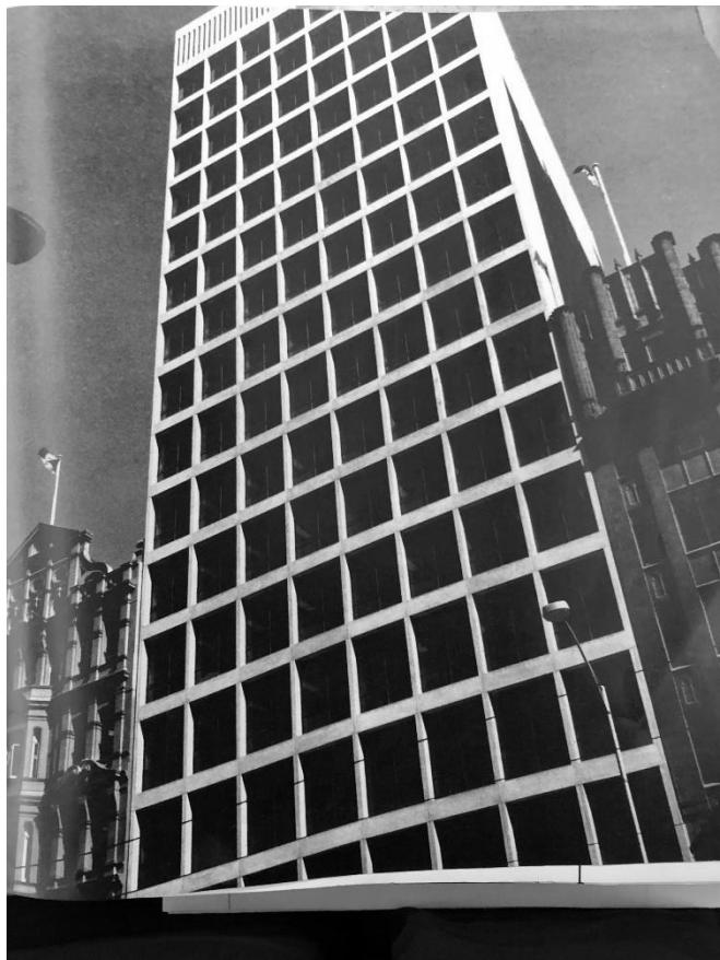
Figure 5. Photo of the building published in the Sep/Oct 1969 edition of Architect (Sep-Oct 1969:25).
