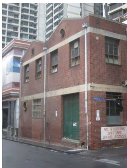
Figure 3. Substation at 620-648 Little Bourke Street constructed 1910-1925.
