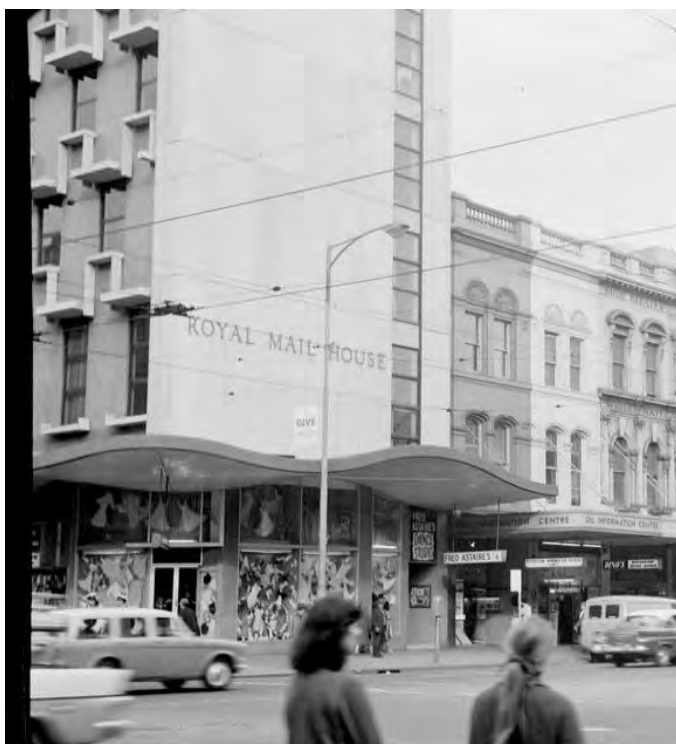
Figure 5. Detail of a 1966 photo showing the western end of the completed building (SLV, K. J. Halla, photographer, Image H36133/209).
