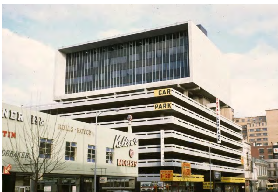
Figure 6. Total House at the corner of Russell and Little Bourke Street, 1966 (State Library of Victoria H91.244/5423)
