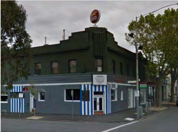
Figure 5. Royal Mail Hotel, 519 Spencer Street West Melbourne constructed 1938. (Source: Google Maps)
