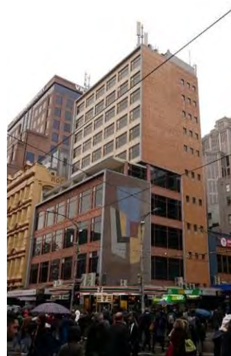
Former Hosie's Hotel, 1-5 Elizabeth Street & 288-290 Flinders Street (Mussen McKay & Potter, 1954-55), included in HO505 Flinders Gate Precinct as a Significant place.
