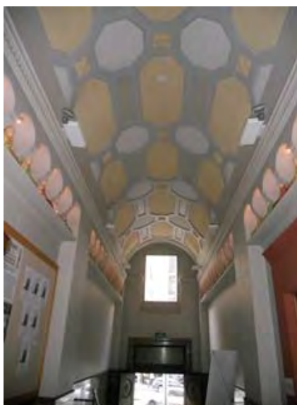
Figure 11. Entry with decorative plaster vaulted ceiling. (Source: Melbourne Heritage Action)
