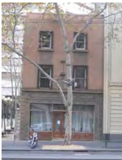
Figure 2. 74 Collins Street, former residence and surgery constructed 1855.
