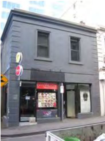
Figure 9. 474 Little Lonsdale Street constructed 1870s. (Source: Context 2017)
