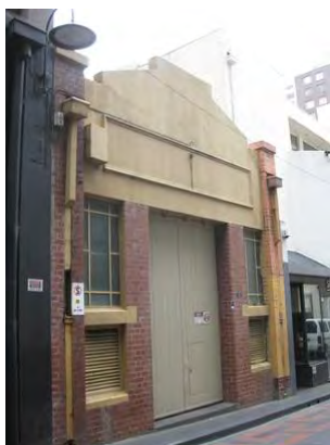
Figure 7. 21 Market Lane, unknown built date
