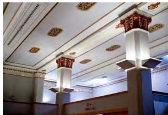
Figure 10. Ground level chamber ceiling and column detail ceiling. (Source: Melbourne Heritage Action)
