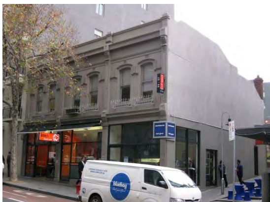
Figure 6. 53-57 Lonsdale Street, built c1880-81.
