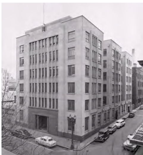
Figure 1. Exterior, Melbourne and Metropolitan Tramways Board, 616-622 Little Collins Street, Melbourne, c.1952, by Lyle Fowler (Source:SLV)
