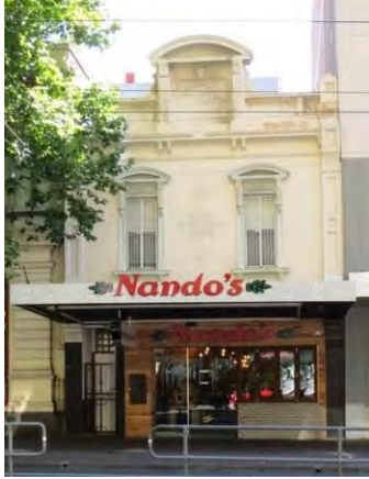
Figure 7. 380 Elizabeth Street, built c1850s, façade 1888
