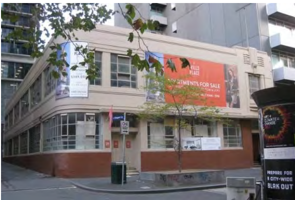
Figure 7. 17-23 Wills Street, built c1930s.
