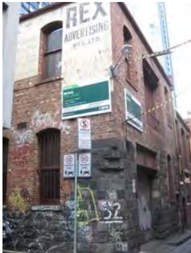
Figure 7. 32-34 Guildford Lane constructed 1908 & 1920.
