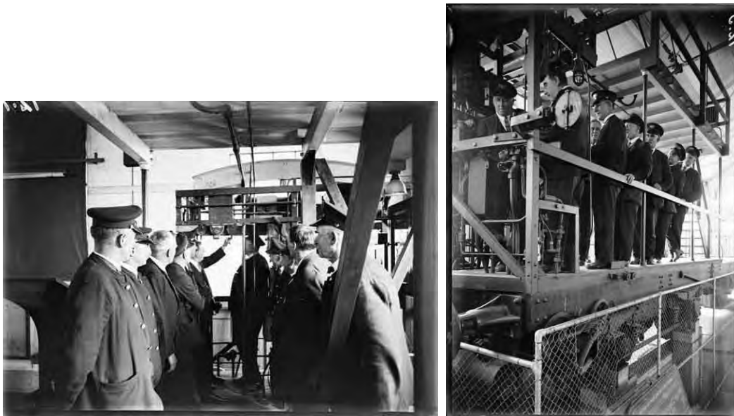
Figures 15 & 16. Photographs of the interior of the Princes Bridge Lecture Room, undated (Source: PROV, VPRS 12903/P1 item 012)
