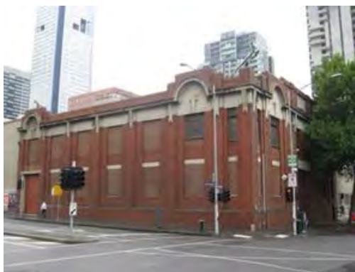
Figure 2. Substation at 651-669 Lonsdale Street constructed 1915.
