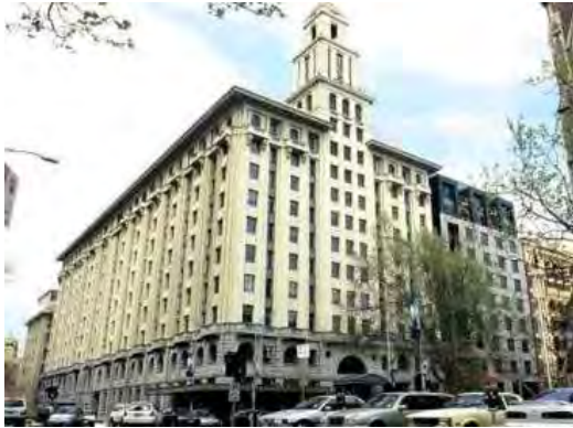
Figure 6. 141-165 Collins Street constructed 1929. (Source: VHD)
