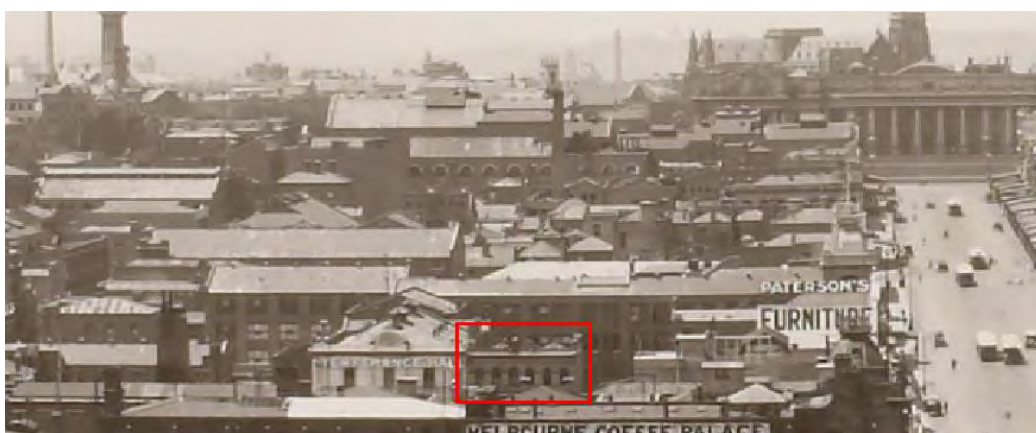
Figure 1. A 1920s bird-eye view over Bourke Street shows the subject building at its full extent. (Source: Row 1932, SLV)
