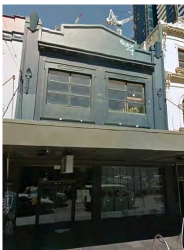
Figure 4. 295-297 Elizabeth Street, built in the early 1930s. (Source: Google 2019)
