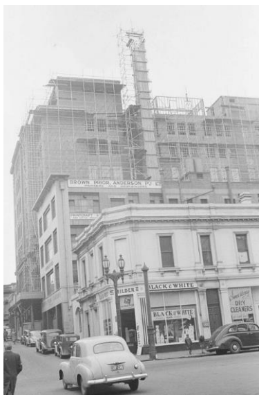
Figure 3. The subject building is shown in the middle ground in 1955 with the multi-storey City West Telephone Exchange in Little Bourke Street under construction behind. A sign for the original occupants Brown, Prior, Anderson P/L. is clearly visible on the side of the building. (Source: Strizic 1955, SLV copyright)
