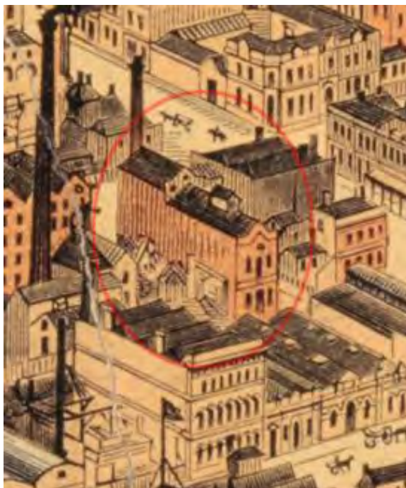
Figure 1. Russell & Gillespie's flour mill chimney and back building facing Francis Street shown in a section of Melbourne, 1882, by A C Cooke (Source: SLV).
