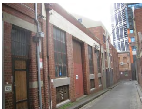
Figure 6., Substation at 12-14 Guildford Lane constructed c1920.
