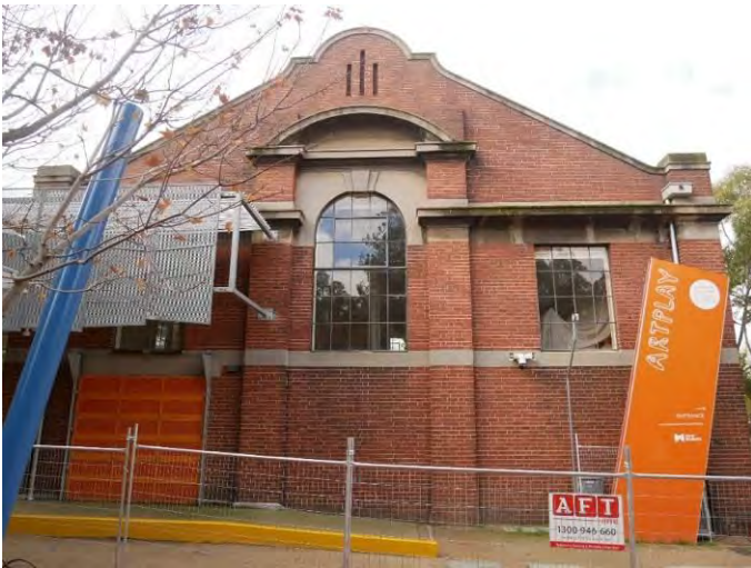
Figure 24. West elevation of the Former Princes Bridge Lecture Room. (Source: GJM Heritage May 2020)
