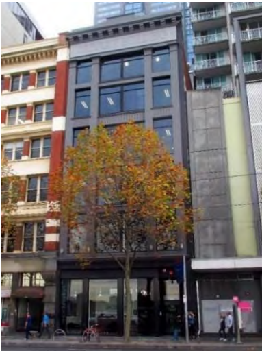
Figure 5. 96-98 Flinders Street, built in 1915. (Source: Context 2017).
