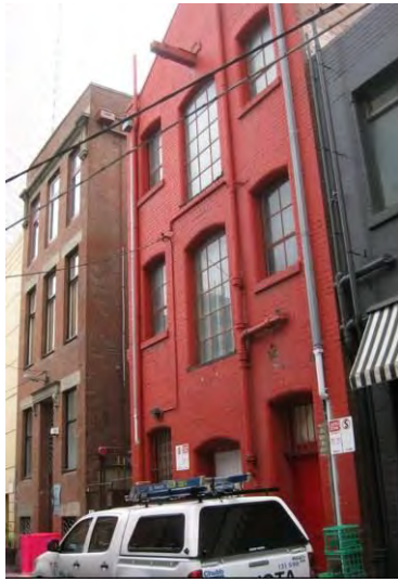
Figure 6. 17 Somerset Place constructed c1907-08.
