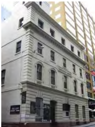
Figure 3. 538-542 Little Collins Street constructed 1878-79.
