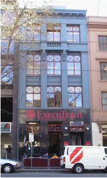
Figure 4. 482-484 Bourke Street, built in 1926. (Source: iHeritage)
