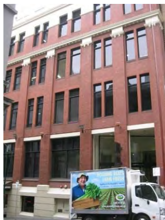
Figure 6. 401-405 Little Bourke Street, built in 1911 and remodelled in 1933.
