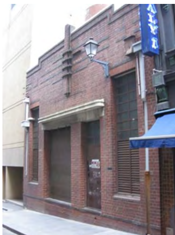
Figure 8. 23-25 George Parade constructed 1938. (Source: Context 2017)
