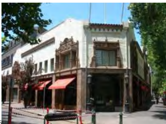
Figure 10. 375-385 St Kilda Road constructed 1926-29. (Source: HERMES)
