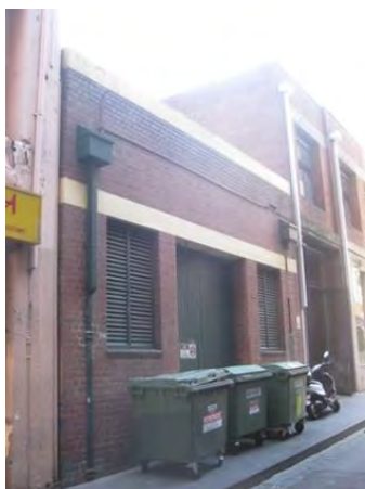
Figure 5. Substation at 28 Crossley Street, unknown built date.
