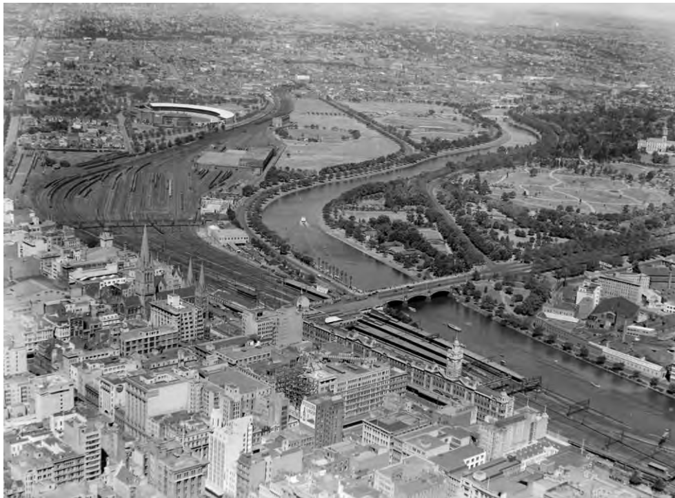
Figure 2. Aerial view from the north-west, showing the extent of the Jolimont railway yards, Victorian Railways, c 1945-c1954 (Source: SLV).
