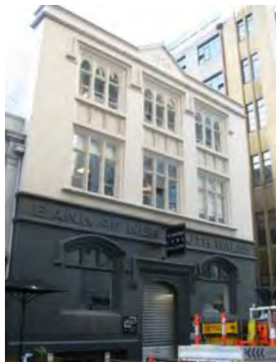
Figure 8. 137-139 Flinders Lane constructed 1924. (Source: Context 2018)
