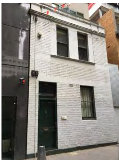
Figure 8. 20 Ridgway Place constructed 1898. (Source: Context 2017)
