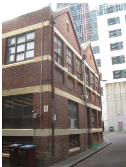
Figure 4. 1-3 Evans Lane constructed 1913.
