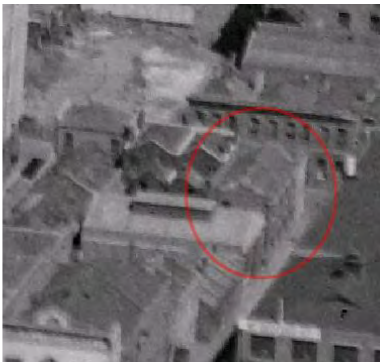
Figure 1. The boundary between the original 1870s rendered wall and newly added face brick part is clearly shown, from Aerial View of Melbourne, c.1945, by Victorian Railways (Source: SLV).
