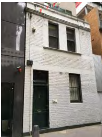
Figure 3. 20 Ridgway Place constructed 1896. (Source: Context 2017)
