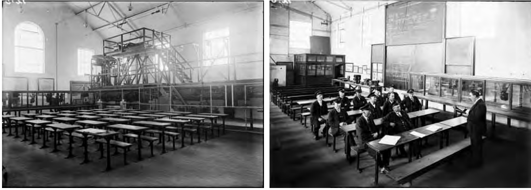
Figures 13 & 14. Photographs of the interior of the Princes Bridge Lecture Room, undated (Source: PROV, VPRS 12903/P1 item 012)
