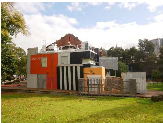
Figure 26. East elevation of the Former Princes Bridge Lecture Room, showing later addition. (Source: GJM Heritage May 2020)
