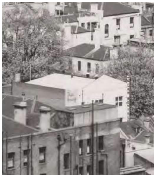
Figure 3. A view of 39-41 Little Collins Street with a sign 'Car Rentale' in Aerial views of Melbourne, looking south west and west. (Source: Commercial Photographic Company pre-1965, SLV)
