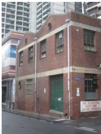
Figure 3. Substation at 620-648 Little Bourke Street constructed between 1910 and 1925.
