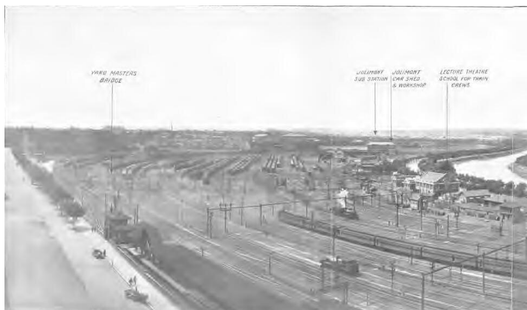
Figure 5. Part of Panoramic view of Flinders Street yard from C T Stephenson, The Electrification of the metropolitan railway system of Melbourne , 1919.
