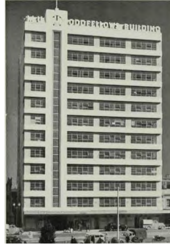
Figure 4. Photograph showing the MUOB in 1941. (Source: Building Vol 69, No 9, September 24 1941:10 copyright)
