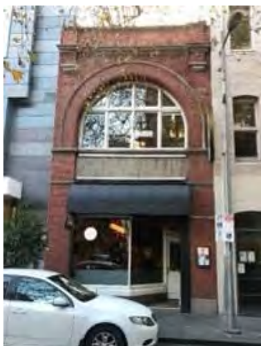
Figure 4. 37 Little Collins Street constructed. (Source: CoM, 2018)
