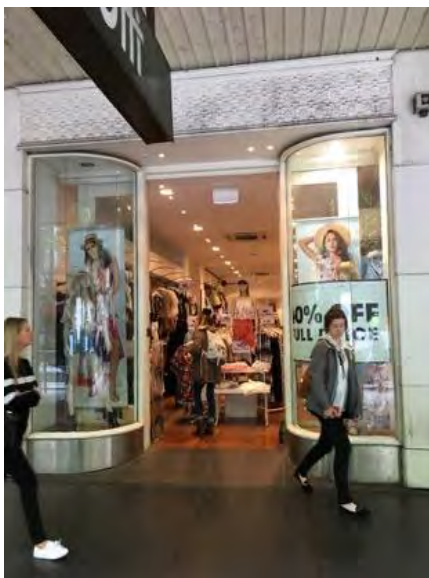
Figure 9. Shopfront at 161 Swanston Street retaining a recessed front entrance and curved glass with pressed metal panel above. (Source: Context 2017).
