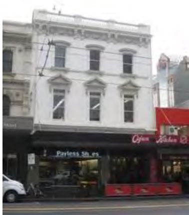
Figure 6. 136-140 Elizabeth Street, unknown built date.
