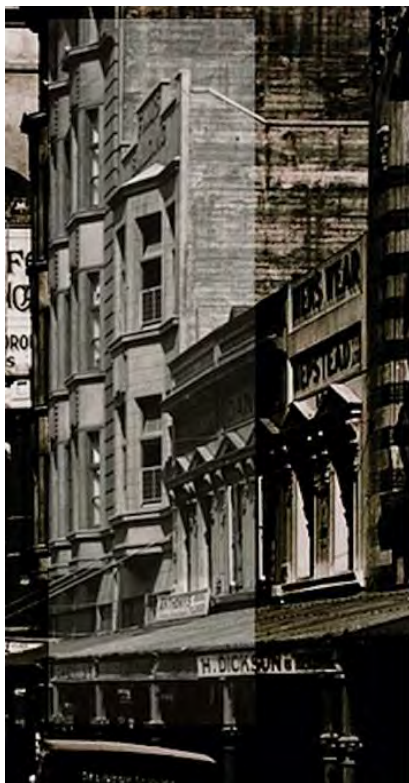
Figure 1. The three-storey Faul's Building at 139-141 Swanston Street is shown second from the left. Date unknown. (Source: Melbourne Heritage Action 2015)
