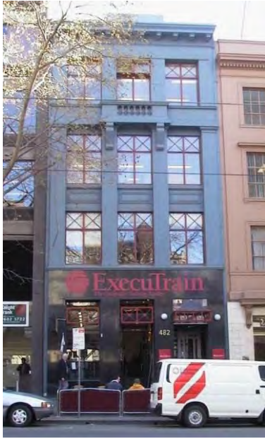
Figure 10. 482-484 Bourke Street, built in 1926. (Source: iHeritage)
