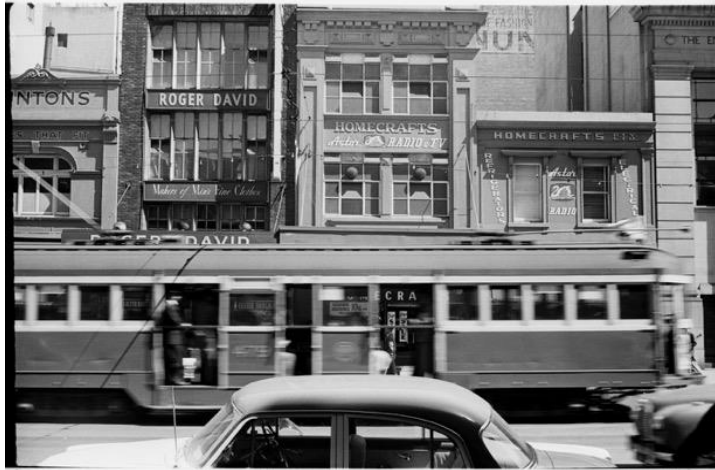
Figure 5. Showing the three-storey buildings at 207-209 Swanston Street occupied by Roger David and 211-213 Swanston Street occupied by Homecrafts c1950. (Source: Strizic c1950-c1980, SLV)
