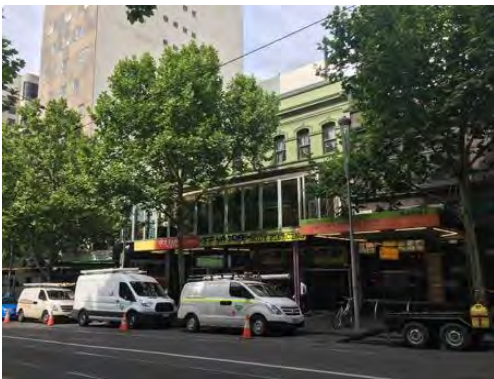
Figure 11. 243-249 Swanston Street with its added glazed balcony. (Source: Context 2017).
