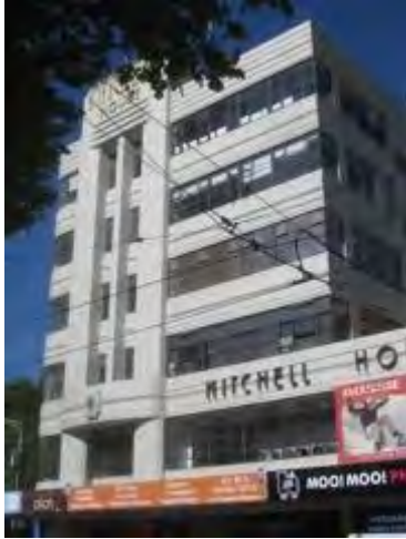
Figure 4. 352-362 Lonsdale Street constructed in 1937. (Source: CoMMAps)
