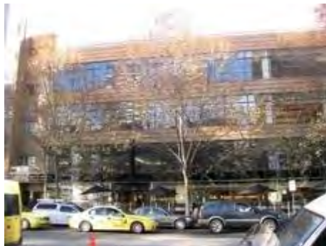
Figure 6. 546-566 Collins Street constructed 1935. (Source: CoMMAps)
