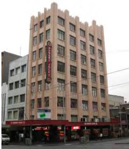
Figure 5. Norman's Corner Stores, 180-182 Bourke Street, built in 1935.
