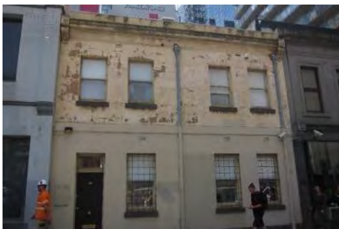
Figure 9. 120-122 Little Lonsdale Street, c1855 and in HO984. (Source: Context 2017)
