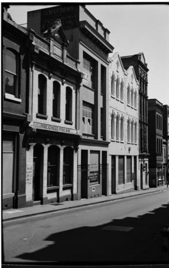
Figure 7. Little Lonsdale Street, 1968, showing numbers 281 (middle two-storey building) and 283-285 (to right of 281). (Source: Halla 1968, SLV)
