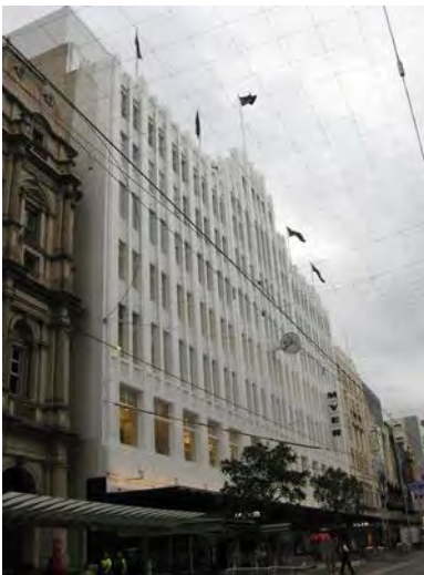
Figure 5. Myer Emporium, 314-316 Bourke Street, built in 1933.
