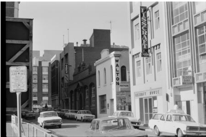
Figure 4. Flinders Lane between ACDC Lane (formerly Corporation Lane) and Exhibition Street showing Lisscraft House at 107-109, Walton Textiles at 103-105, and nos.87-95. (Source: Halla c1972, SLV H36133/484 copyright )
