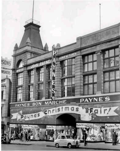
Figure 4. Now demolished Payne's buildings between 134-144 Bourke Street in 1955. (Source: Herald 2 December 2018)
