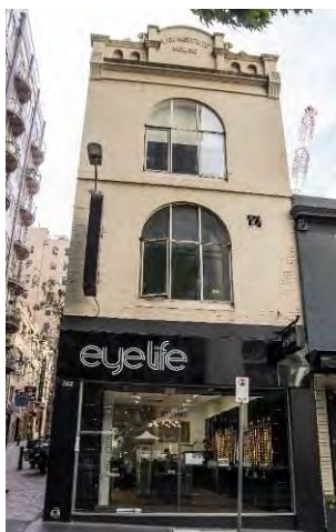
Figure 7. 382 Little Collins Street constructed 1905 and altered in 1924. (Source: Context 2019)
