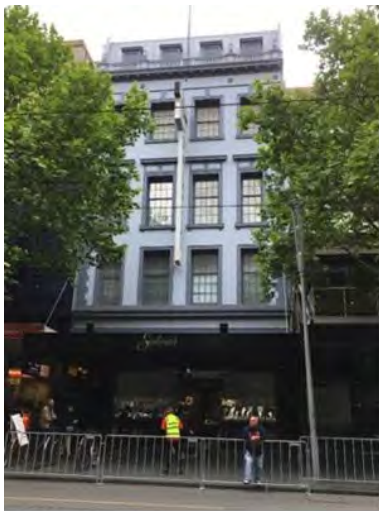
Figure 5. 152-156 Swanston Street, constructed 1888 and remodelled in 1938-39. (Source: Context 2017)
