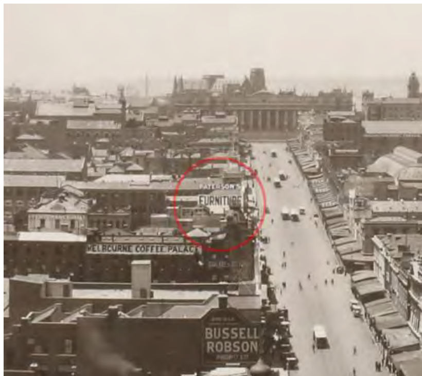
Figure 4. Patersons Furniture Warehouse in 1920 shown in a section of Melbourne 1920, showing Bourke Street, 1920, by Row. (Source: SLV)
