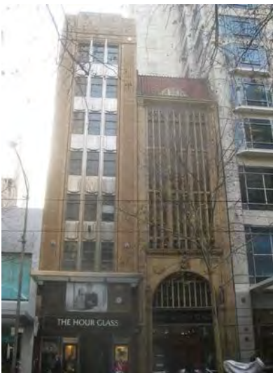
Figure 15. 250 Collins Street on right (built in 1930) and 252 Collins Street on left (built in 1935).
