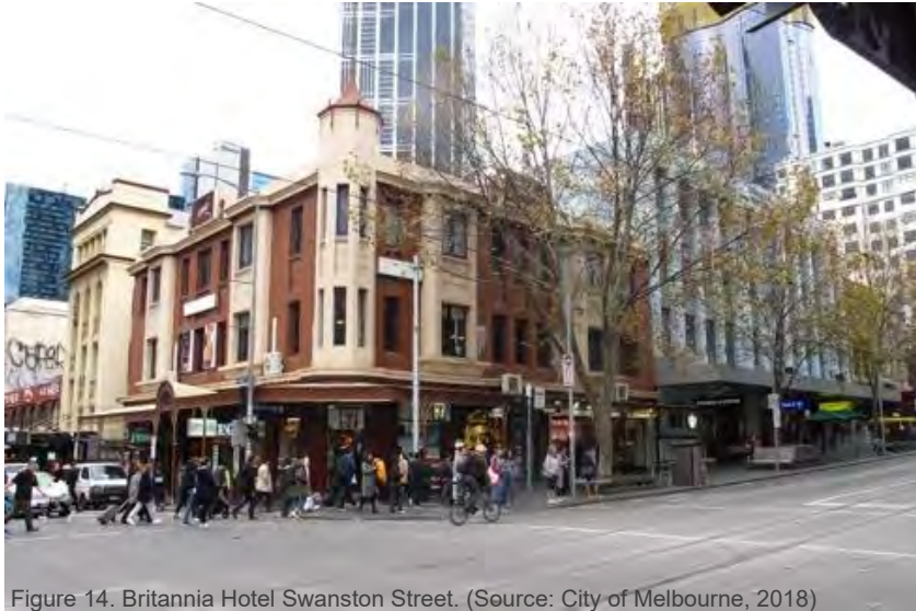
Figure 14. Britannia Hotel Swanston Street. (Source: City of Melbourne, 2018)
