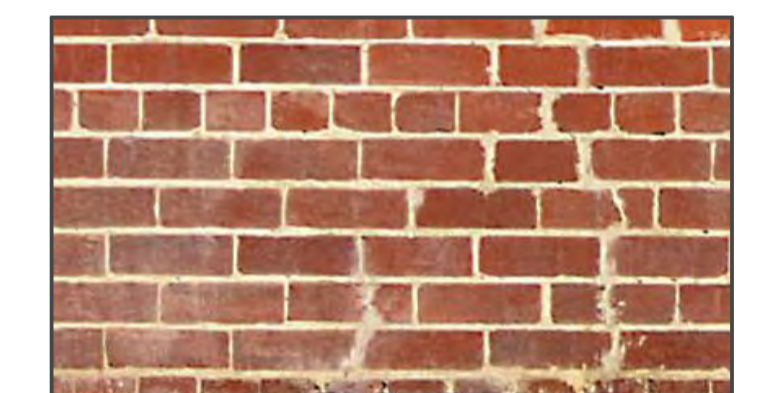
B1- RECYCLED RED BRICK, BRICKS FROM EXISTING FACADE TO BE CLEANED AND RE-USED
