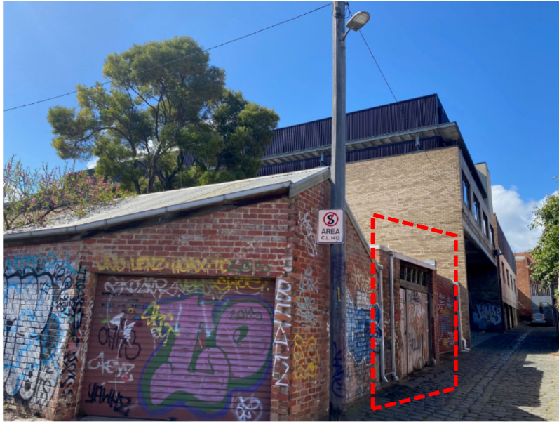
Figure 3 Rear of Site and adjoining properties
