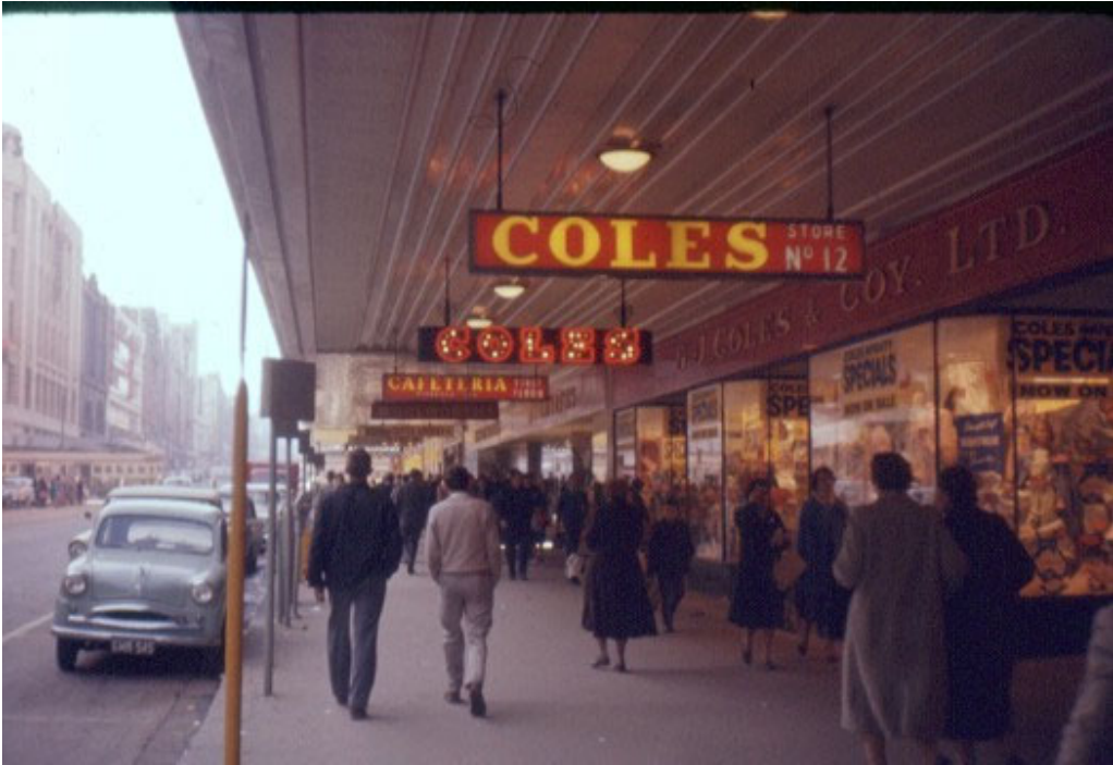
Photo Evidence of original shopfront layout to Bourke Street.
