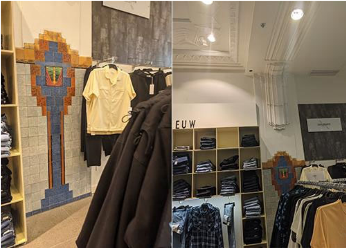
Surviving art deco details on the 1st Floor that should be enhanced.
