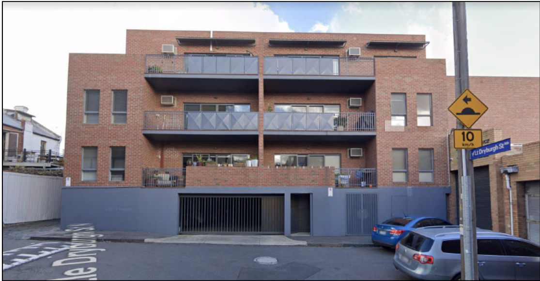
Figure 6 - Building West of the Site (700 Queensberry Street, North Melbourne)
