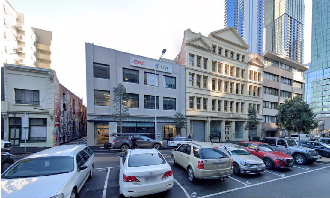
Figure 3 Image of Site from Franklin Street with Blender Lane on left (Source: Compass)
