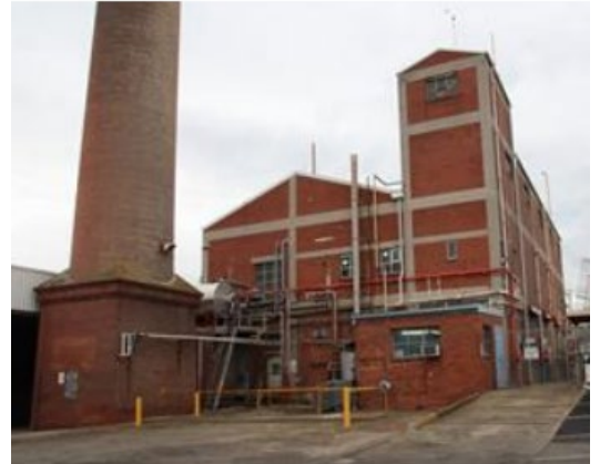
Chimney and boiler house of the Former Kraft Factory at 1 Vegemite Way (Source: P Mills 2020)
