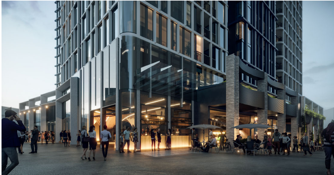
Podium view from the Stadium concourse. Source: Cox Architecture 2021
