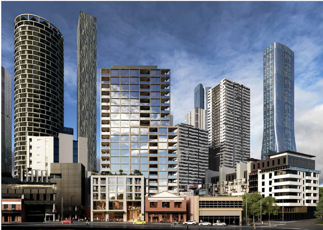
15. Perspective of proposal and surrounds from Queen Street: Urban Context Report - March 2021. BatesSmart Pty Ltd. *Note the scheme has since changed by reducing the height of the southern podium wall from 40 metres (shown in this image) to 22 metres.
