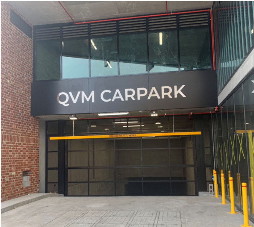
Figure 2: Practical completion of the 500 space Queen Victoria Market customer car park on Queen Street occurred mid March 2021. Following fit out, the car park is scheduled to be operational in July 2021.
