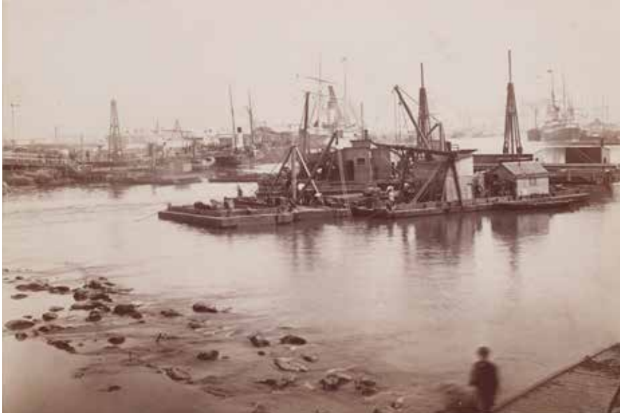
Image 6. This photograph shows the Yarra falls (the rocks in the foreground) being removed in 1883. The dredges can be seen hauling away large rocks. Source : Nettleton, C 1883, 'Dredge on Yarra', accessed on 21 April 2021: slv.vic.gov.au
