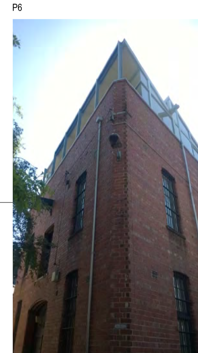
54a canning street off nicholls lane 3 storey modern alterations and additions to existing building with balcony
