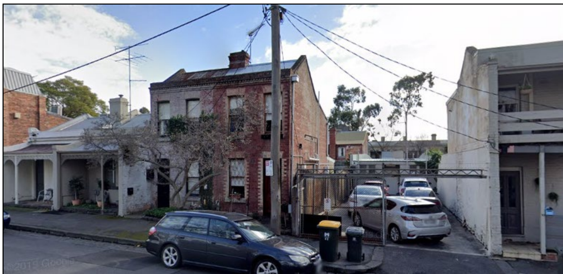
Figure 7 – Rear of 65 Elgin Street and 14 and 16 MacArthur Place North
