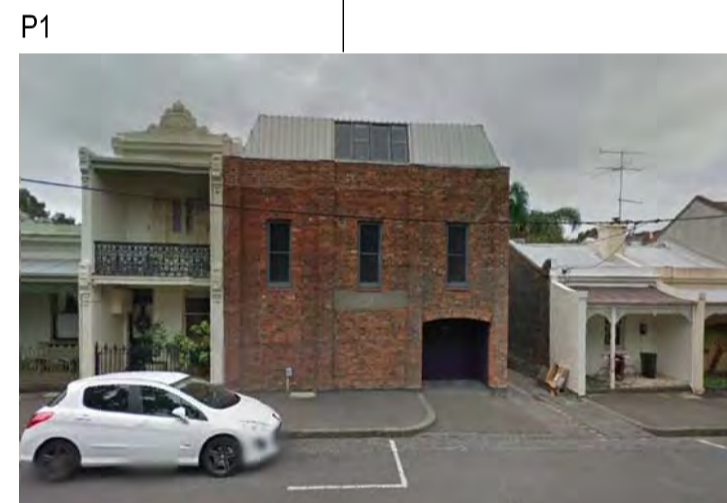
22 macarthur place north 3 storey modern addition to existing building
