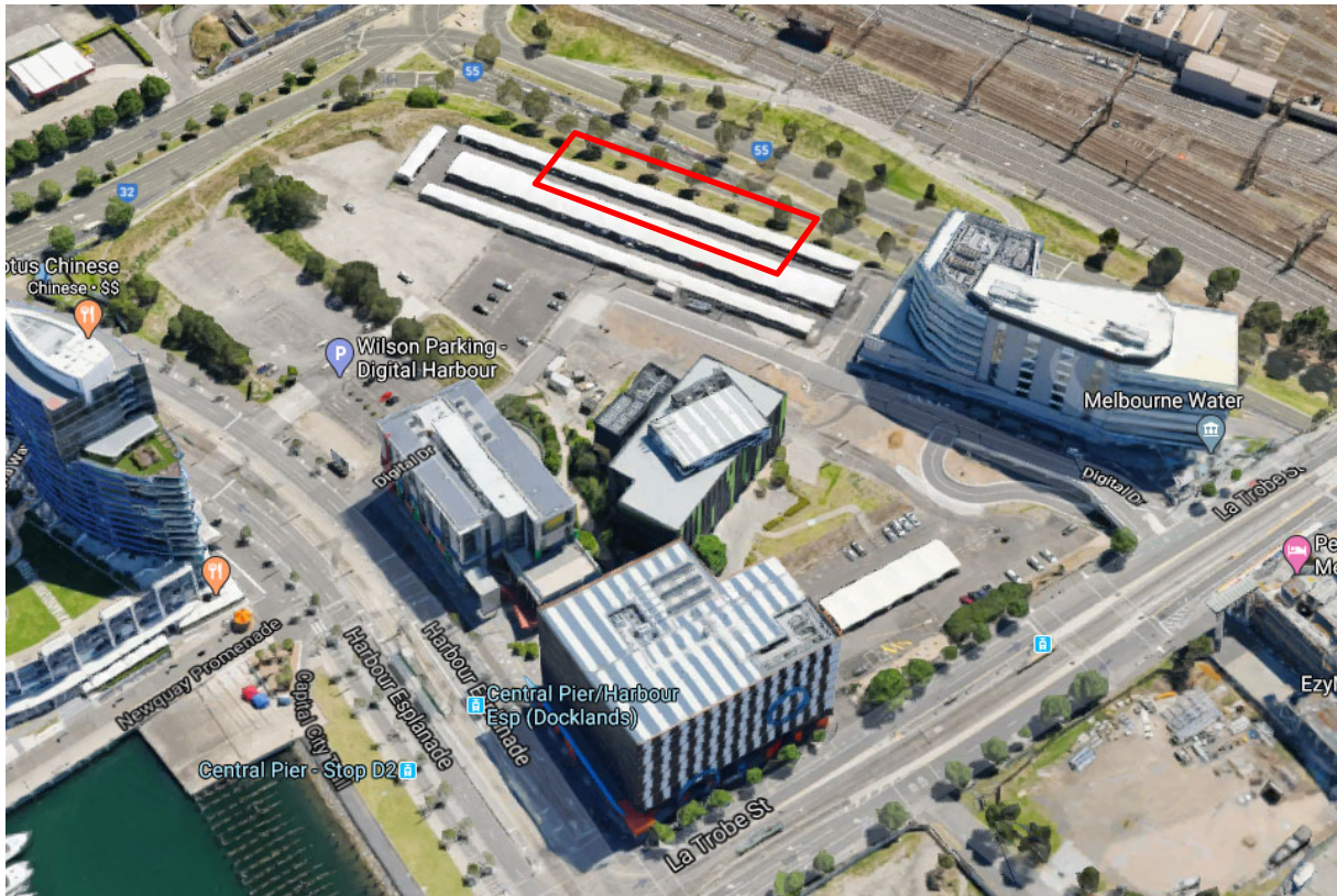
Figure 1: Aerial image of Digital Harbour precinct. Subject site highlighted in red (source: Google maps)
