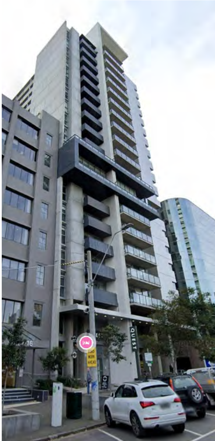
Figure 3: The adjoining building to the east (source: Google streetview)
