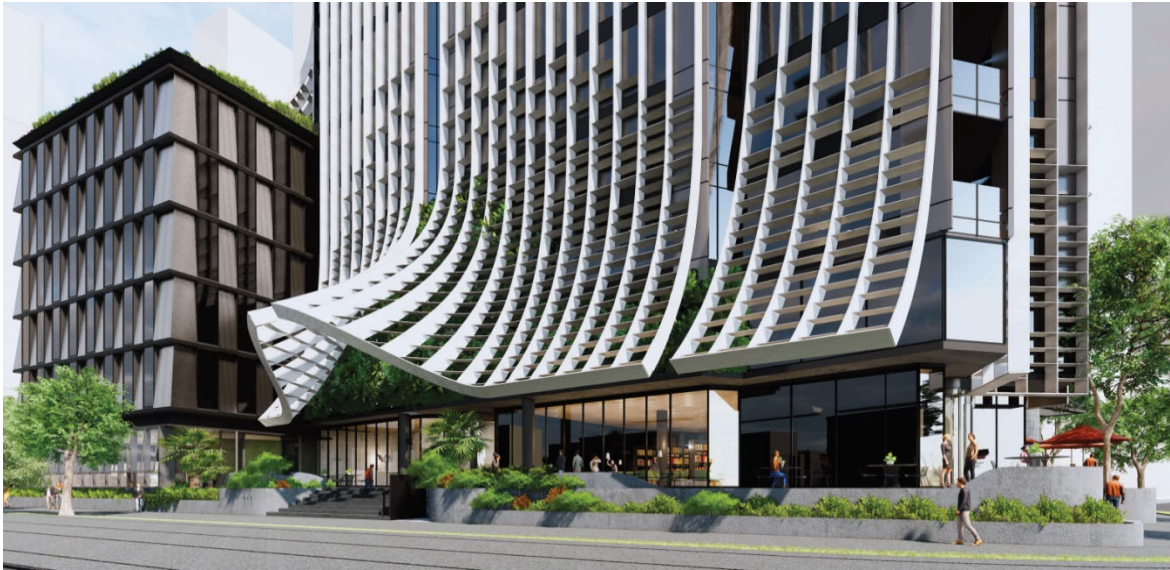
Figure 13 - Lorimer Street frontage showing access point to office and community space (source: application plans prepared by Rothe Lowman)
