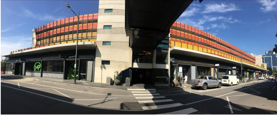
Figure 6 – West elevation of the existing building on the site, taken on 8 January 2020
