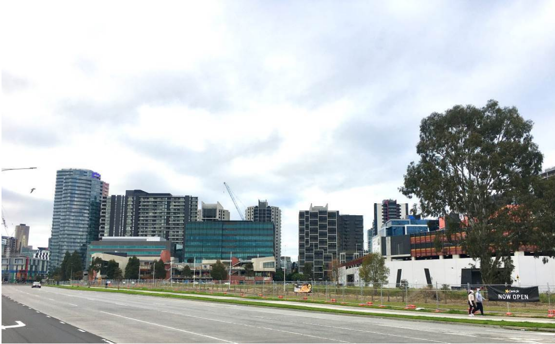
Figure 4 – View SE across the site from Footscray Road, taken on 17 August 2020
