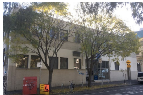
Recent photograph of the Bouverie Street elevation
