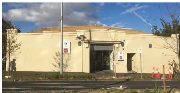
Recent photograph of the Leicester Street elevation
