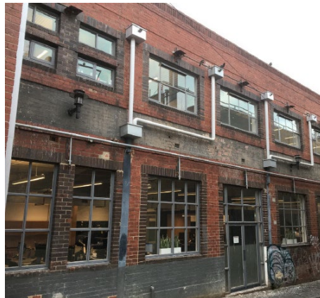
Recent photograph of the Little Pelham Street elevation
