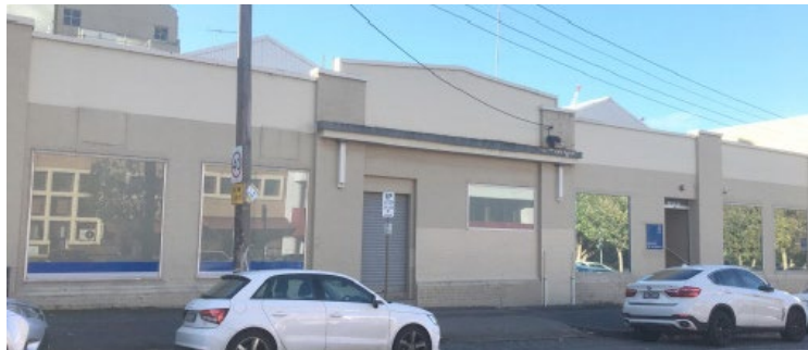
Recent photograph of the front façade to Pelham Street
