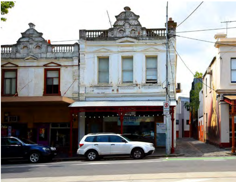
Figure 6 550 Queensbury Street before and after awning reconstruction.
