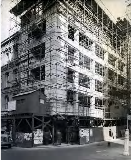
Figure 1. 103-105 Queen Street during construction work in September 1956. (Source: Cross-Section 1956)
