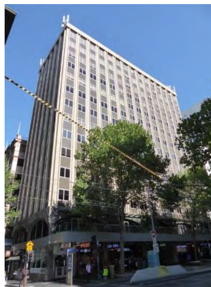
Former State Savings Bank of Victoria, 45-63 Swanston Street, (Buchan Laird & Buchan, 1974) included in HO505 Flinders Gate Precinct (Non-contributory).
