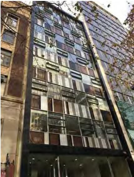
London Assurance House, 468-470 Bourke Street (Bernard Evans, 1960).
