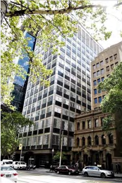
Former Reserve Bank of Australia, 56-64 Collins Street (Commonwealth Department of Works, 1964-66) included in HO504 Collins East Precinct as a Contributory place.
