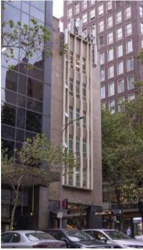
Former Ajax House, 103-105 Queen Street (HD Berry, 1956).
