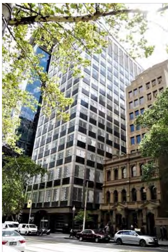
Former Reserve Bank of Australia, 56-64 Collins Street (Commonwealth Department of Works, 1964-66) included in HO504 Collins East Precinct as a Contributory place.
