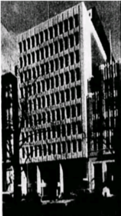
Figure 3. A 1998 photograph shows the building prior to its refurbishment in 2002, which saw the first floor extended to the building line and glazed. In the above image, the first floor is clearly recessed beneath the upper levels and the double height street level under-croft and colonnade is clearly intact. (Source: Age 16 September 1998:30)
