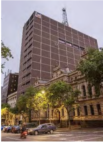
Lonsdale Exchange, 447-553 Lonsdale Street (Commonwealth Department of Works, 1969)
