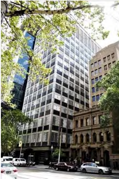
Former Reserve Bank of Australia, 56-64 Collins Street (Commonwealth Department of Works, 1964-66) included in HO504 Collins East Precinct as a Contributory place.
