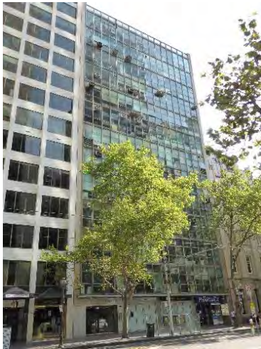
Coates Building, 18-22 Collins Street (John A La Gerche, 1958-59) included in HO504 Collins East Precinct as a Significant place.
