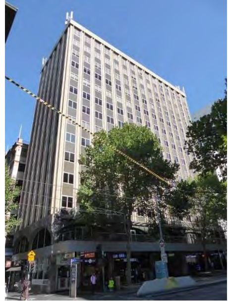
Former State Savings Bank of Victoria, 45-63 Swanston Street, (Buchan Laird & Buchan, 1974) included in HO505 Flinders Gate Precinct (Non-contributory).
