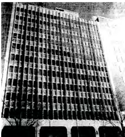
Figure 6. Image from a 1989 auction notice for one of the ground-level shops shows the original structure of the colonnade. (Source: Age 7 November 1989:33)
