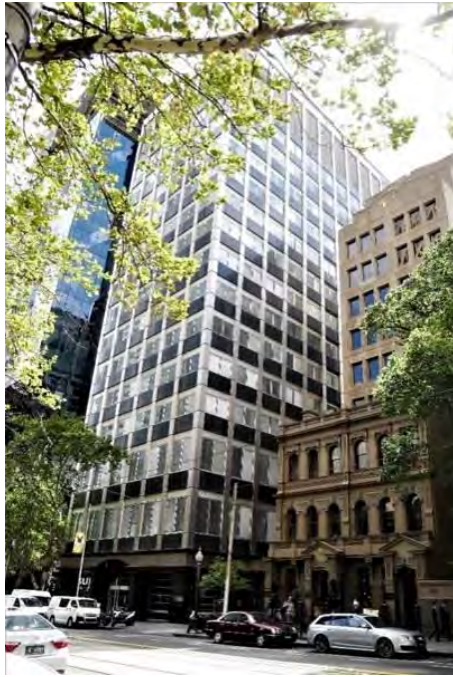
Former Reserve Bank of Australia, 56-64 Collins Street (Commonwealth Department of Works, 1964-66) included in HO504 Collins East Precinct as a Contributory place.
