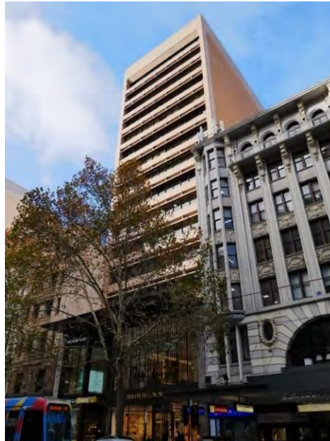
Former Commercial Banking Company of Sydney Building, 251-257 Collins Street, (Bates Smart & McCutcheon, 1974-73) included in HO502 The Block Precinct (fronting Collins Street) & HO506 (fronting Flinders Lane) (Non-contributory).
