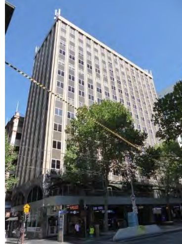
Former State Savings Bank of Victoria, 45-63 Swanston Street, (Buchan Laird & Buchan, 1974) included in HO505 Flinders Gate Precinct (Non-contributory).
