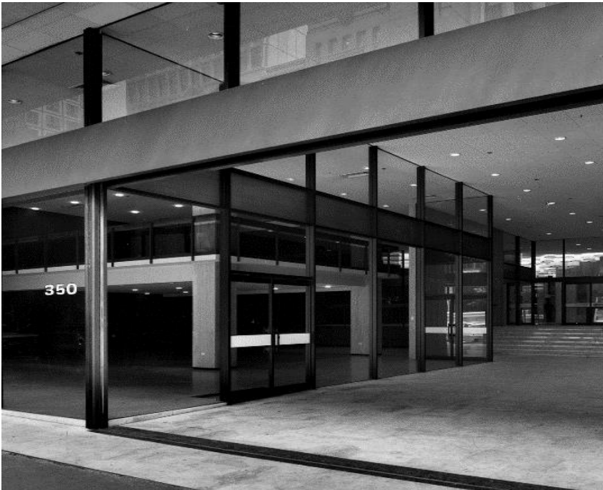
Figure 7. Part of the Collins Street entrance in 1975 (SLV, Wolfgang Sievers, photographer, Image H99.50/88).
