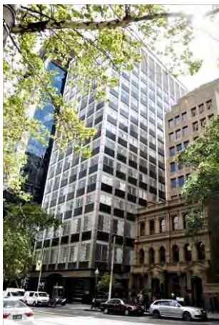
Former Reserve Bank of Australia, 56-64 Collins Street (Commonwealth Department of Works, 1964-66) included in HO504 Collins East Precinct as a Contributory place.
