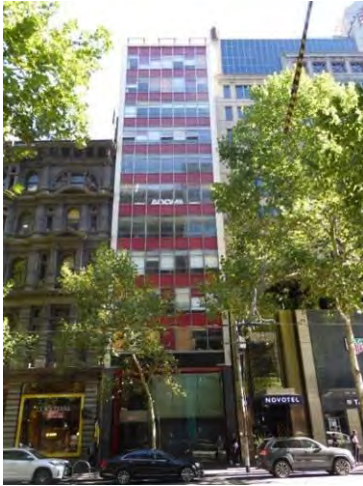
Former Allans Building, 276-278 Collins Street (Godfrey & Spowers, Hughes, Merton and Lobb with Charles N Hollinshed, 1956-57) included in HO502 The Block Precinct as a Significant place.
