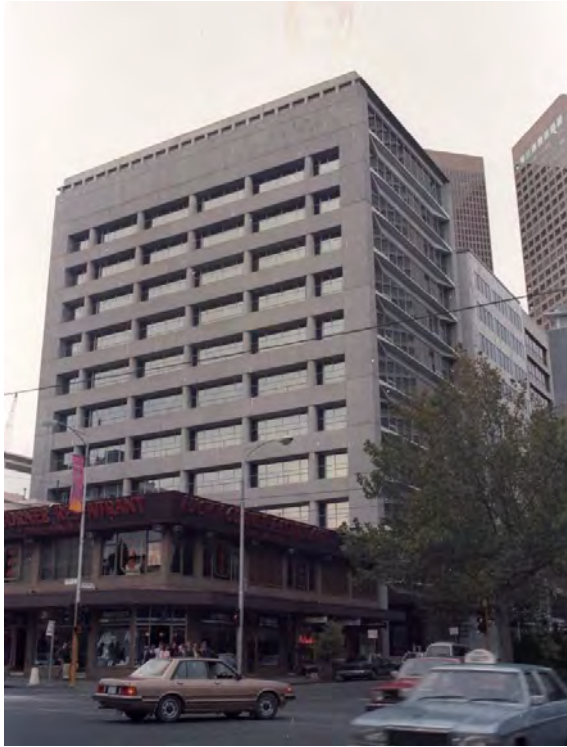
Figure 8. The building in 1984 (City of Melbourne Libraries online Heritage Collection, Reference no. Butler13724).
