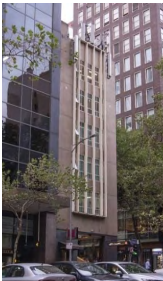
Former Ajax House, 103-105 Queen Street (HD Berry, 1956).
