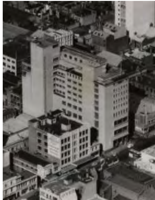
Figure 2. Aerial view of the Telephone Exchange and Postal Building, Russell Street, Melbourne, Victoria 1954-60. (Source: Charles Pratt and Airspy 1954-56, SLV copyright)
