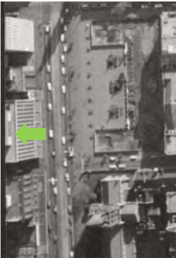
Figure 5. Detail of a 1976 aerial, showing the present State Savings Bank (SLV, Wolfgang Sievers, photographer, Image H2003.100/977).
