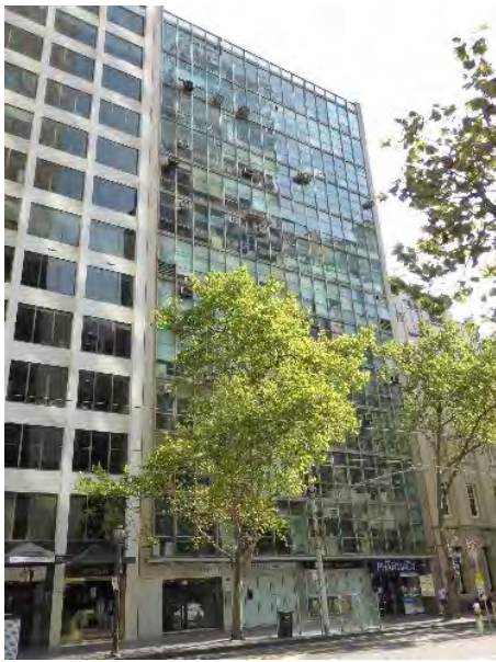
Coates Building, 18-22 Collins Street (John A La Gerche, 1958-59) included in HO504 Collins East Precinct as a Significant place.
