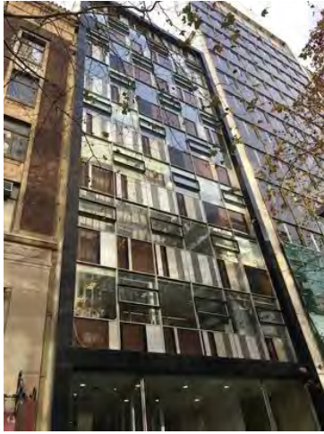
London Assurance House, 468-470 Bourke Street (Bernard Evans, 1960).
