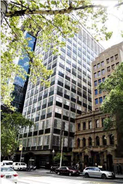
Former Reserve Bank of Australia, 56-64 Collins Street (Commonwealth Department of Works, 1964-66) included in HO504 Collins East Precinct as a Contributory place.
