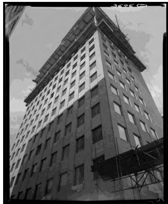
Figure 5. Houston Building nearing completion in 1965 (NLA, Wolfgang Sievers, photographer, object)
