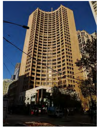
Former MLC Building, 303-317 Collins Street (Demaine, Russell, Trundle, Armstrong & Orton, c1970-1973)
