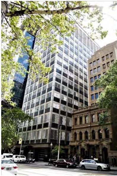
Former Reserve Bank of Australia, 56-64 Collins Street (Commonwealth Department of Works, 1964-66) included in HO504 Collins East Precinct as a Contributory place.
