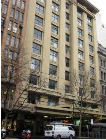
Figure 5. Capitol Arcade, 115 Swanston Street, built in 1924.
