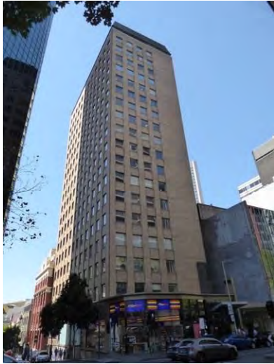
The Former Houston Building, 184-192 Queen Street (E & G Kolle & Associates, 1965)
