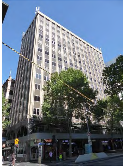
Former State Savings Bank of Victoria, 45-63 Swanston Street, (Buchan Laird & Buchan, 1974) included in HO505 Flinders Gate Precinct (Non-contributory).
