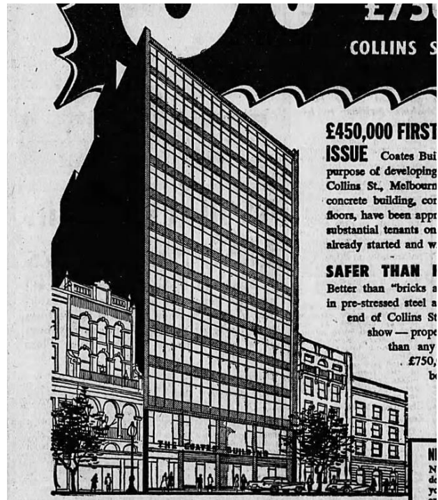
Figure 5. An illustration of the proposed design, published in July 1958 while the building was under construction ( Age , 30 Jul 1958:7).
