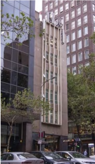
Former Ajax House, 103-105 Queen Street (HD Berry, 1956).
