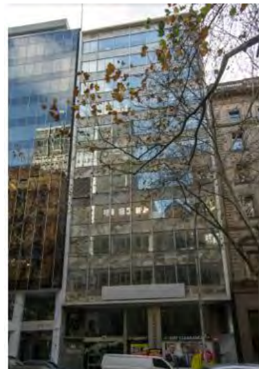
Former Atlas Assurance Building, 404-406 Collins Street (H Garnet Alsop & Partners, 1958-61) (Interim HO1008).
