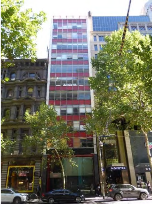
Former Allans Building, 276-278 Collins Street (Godfrey & Spowers, Hughes, Mewton & Lobb, 1956-57) included in HO502 The Block Precinct as a Contributory place.
