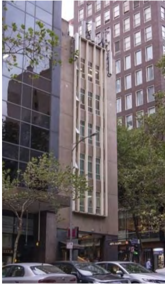
Former Ajax House, 103-105 Queen Street (HD Berry, 1956).
