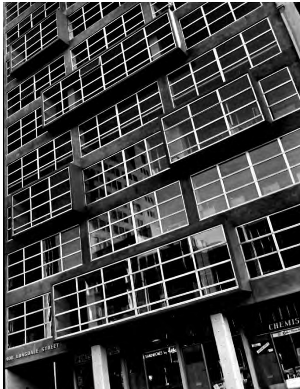
Figure 3. A detail of the facade in 1958 (SLV, Wolfgang Sievers, photographer, Image H99.50/27).
