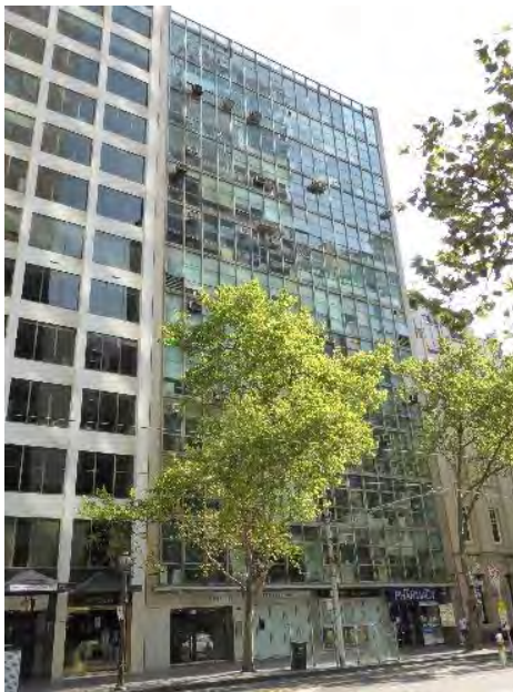
Coates Building, 18-22 Collins Street (John A La Gerche, 1958-59) included in HO504 Collins East Precinct as a Significant place.
