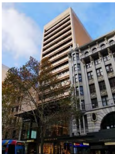
Former Commercial Banking Company of Sydney Building, 251-257 Collins Street, (Bates Smart & McCutcheon, 19741-73 included in HO502 The Block Precinct (fronting Collins Street) & HO506 (fronting Flinders Lane) (Non-contributory).
