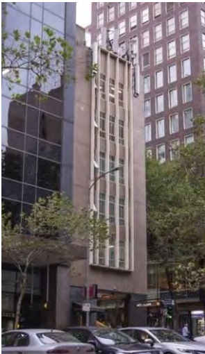
Former Ajax House, 103-105 Queen Street (HD Berry, 1956).
