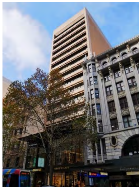
Former Commercial Banking Company of Sydney Building, 251-257 Collins Street, (Bates Smart & McCutcheon, 19741-73 included in HO502 The Block Precinct (fronting Collins Street) & HO506 (fronting Flinders Lane) (Non-contributory).
