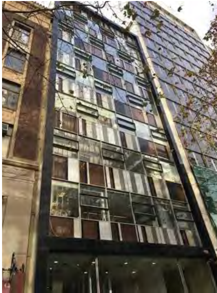
London Assurance House, 468-470 Bourke Street (Bernard Evans, 1960).
