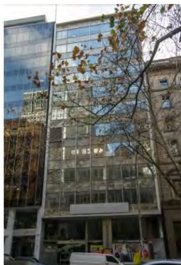
Former Atlas Assurance Building, 404-406 Collins Street (H Garnet Alsop & Partners, 1958-61) (Interim HO1008).
