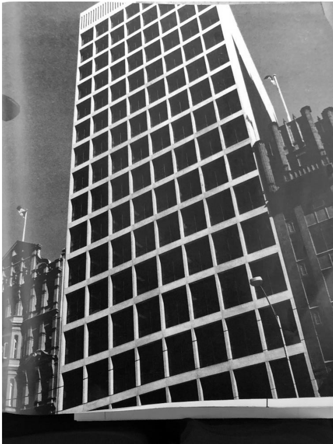
Figure 5. Photo of the building published in the Sep/Oct 1969 edition of Architect (Sep-Oct 1969:25).
