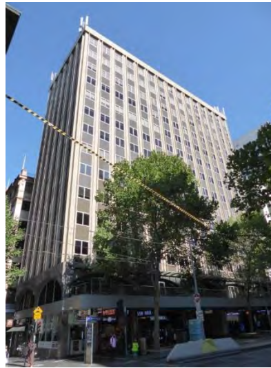
Former State Savings Bank of Victoria, 45-63 Swanston Street, (Buchan Laird & Buchan, 1974) included in HO505 Flinders Gate Precinct (Non-contributory).
