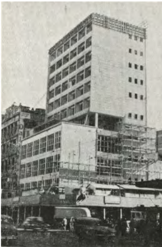
Figure 6. The construction phase, July 1955 ( Cross-Section , Jul 1955).
