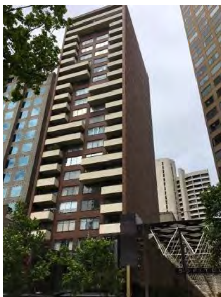
Apartment Building, 13-15 Collins Street (Kurt Popper, 1970) (Interim HO1265, & currently included as a Significant place in Collins East Precinct HO504)
