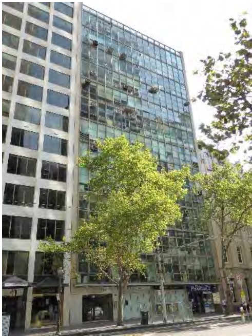
Coates Building, 18-22 Collins Street (John A La Gerche, 1958-59) included in HO504 Collins East Precinct as a Significant place.
