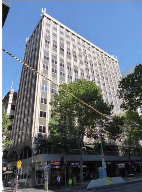
Former State Savings Bank of Victoria, 45-63 Swanston Street, (Buchan Laird & Buchan, 1974) included in HO505 Flinders Gate Precinct (Non-contributory).
