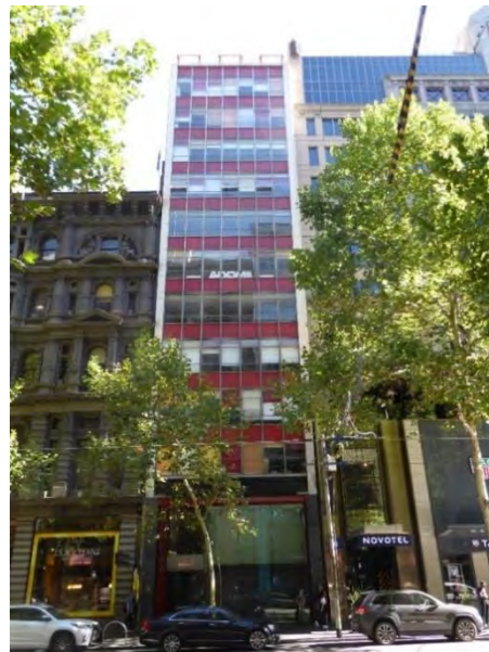
Former Allans Building, 276-278 Collins Street (Godfrey & Spowers, Hughes, Mewton & Lobb, 1956-1957) included in HO502 The Block Precinct as a Significant place.
