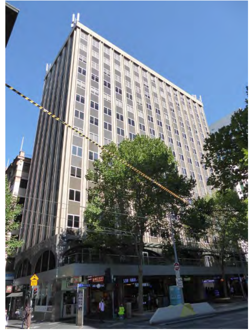
Former State Savings Bank of Victoria, 45-63 Swanston Street, (Buchan Laird & Buchan, 1974) included in HO505 Flinders Gate Precinct (Non-contributory).
