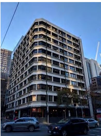
Office Building, 589-603 Bourke Street (Peddle Thorp
