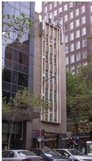
Former Ajax House, 103-105 Queen Street (HD Berry, 1956).
