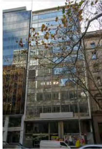
Former Atlas Assurance Building, 404-406 Collins Street (H Garnet Alsop & Partners, 1958-61) (Interim HO1008).
