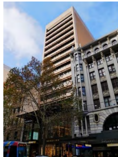
Former Commercial Banking Company of Sydney Building, 251-257 Collins Street, (Bates Smart & McCutcheon, 1974-73) included in HO502 The Block Precinct (fronting Collins Street) & HO506 (fronting Flinders Lane) (Non-contributory).
