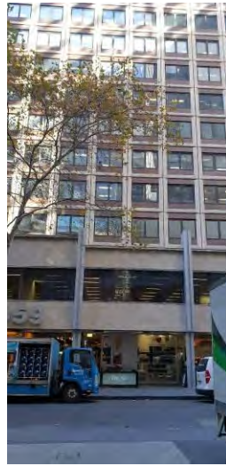
Cowan House, 457-469 Little Collins Street (E & G Koller, 1969)
