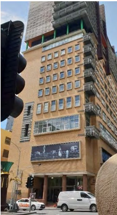
Figure 8. 114-120 Russell Street, built in 1948-1954. (Source: Context 2018)
