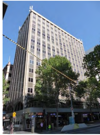
Former State Savings Bank of Victoria, 45-63 Swanston Street, (Buchan Laird & Buchan, 1974) included in HO505 Flinders Gate Precinct (Non-contributory).
