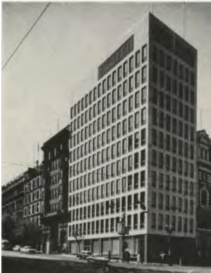
Figure 6. An image of the building published in 1962 ( Cross-Section No. 114, Apr 1962).
