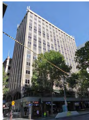
Former State Savings Bank of Victoria, 45-63 Swanston Street, (Buchan Laird & Buchan, 1974) included in HO505 Flinders Gate Precinct (Non-contributory).
