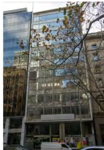
Former Atlas Assurance Building, 404-406 Collins Street (H Garnet Alsop & Partners, 1958-61) (Interim HO1008).
