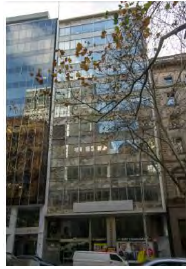
Former Atlas Assurance Building, 404-406 Collins Street (H Garnet Alsop & Partners, 1958-61) (Interim HO1008).
