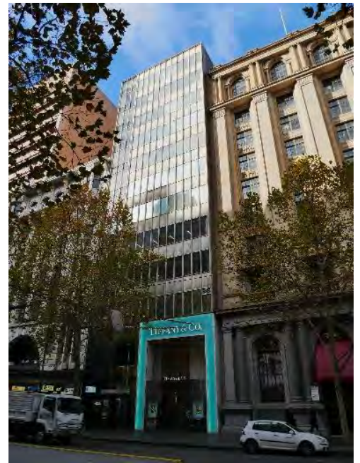
Former Bank of Adelaide Building, 265-269 Collins Street (Godfrey & Spowers, Hughes, Mewton & Lobb, 1959-60) included in HO502 The Block Precinct as a Contributory place.
