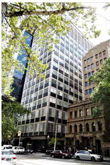
Former Reserve Bank of Australia, 56-64 Collins Street (Commonwealth Department of Works, 1964-66) included in HO504 Collins East Precinct as a Contributory place.
