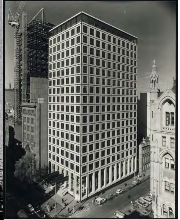
Figure 4. Photograph showing Legal & General House completed. (Source: Crothers 1967, SLV)
