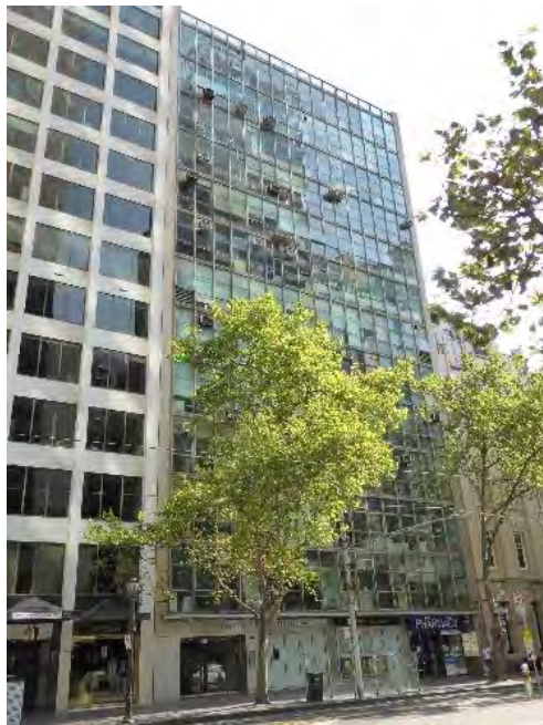
Coates Building, 18-22 Collins Street (John A La Gerche, 1958-59) included in HO504 Collins East Precinct as a Significant place.
