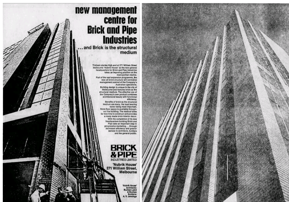
Figure 3. A 1972 advertisement showing the newly erected Nubrik House viewed from the southwest (left) and another 1972 photograph showing the view from southeast (right). (Source: Age 6 November 1972:24; Age 18 December 1972:13)
