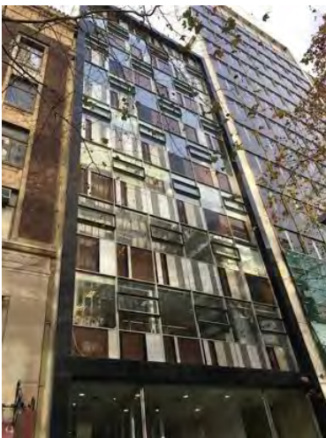
London Assurance House, 468-470 Bourke Street (Bernard Evans, 1960).
