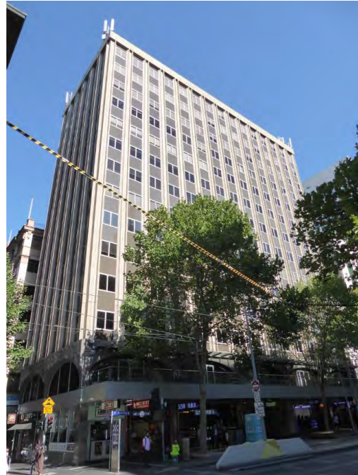
Former State Savings Bank of Victoria, 45-63 Swanston Street, (Buchan Laird & Buchan, 1974) included in HO505 Flinders Gate Precinct (Non-contributory).
