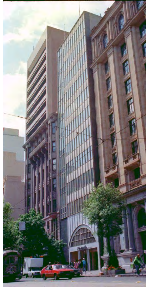
Figure 6. The building in 1984 with an altered ground floor shopfront (City of Melbourne Libraries online Heritage Collection, Reference no. Butler13528).
