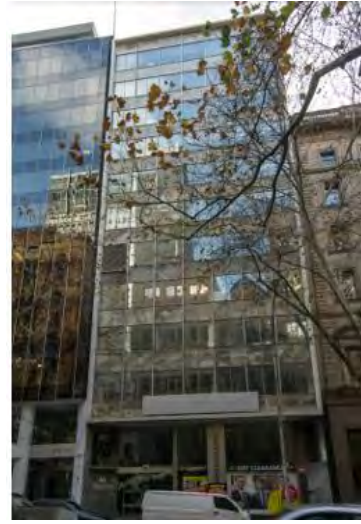
Former Atlas Assurance Building, 404-406 Collins Street (H Garnet Alsop & Partners, 1958-61) (Interim HO1008).
