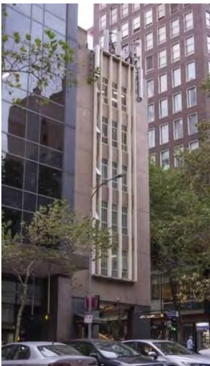
Former Ajax House, 103-105 Queen Street (HD Berry, 1956).
