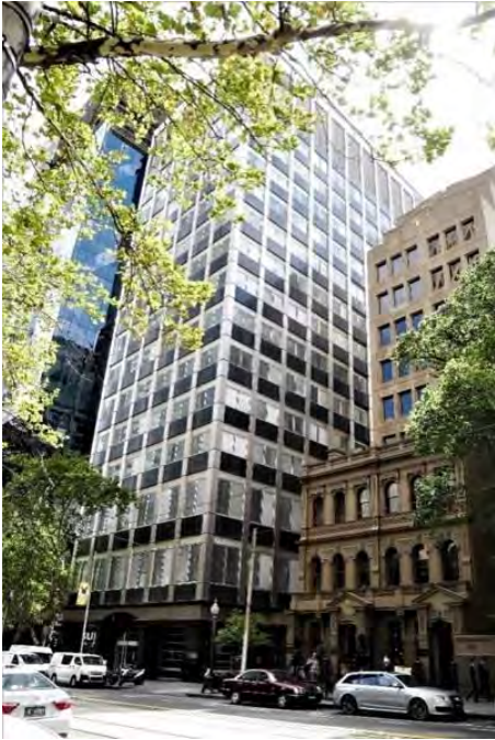
Former Reserve Bank of Australia, 56-64 Collins Street (Commonwealth Department of Works, 1964-66) included in HO504 Collins East Precinct as a Contributory place.
