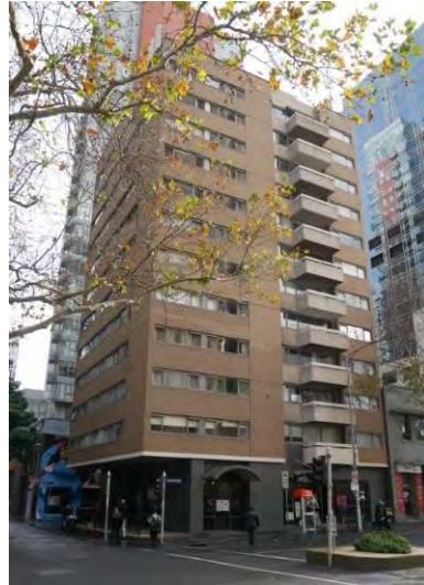
Exhibition Towers, 287-293 Exhibition Street (Kenneth McDonald & Associates, 1969-71)
