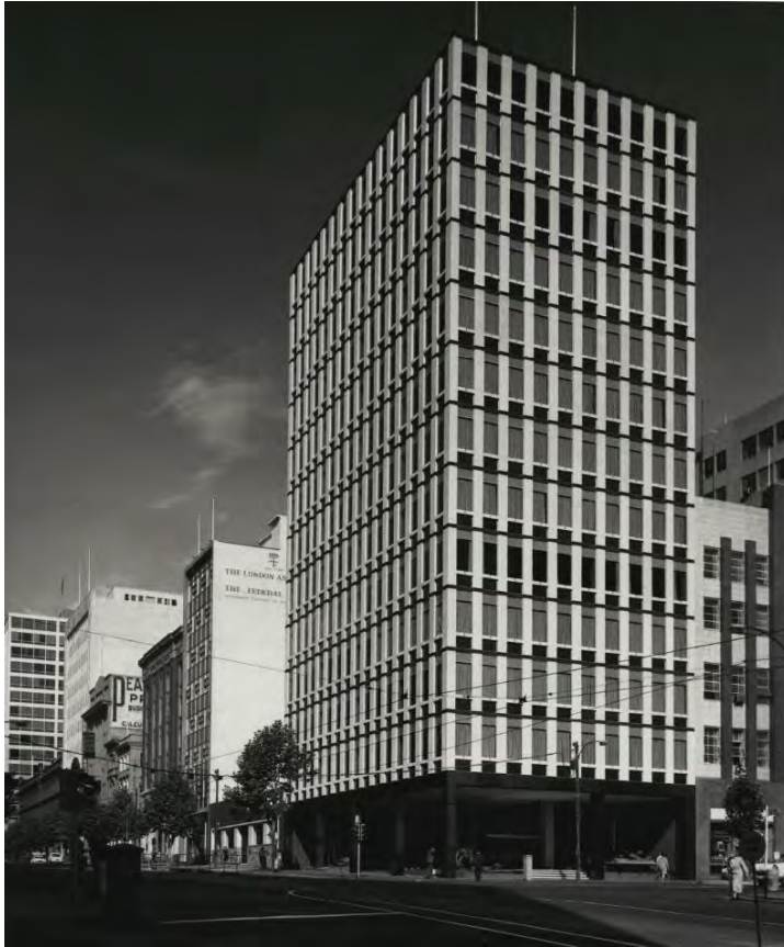
Figure 1. South British Insurance building, corner of Bourke and Queen Streets, 1961. (Source: Sievers 1961, SLV copyright)
