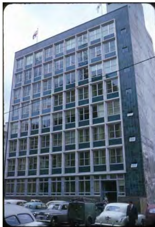
Figure 2. The building as it was soon after construction, faced in blue tiles. The building was actually constructed to be eight stories, rather than the initial seven. (Source: 'HC Sleigh and Co, 1957, NAA)
