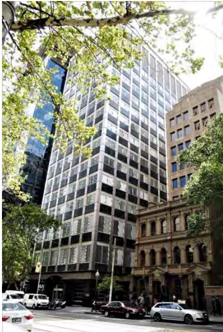
Former Reserve Bank of Australia, 56-64 Collins Street (Commonwealth Department of Works, 1964-66) included in HO504 Collins East Precinct as a Contributory place.
