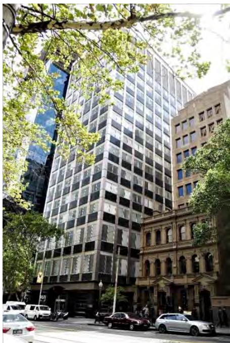
Former Reserve Bank of Australia, 56-64 Collins Street (Commonwealth Department of Works, 1964-66) included in HO504 Collins East Precinct as a Contributory place.
