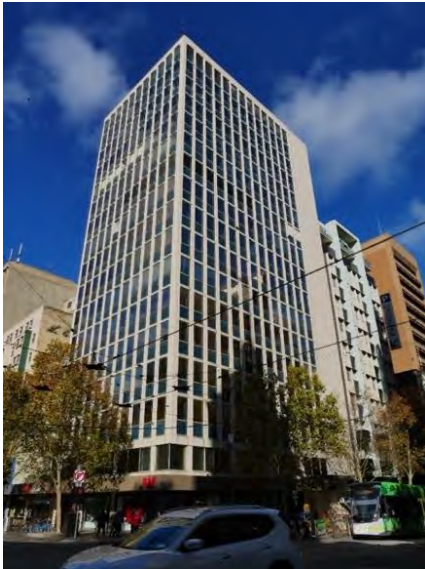
Wales Corner, 221-231 Collins Street (Stephenson & Turner, 1964-66) included in HO502 The Block Precinct (fronting Collins Street) & HO506 (fronting Swanston Street) Collins East Precinct as a Contributory place.
