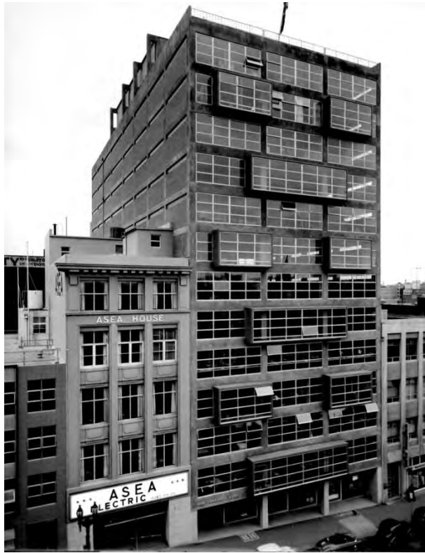
Figure 2. The newly completed building in 1958 (SLV, Wolfgang Sievers, photographer, Image H99.50/26).
