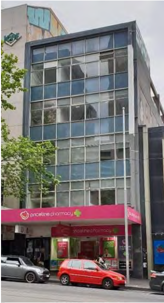
Former Ajax House, 103-105 Queen Street (HD Berry, 1956).
