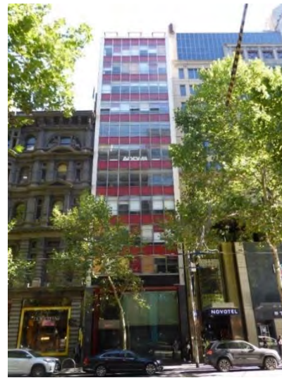
Former Allans Building, 276-278 Collins Street (Godfrey & Spowers, Hughes, Mewton & Lobb, 1956-57) included in HO502 The Block Precinct as a Significant place.
