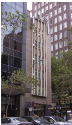
Former Ajax House, 103-105 Queen Street (HD Berry, 1956).
