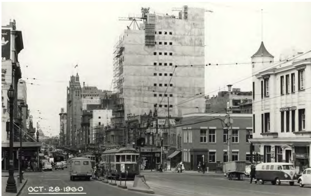
Figure 1. State Bank building, corner Little Bourke and Swanston streets under construction, 28 October 1960. (Source: Commercial Photographic Co 1960, SLV)
