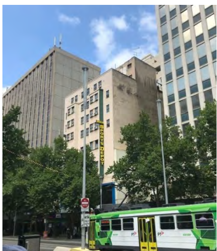
Figure 15. The Graham Hotel (GJM Heritage, February 2020)
