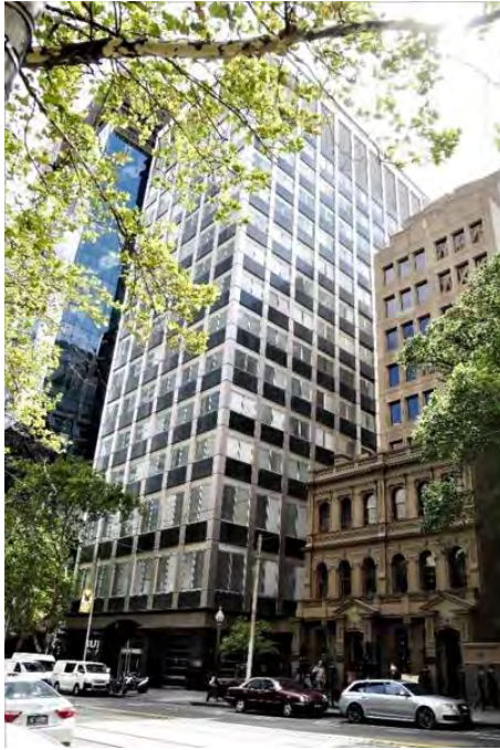
Former Reserve Bank of Australia, 56-64 Collins Street (Commonwealth Department of Works, 1964-66) included in HO504 Collins East Precinct as a Contributory place.
