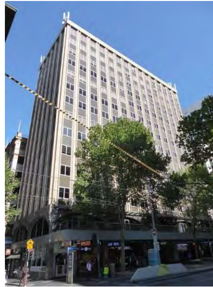
Former State Savings Bank of Victoria, 45-63 Swanston Street, (Buchan Laird & Buchan, 1974) included in HO: Flinders Gate Precinct (Non-contributory).
