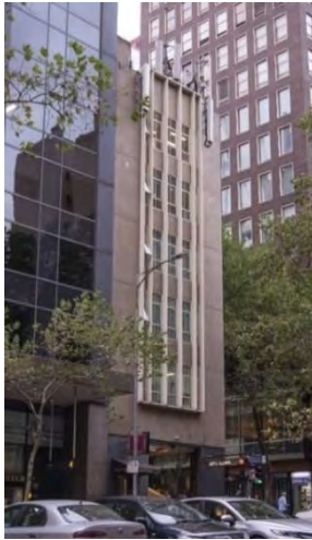
Former Ajax House, 103-105 Queen Street (HD Berry, 1956).
