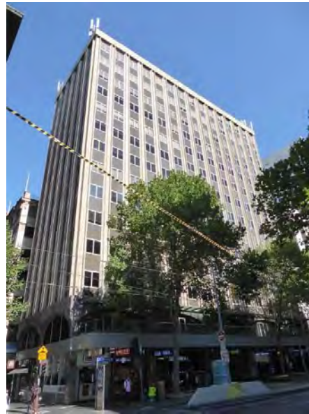
Former State Savings Bank of Victoria, 45-63 Swanston Street, (Buchan Laird & Buchan, 1974) included in HO505 Flinders Gate Precinct (Non-contributory).
