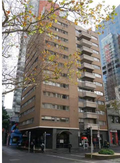
Exhibition Towers, 287-293 Exhibition Street (Kenneth McDonald & Associates, 1969-71)
