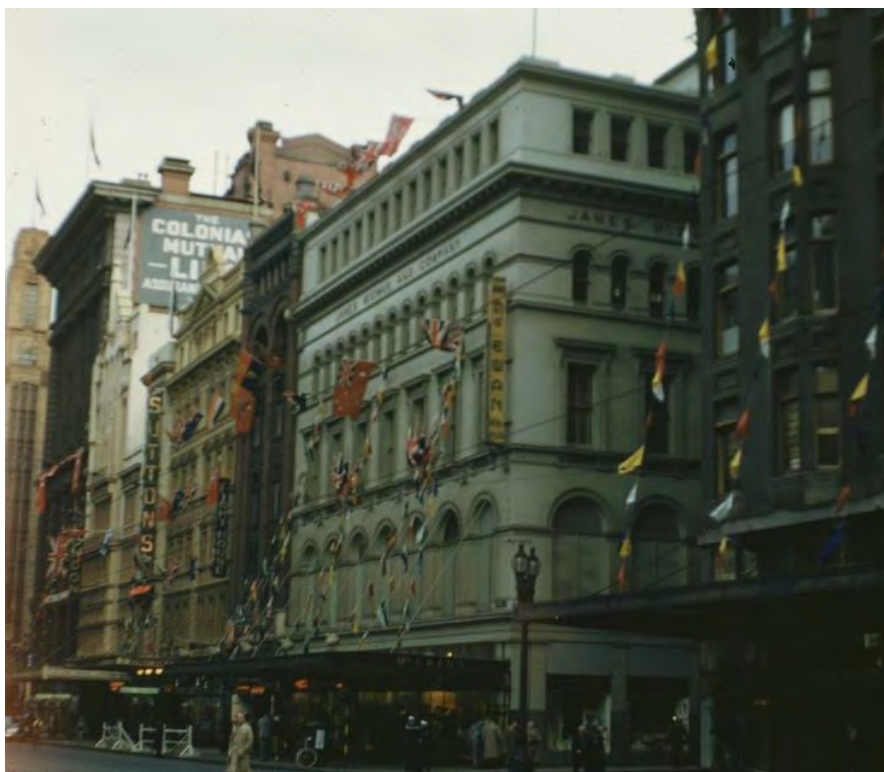
Figure 1. Showing the five-storey 1870 McEwan's building (demolished c1967) facing Elizabeth Street at the corner of Little Collins Street in 1953. (Source: Gordon 1953, SLV)
