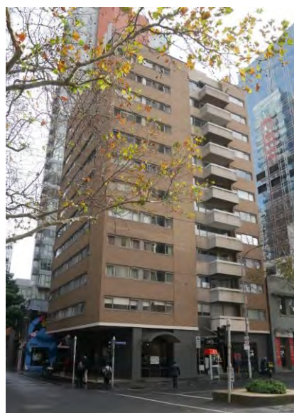
Exhibition Towers, 287-293 Exhibition Street (Kenneth McDonald & Associates, 1969-71)
