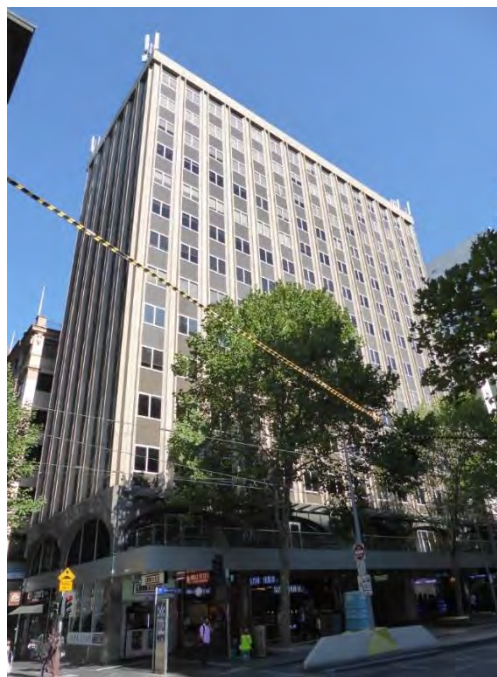
Former State Savings Bank of Victoria, 45-63 Swanston Street, (Buchan Laird & Buchan, 1974) included in HO505 Flinders Gate Precinct (Non-contributory).
