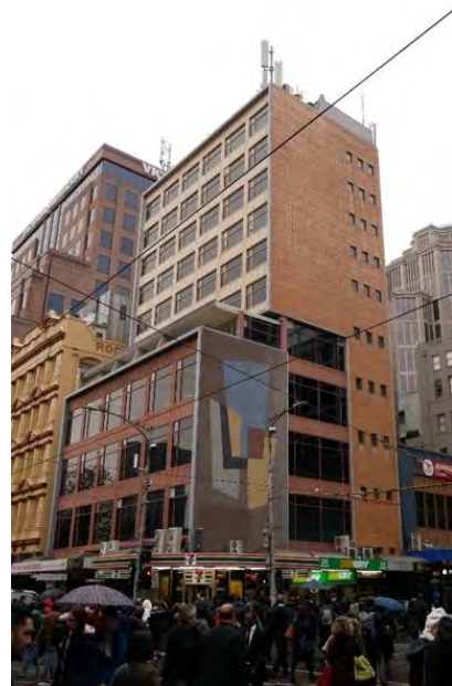
Former Hosie's Hotel, 1-5 Elizabeth Street & 288-290 Flinders Street (Mussen McKay & Potter, 1954-55), included in HO505 Flinders Gate Precinct as a Significant place.
