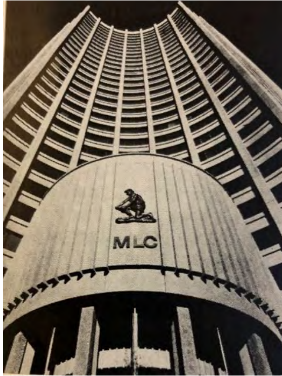
Figure 4. Photo of the building published in the May/June edition of Architecture in Australia (AIA, May/Jun 1973:8).
