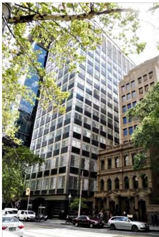
Former Reserve Bank of Australia, 56-64 Collins Street (Commonwealth Department of Works, 1964-66) included in HO504 Collins East Precinct as a Contributory place.
