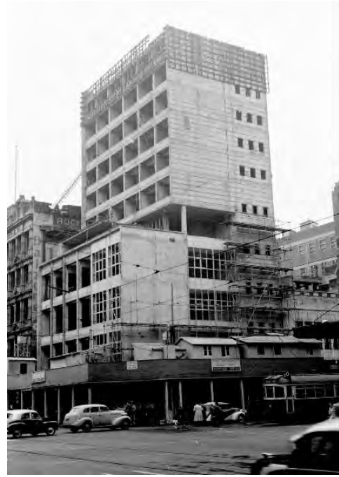
Figure 5. Construction phase, in 1955 (SLV, Mark Strizic, photographer, Image H2008.11/1086).
