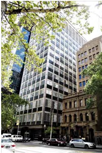
Former Reserve Bank of Australia, 56-64 Collins Street (Commonwealth Department of Works, 1964-66) included in HO504 Collins East Precinct as a Contributory place.
