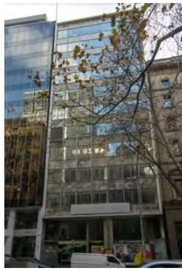
Former Atlas Assurance Building, 404-406 Collins Street (H Garnet Alsop & Partners, 1958-61) (Interim HO1008).
