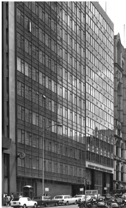
Figure 1. The Union Insurance Society of Canton Ltd building at 43-51 Queen Street in 1970 showing the clock at its southern end (Source: Sievers, 1970 SLV copyright )
