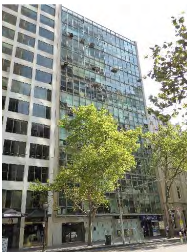
Coates Building, 18-22 Collins Street (John A La Gerche, 1958-59) included in HO504 Collins East Precinct as a Significant place.
