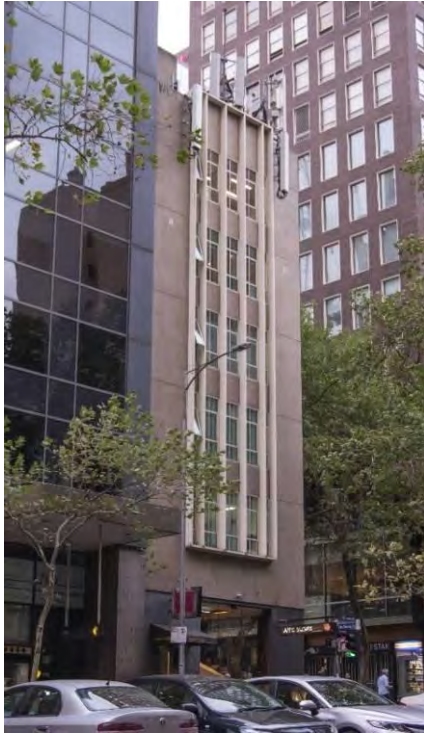
Former Ajax House, 103-105 Queen Street (HD Berry, 1956).
