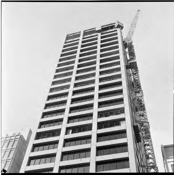
Figure 6. The tower under construction; photo dated c1975 (SLV, Hans Bonney, photographer, Image H2009.50/262).
