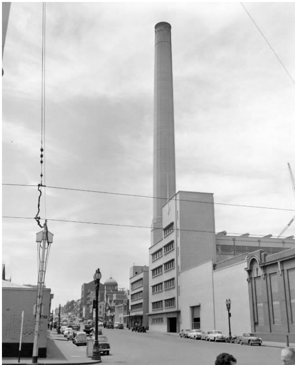
Figure 6. View of the power station buildings along Lonsdale Street, showing the Substation J brick building (with windows bricked in) (far right) and the new 1950s reinforced concrete buildings and tower to the east. (Source: Richards 1957, Museums Victoria in copyright )
