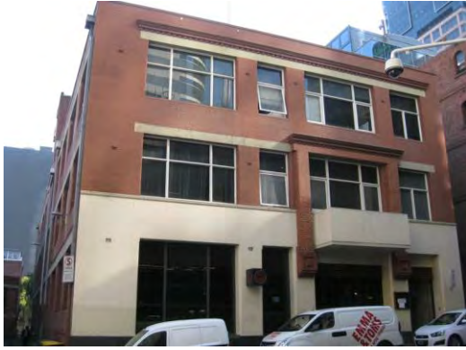
Figure 7. 562-566 Little Bourke Street, built in the 1920s.
