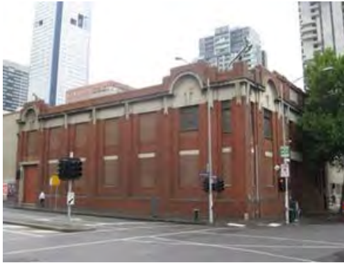
Figure 2. Substation at 651-669 Lonsdale Street constructed 1915.
