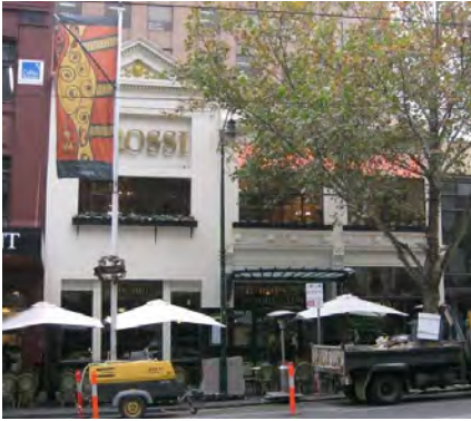
Figure 4. Grossi Florentino, 78-84 Bourke Street, built in 1860 & 1922.
