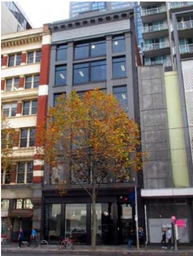
Figure 5. 96-98 Flinders Street, built in 1915. (Source: Context 2017).
