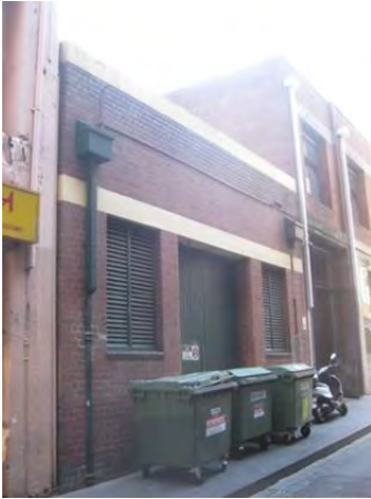
Figure 5. Substation at 28 Crossley Street, unknown built date.
