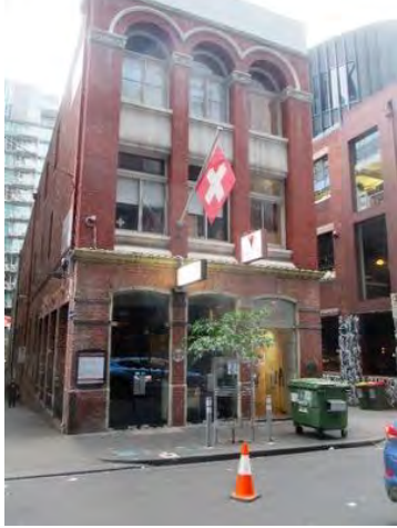
Figure 7. 87-89 Flinders Lane Melbourne, built in 1906. (Source: Context, May 2017)
