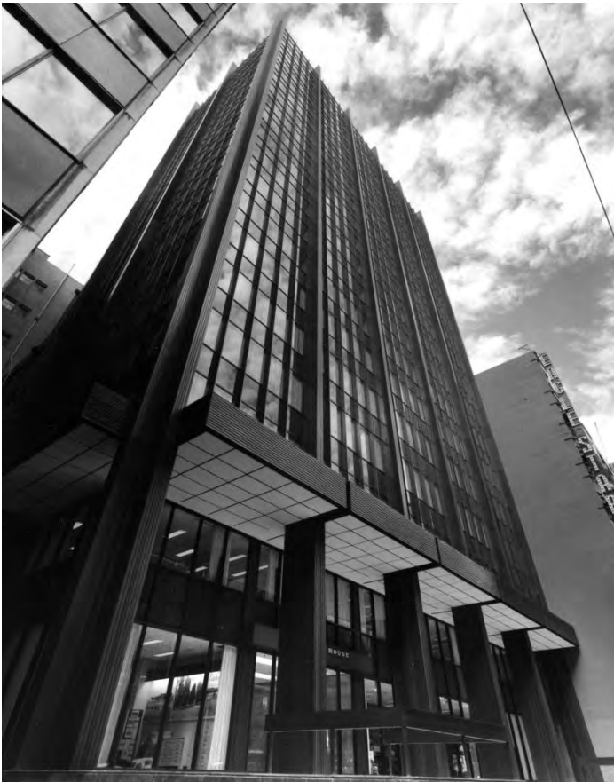
Figure 7. The building in 1969 (SLV, Wolfgang Sievers, photographer, Image H99.50/368).
