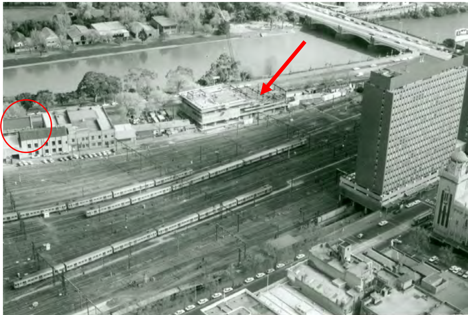
Figure 4. View of Jolimont Railway Yards from ANZ Tower, 1979, showing subject building (circled), Metro train control facility under construction (arrow) and Princes Gate tower to the right. (Source: Culture Victoria website).
