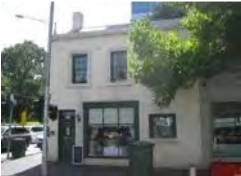
Figure 5. 330 King Street constructed 1850.
