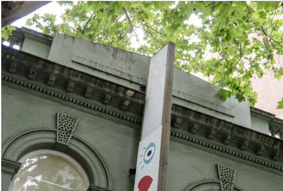
Figure 6. Close-up view of the refined upper-level detailing including the parapet and open balustrade, cornice supported on acanthus leaf brackets with a line of fine dentils below, and semi-circular arched windows with vermiculated keystone. (Source: Context, January 2020)
