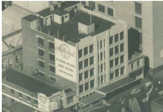
Figure 3 1950s, showing the verandah in its current condition and the original windows to the upper levels. (Source: CD Pratt, SLV)
