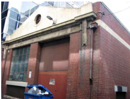
Figure 8. Substation, 10-14 Park Street constructed 1928. (Source: Context 2017)
