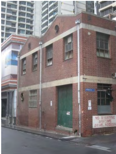
Figure 3. Substation at 620-648 Little Bourke Street constructed 1910-1925.
