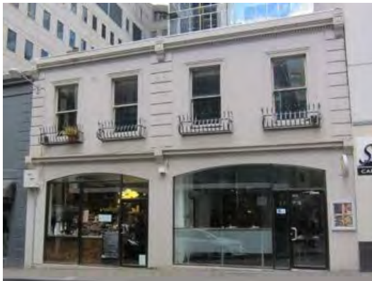
Figure 2. 470-472 Little Lonsdale Street constructed 1872.
