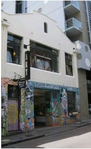
Figure 9 34-36 Little Latrobe Street, built in 1929.
