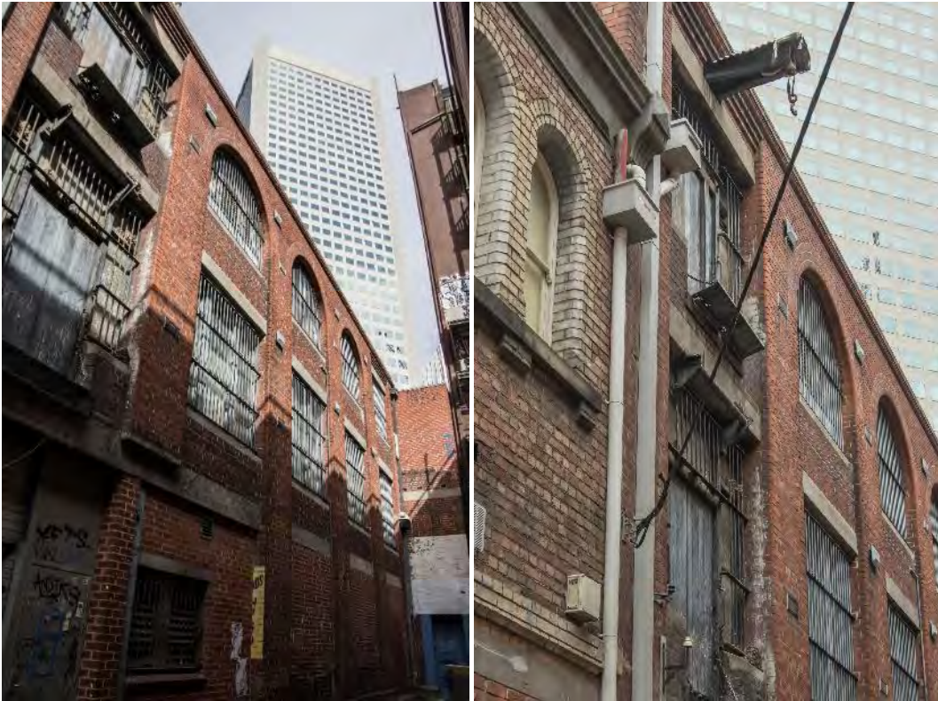
Figure 9. The 1912 warehouse fronting Warburton Lane, at the rear of 384-386 Bourke Street (left). Note the upper-level detailing of the Warburton Lane warehouse, including the corbel heads detailing above each end bay, timber loading doors and a hoist (right). (Source: Context, March 2019)
