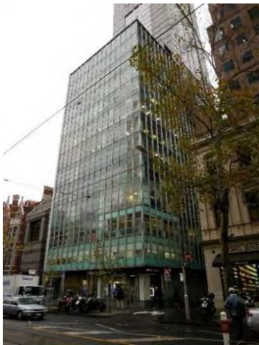
Former Gilbert Court, 100-104 Collins Street (John A La Gerche, 1954-55) included in HO504 Collins East Precinct as a Significant place.
