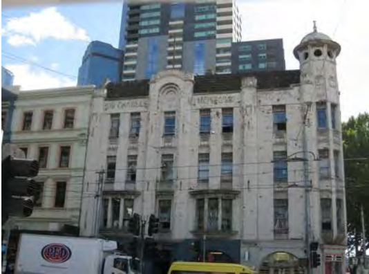
Figure 2. 2-8 Spencer Street, built in 1913.
