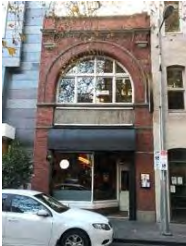
Figure 4. 37 Little Collins Street constructed. (Source: CoM, 2018)
