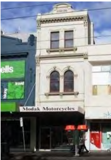
Figure 22. 299 Elizabeth Street, constructed 1885. (Source: CoMMaps)
