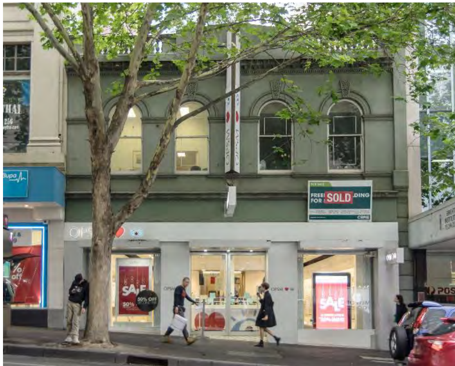
Figure 5. Bourke Street elevation of 384-386 Bourke Street. Note the unusual moulded string course that runs between each pair of upper-level windows at the sill level. (Source: Context, January 2020)
