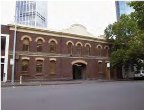
Figure 3. 61-69 A'Beckett Street constructed 1871.
