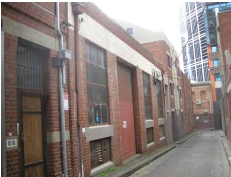
Figure 6. 12-14 Guildford Lane, substation constructed c1920.
