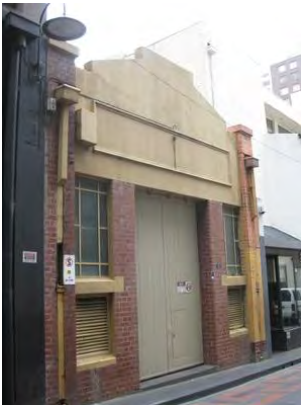
Figure 7. 21 Market Lane, unknown built date
