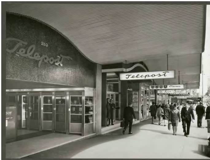
Figure 7. A 1967 photo showing the shopfronts and soffit of the canopy (SLV, Wolfgang Sievers, photographer, Image H98.30/237).
