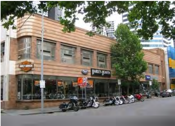
Figure 9. 111-125 A'Beckett Street, built in 1936.
