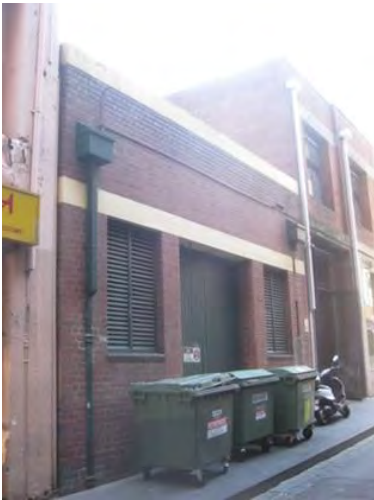
Figure 5. Substation at 28 Crossley Street, unknown build date.
