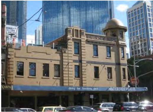
Figure 7. 508-514 Flinders Street, built in 1925.
