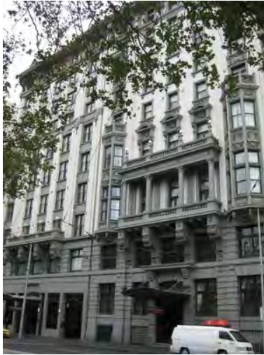
Figure 7. 318-324 Flinders Street, built in 1913.
