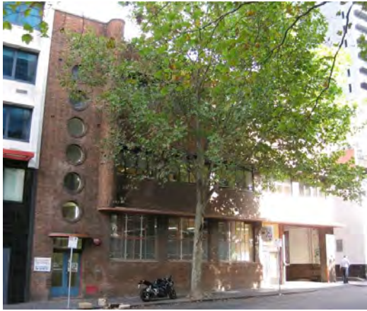
Figure 5. 185-187 A'Beckett Street, built in 1937.
