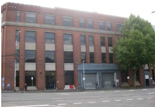
Figure 7. 258-274 Queensberry Street, Carlton, built in 1928.
