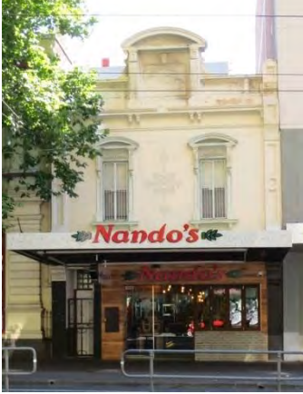
Figure 7. 380 Elizabeth Street, built c1850s, façade 1888
