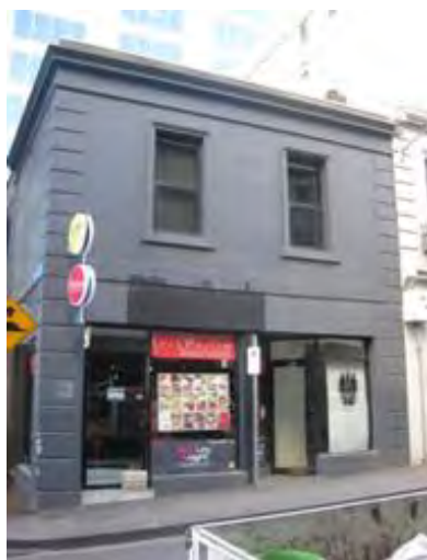
Figure 1. 474 Little Lonsdale Street constructed 1879.
