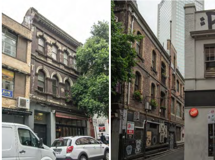
Figure 25, 365-367 Little Bourke Street, built in 1887, showing the front elevation (left) and rear warehouses (right). (Source: Context, January 2020)
