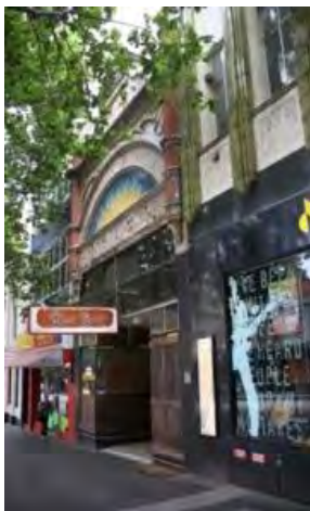
Figure 2. Exhibition Boot Company, 160-162 Bourke Street constructed 1904.
