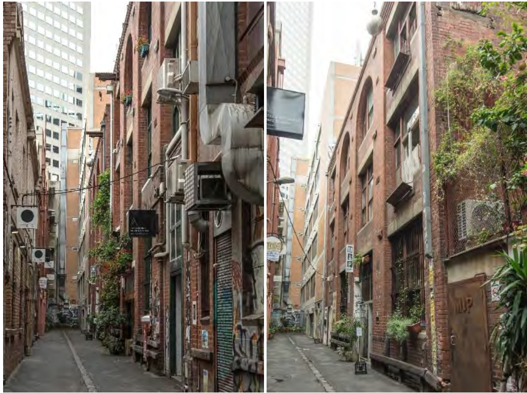
Figure 10. 2-6 and 8-14 Rankins Lane (left) and 8-14 Rankins Lane (right). (Source: Context, January 2020)
