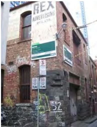
Figure 7. 32-34 Guildford Lane constructed 1908 & 1920.
