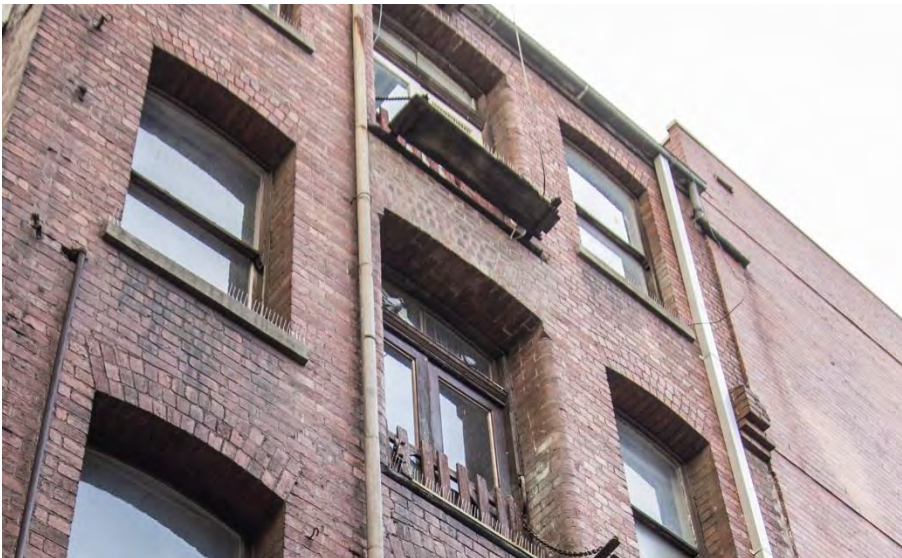
Figure 22. Note the remnant corbelled bracket on the northern (RHS) edge of the second floor of 3 Kirks Lane. (source: Context, January 2019)
