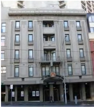
Figure 4. 66-70 Spencer Street, built in 1926-28.
