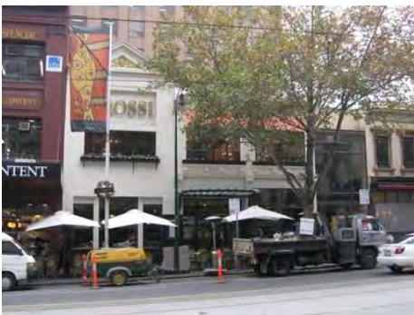
Figure 6. 78-84 Bourke Street constructed 1860 and 82-84 Bourke Street constructed 1922.
