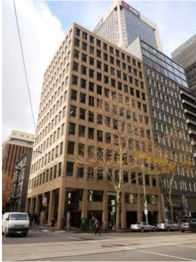
Office Building, 178-188 William Street (McIntyre McIntyre & Partners, 1972-73)
