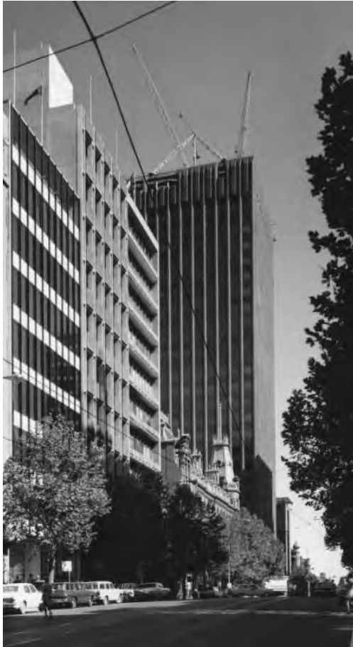
Figure 8. The AMP Tower under construction in 1969 (NLA, Wolfgang Sievers, photographer, object 160948175).
