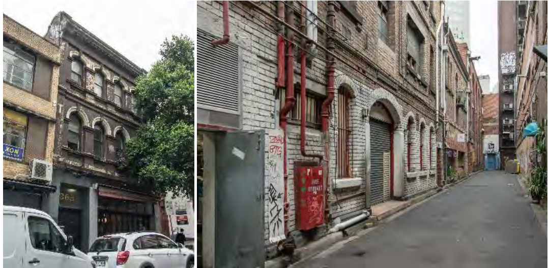
Figure 7. Little Bourke Street elevation (left) and Warburton Lane elevation (right) of 365-367 Little Bourke Street. (Source: Context, January 2020)
