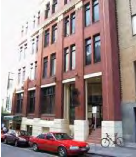
Figure 7. 401-405 Little Bourke Street, built in 1911 and remodelled in 1933.
