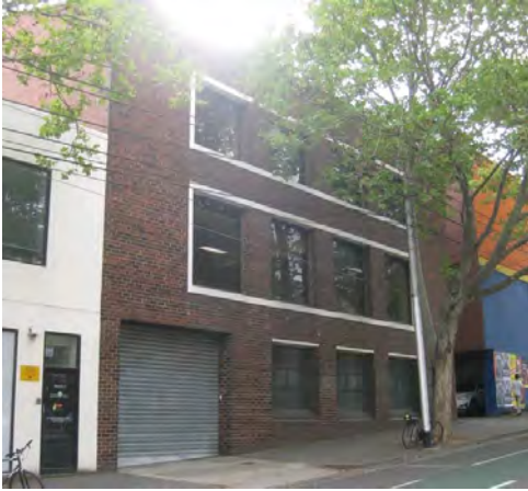
Figure 8. 198-202 Queensberry Street, Carlton, built in 1943.
