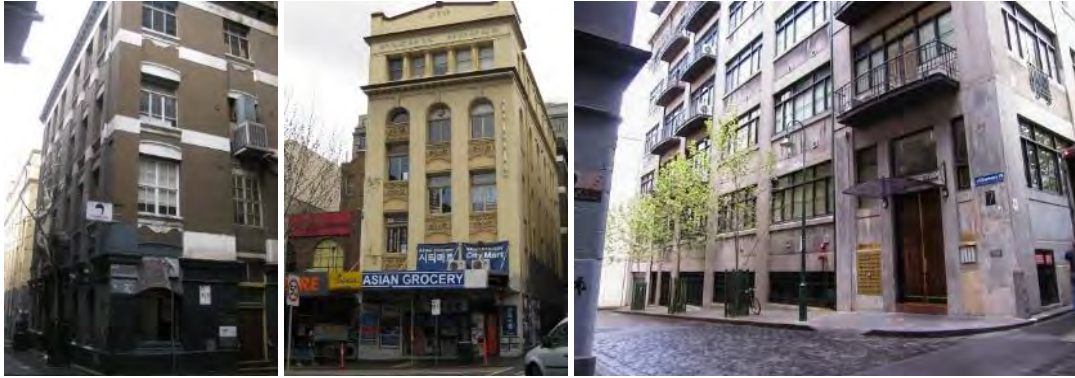
Figure 14. 2-20 Drewery Place, built in 1890 (left), 268-270 Lonsdale Street (middle) and 5-7 Drewery Lane (right).
