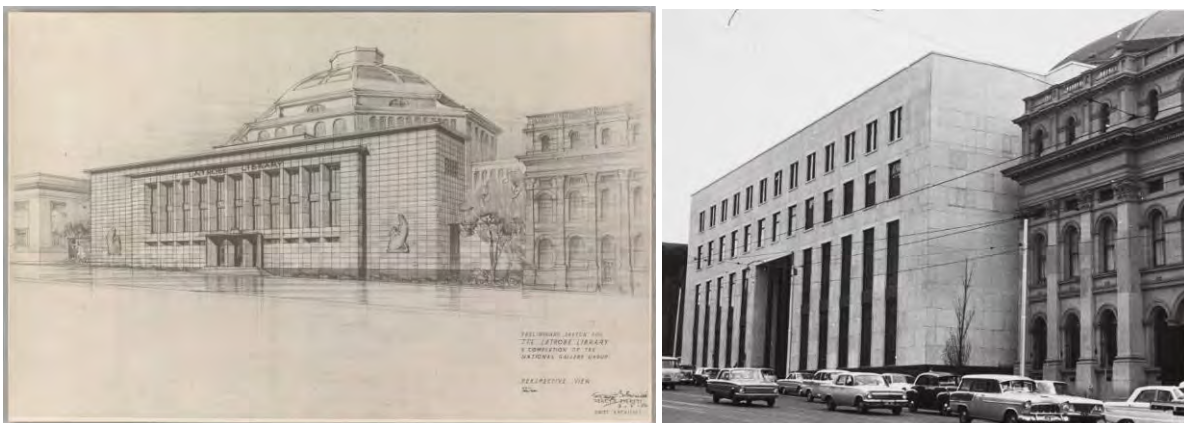
Figure 9 and 10. Preliminary sketch of the proposed La Trobe Library, 1950 and the completed design, 1964 (State Library of Victoria H28187 and H30064)
