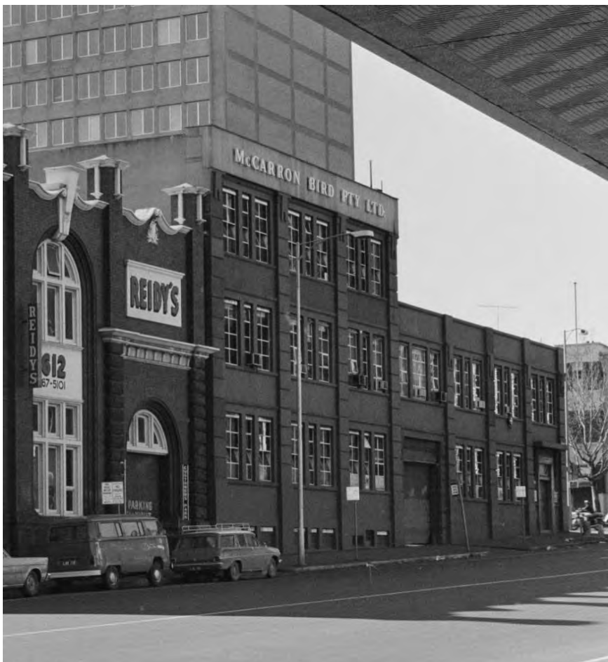
Figure 4. Extract of a photograph showing the subject building c1960s, then occupied by McCarron Bird Pty Ltd printers. (Source: K J Halla c1960s, SLV copyright)
