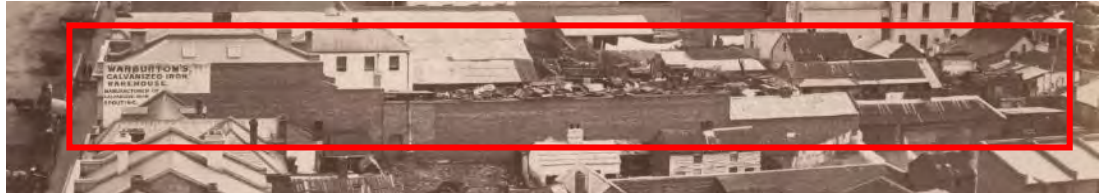
Figure 1. Extract of a c1870 photograph showing the premises of Thomas Warburton outlined in red (then addressed as 23-25 Bourke Street West). (Source: Nettleton c1870, SLV)
