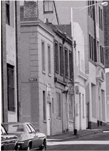
Figure 1. 472-470 Little Lonsdale shown in a section of Little Lonsdale Street North between Eagle Alley and William Street, Melbourne, Vic, c.1960-1969, by Halla (Source: SLV).
