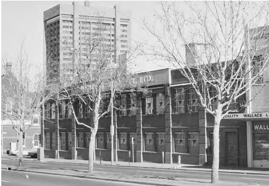
Figure 3. Extract of a photograph showing the subject building (McCarron Bird Pty Ltd) c1960s, looking southwest from King Street. (Source: K J Halla c1960s, SLV copyright)
