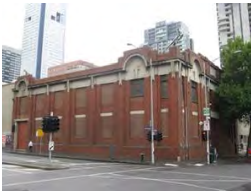
Figure 2. Substation at 651-669 Lonsdale Street constructed 1915.
