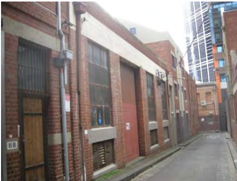
Figure 6., Substation at 12-14 Guildford Lane constructed c1920.
