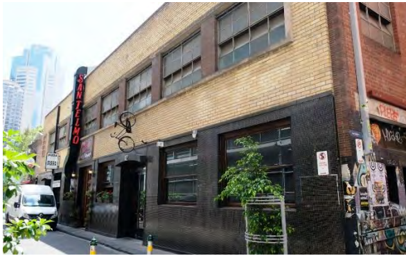
Figure 12. 12-18 Meyers Place, built in 1940. (Source: Context 2018)
