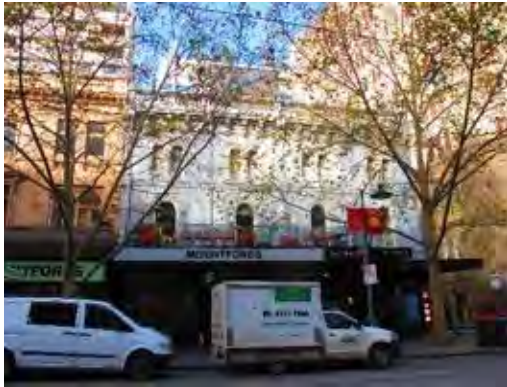
Figure 5. 209-215 Bourke Street constructed 1876. (Context 2018)
