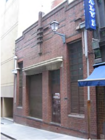
Figure 17. 23-25 George Parade, constructed in 1938. (Source: Context 2017)
