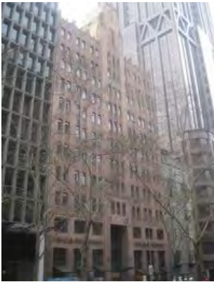
Figure 5. ACA Building, 118-126 Queen Street constructed 1936.
