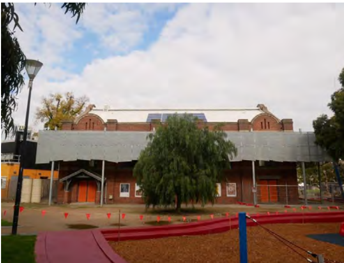
Figure 25. North elevation of the Former Princes Bridge Lecture Room, showing later external screen. (Source: GJM Heritage May 2020)
