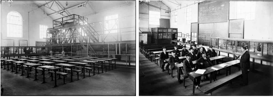
Figures 13 & 14. Photographs of the interior of the Princes Bridge Lecture Room, undated (Source: PROV, VPRS 12903/P1 item 012)
