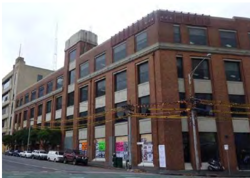
Figure 5. 258-274 Queensberry Street, Carlton, built in 1928.
