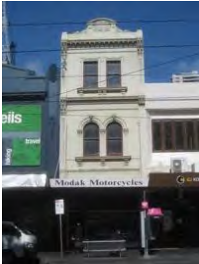
Figure 5. 299 Elizabeth Street constructed 1885.
