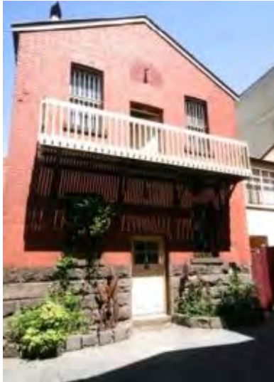
Figure 8. West wing of Currie & Richards showrooms & warehouses constructed c1900. (Source: Butler 2011:221)
