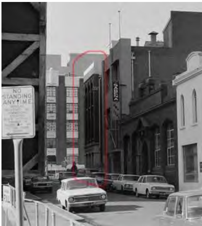
Figure 2. 87-89 Flinders Lane shown in a section of Flinders Lane south, c1972, by K J Halla. (Source: SLV)
