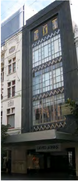
Figure 6. Former Buckley & Nunn Men's Wear store constructed 1933.
