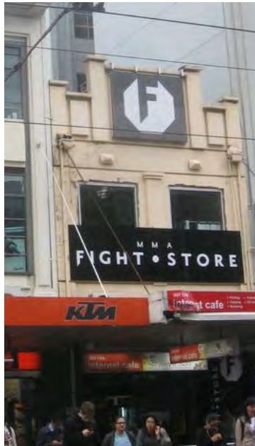
Figure 10. 349 Elizabeth Street, built in c1920s.
