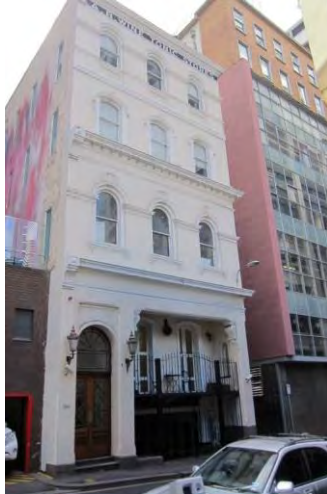
Figure 9. 384-386 Flinders Lane constructed 1885 and 1888. (Source: Context 2018)
