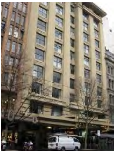
Figure 3. Capitol Arcade, 115 Swanston Street constructed 1924.
