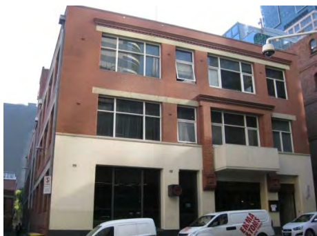
Figure 3. 562-566 Little Bourke Street, constructed in c1920s.
