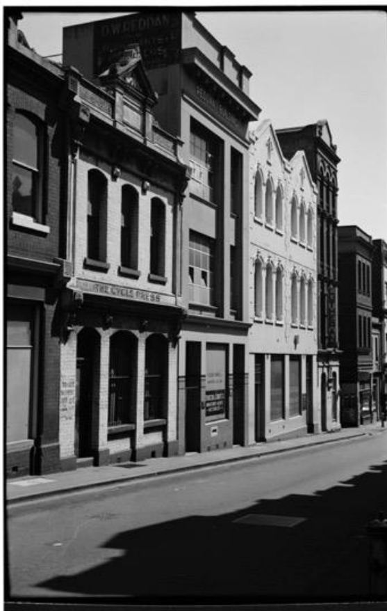
Figure 7. Little Lonsdale Street, 1968, showing numbers 281 (middle two-storey building) and 283-285 (to right of 281). (Source: Halla 1968, SLV)
