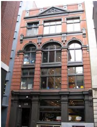
Figure 7. 179 Flinders Lane, built in 1911 (Source: CoMMaps)
