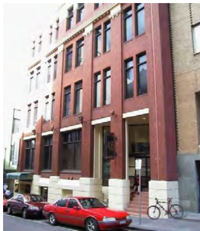
Figure 9. 401-405 Little Bourke Street, built in 1911.
