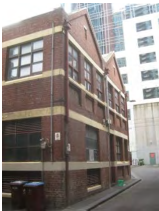
Figure 4. 1-3 Evans Lane, constructed in 1913.
