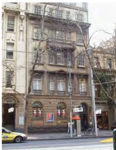
Figure 5. 10-12 Collins Street built in 1916-1925.
