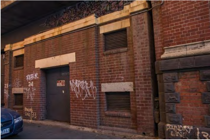
Figure 17. CitiPower substation (c1910s). (Source: Context 2019)
