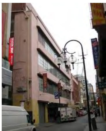
Figure 1. Rear of Target Centre at 222-244 Bourke Street, 209-225 Little Bourke Street, constructed 1937. (Source: CoMMaps)
