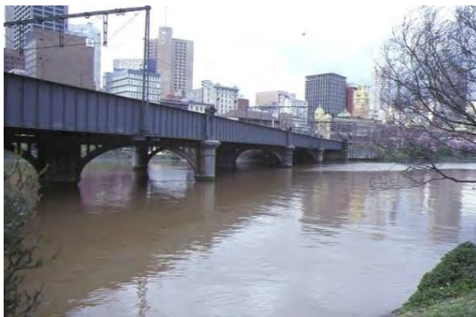
Figure 21. Sandridge Railway Line Bridge, 1886.
