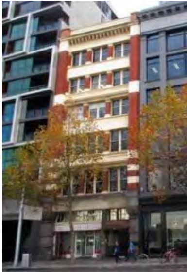
Figure 2. 100-102 Flinders Street constructed 1904. (Source: Context 2017)
