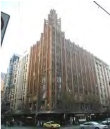
Figure 7. Manchester Unity Building, 220-226 Collins Street, constructed 1932.
