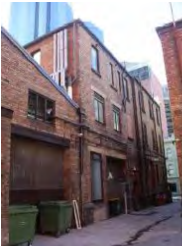
Figure 10. Rear of Union Bond Melbourne Storage Company Ltd constructed 1882.
