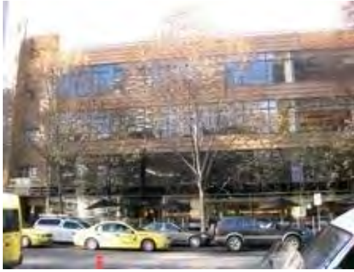
Figure 11. 546-566 Collins Street constructed in 1935.
