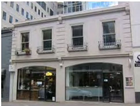
Figure 6. 470-472 Little Lonsdale Street constructed 1872. (Source Context 2017)
