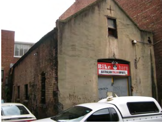
Figure 9. Rear of 361 Little Lonsdale constructed 1854.
