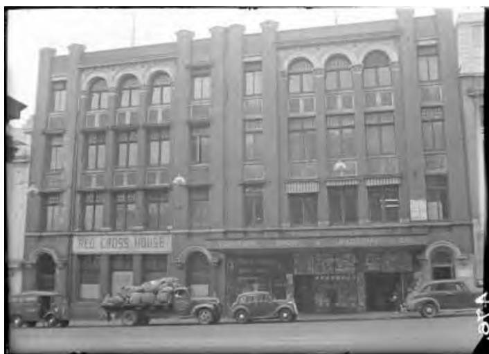
Figure 8. Melbourne Red Cross House, formerly Barnet Glass rubber company (Source: NAA 1917-1968)
