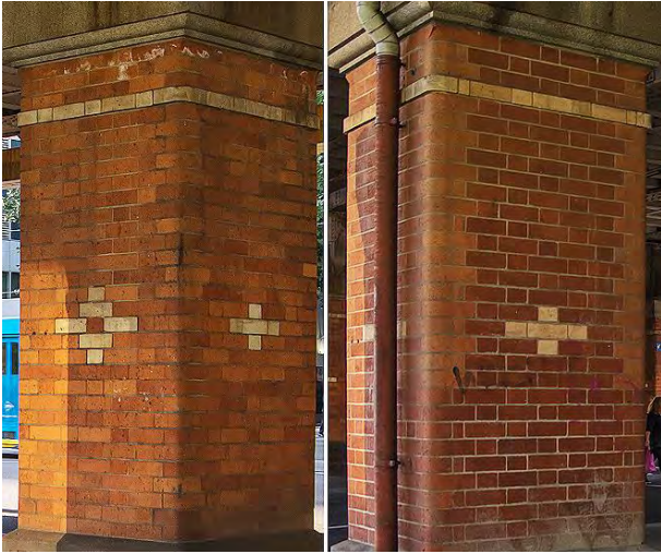
Figure 12. One of the earlier-constructed piers completed by 1891 (left-hand side) and one of the later piers completed by 1917 (right-hand side). Note more uneven and rough surface on the left-hand side example. (Source: Context 2019)
