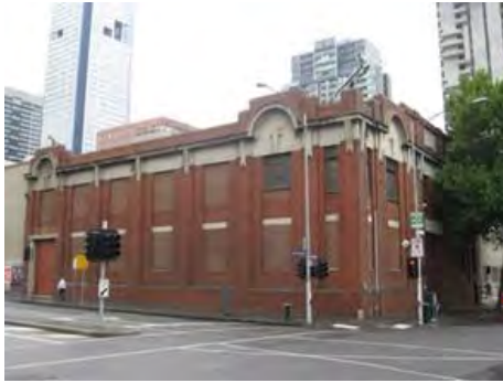
Figure 3. Substation at 651-669 Lonsdale Street constructed 1915.
