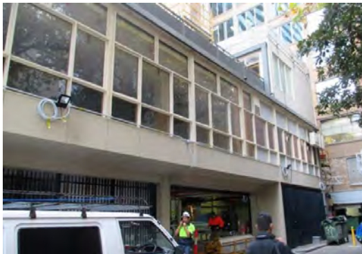
Figure 8. 2-18 Ridgway Place, built in 1958. (Source: Context, 2017)
