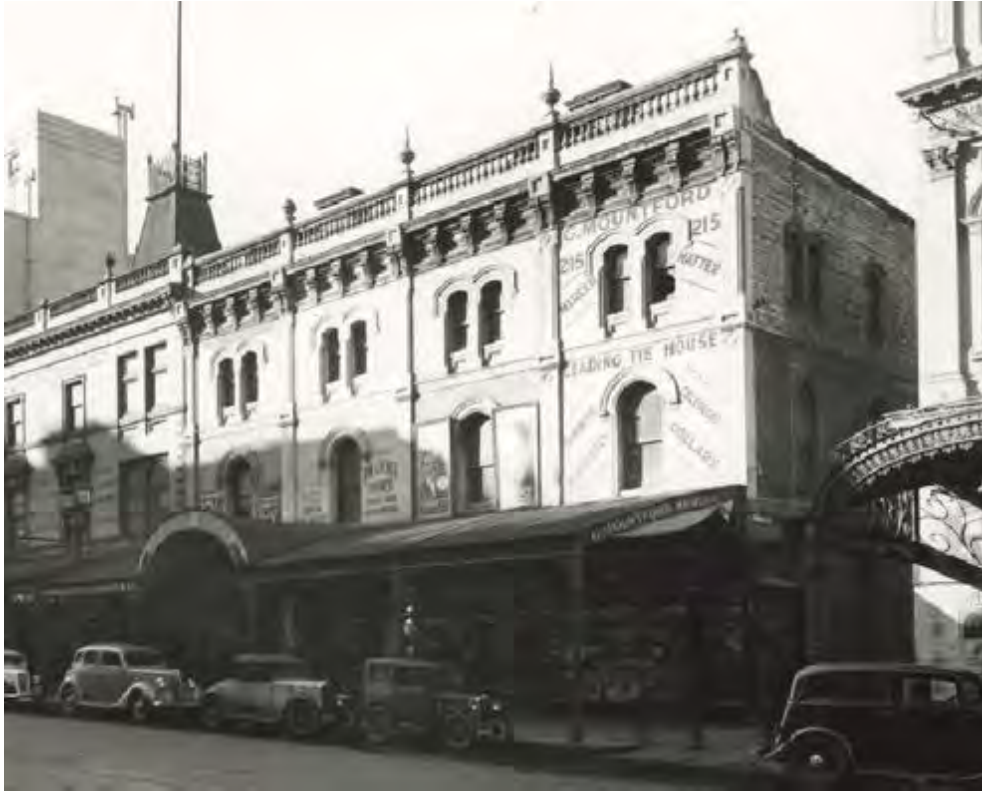
Figure 1. 209-215 Bourke Street in the 1940s. Wall painted signage for G Mountford junior's mercer shop is at 215 Bourke Street. (Source: Commercial Photographic Co c1940s, SLV)
