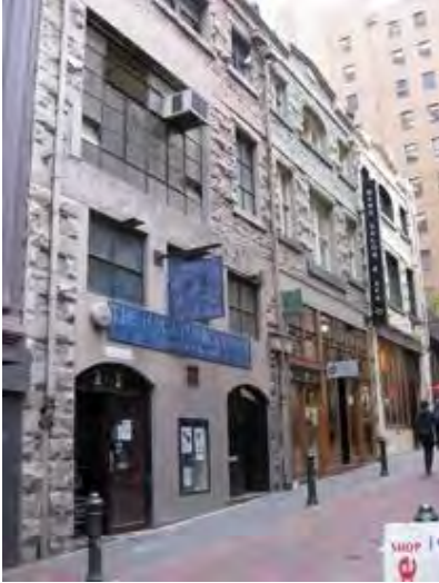
Figure 6. 15-19 McKillop Street constructed 1860.
