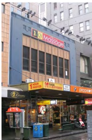
Figure 4. 7-9 Elizabeth Street, constructed in 1933.
