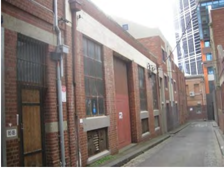
Figure 6. 12-14 Guildford Lane, constructed c 1920.
