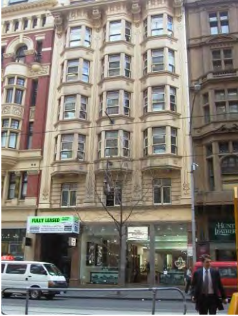
Figure 8. 294-296 Collins Street, built in 1914.
