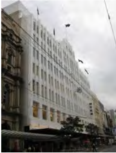
Figure 8. Myer Emporium, 314-316 Bourke Street constructed 1933.
