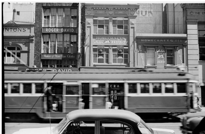
Figure 5. Showing the three-storey buildings at 207-209 Swanston Street occupied by Roger David and 211-213 Swanston Street occupied by Homecrafts c1950. (Source: Strizic c1950-c1980, SLV)
