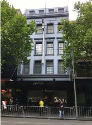
Figure 10. 152-156 Swanston Street originally built in 1888 and remodelled in 1936.
