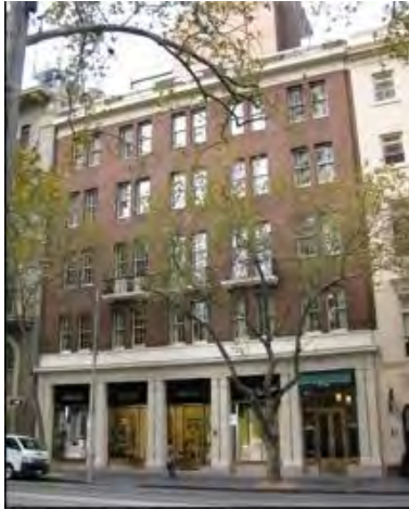
Figure 7. 81 Collins Street, Alexandra Club built 1934.
