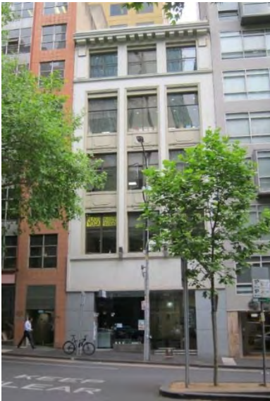
Figure 9. 410-412 Lonsdale Street, built in 1922. (Source: Context 2018)
