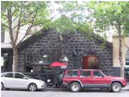
Figure 10. 585 Little Collins Street constructed 1865.
