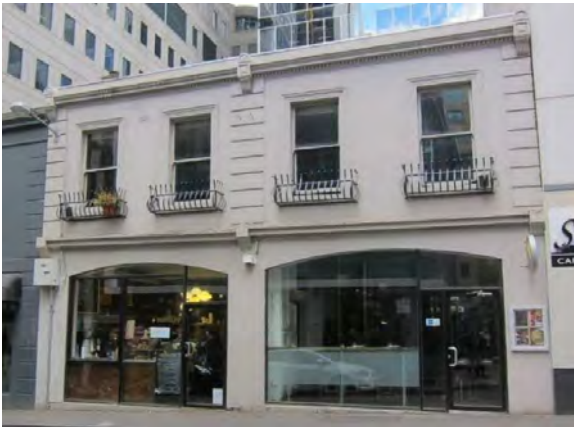
Figure 9. 470-472 Little Lonsdale Street, built in 1872. (Source Context 2017)
