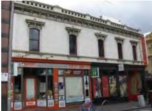
Figure 5. 189-195 Exhibition Street, constructed 1882.
