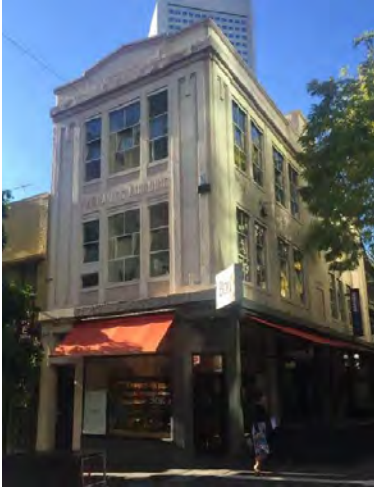
Figure 8. 386-392 Little Bourke Street, built in 1926.
