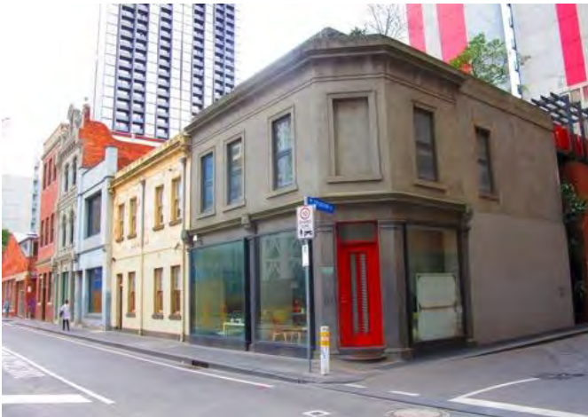
Figure 8. Little Lonsdale Street Precinct, from corner of Little Lonsdale and Exploration Lane. (Source: City of Melbourne 2018)
