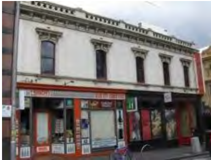
Figure 4. 189-195 Exhibition Street constructed in 1882. (Source: Butler 2011)
