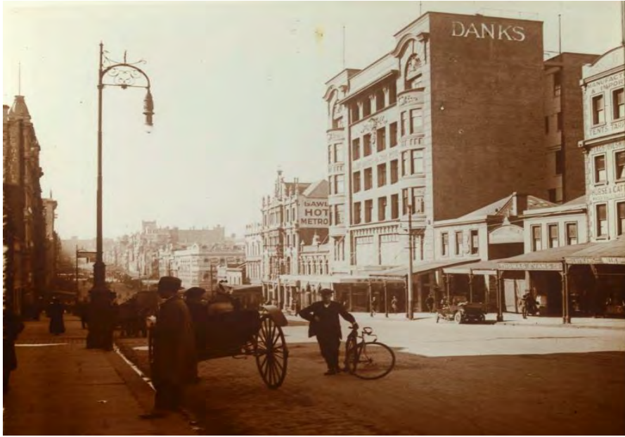
Figure 3. Showing the subject building c1920 after completion, with a large painted 'Danks' sign indicating the presence of the company. (Source: Harvey c1920, SLV)
