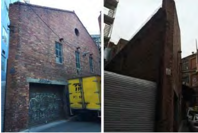
Figure 5. Rear of 369-71 Lonsdale Street constructed 1888.
