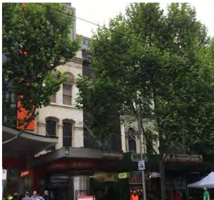
Figure 6. Row of four Victorian-era shops at 166-174 Swanston Street, constructed by 1888. (Source: Context 2017)
