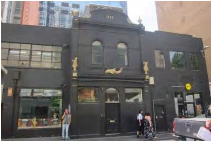
Figure 11. 100-106 Little Lonsdale Street, part of the extension to HO984. (Source: Context 2017)
