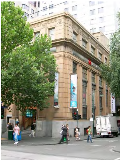
Figure 12. 119-225 Swanston Street, built in 1928 (Source: VHD)
