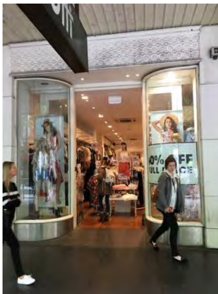
Figure 9. Shopfront at 161 Swanston Street retaining a recessed front entrance and curved glass with pressed metal panel above. (Source: Context 2017).
