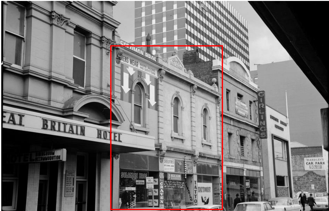
Figure 7. Photograph showing all three buildings that comprised Willis' Buildings in 1966. The buildings had been joined since 1948; the building on the left (with signage of long-time occupants, Solomon Bros) was demolished c1973. (Source: Halla 1966, SLV copyright )
