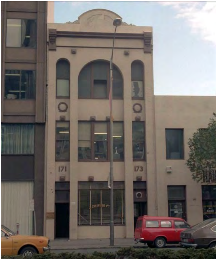
Figure 2. The subject site as it appeared in 1984. 'J Creffield' can be seen in gold lettering across the front window, indicating the firm's presence. (Source: Butler 1984 copyright )
