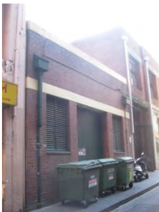
Figure 5. 28 Crossley Street, construction date unknown.
