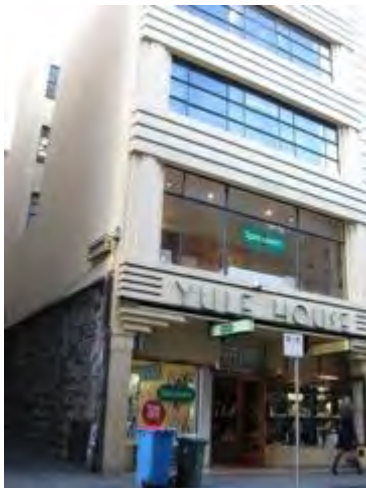
Figure 3. 309-311 Little Collins Street constructed in 1932. (Source: CoMMAps)
