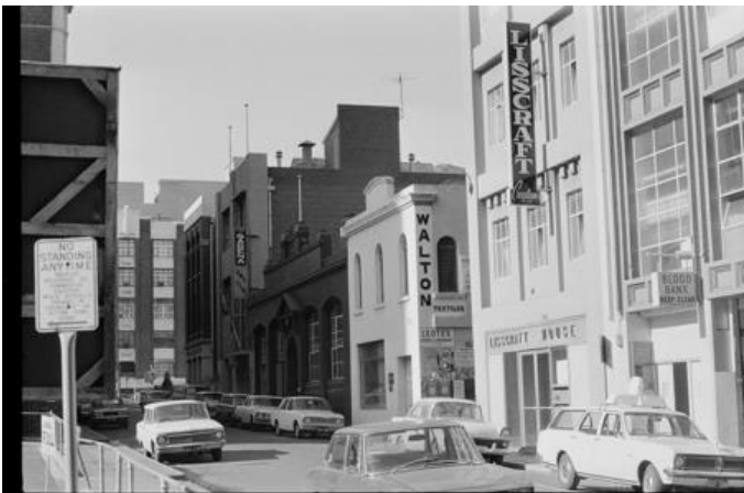
Figure 4. Flinders Lane between ACDC Lane (formerly Corporation Lane) and Exhibition Street showing Lisscraft House at 107-109, Walton Textiles at 103-105, and nos.87-95. (Source: Halla c1972, SLV H36133/484 copyright )
