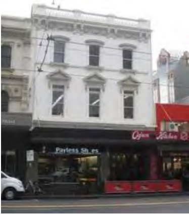
Figure 6. 136-140 Elizabeth Street, unknown built date.
