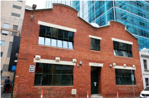
Figure 6. 27-29 Little Lonsdale Street, constructed in 1924.
