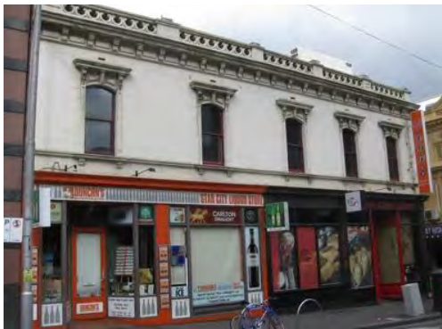
Figure 11. 189-195 Exhibition Street, built in 1882. (Source: Butler 2011)
