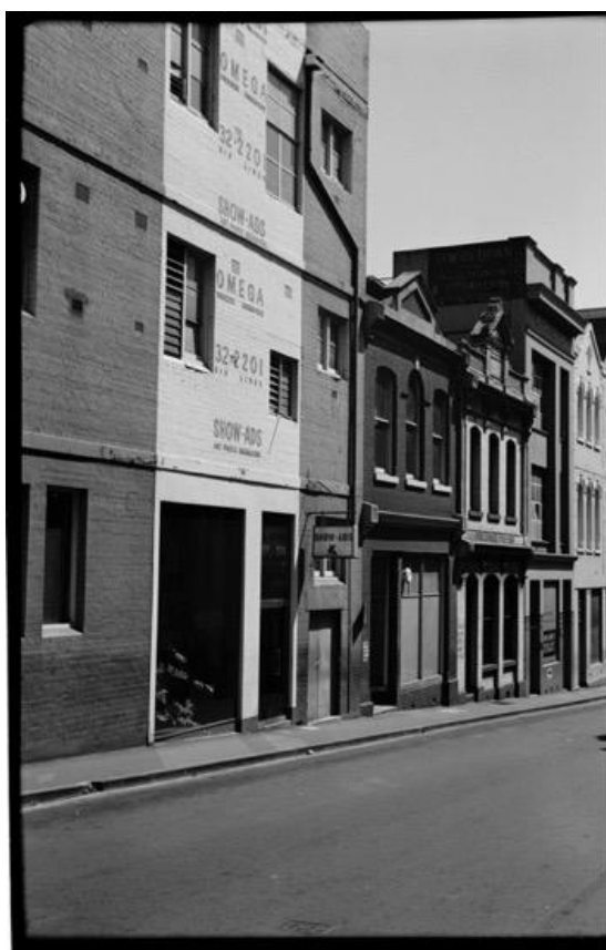
Figure 6. Little Lonsdale Street, 1968, showing numbers 277-279 (middle two-storey building) and 281 (to right of 277-279). (Source: Halla 1968, SLV)
