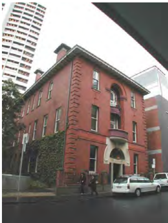
Figure 11. Milton House, 21-25 Flinders lane, 1901. (source: HERMES 130557)
