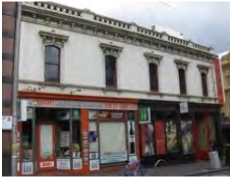
Figure 9. 189-195 Exhibition Street constructed 1882.
