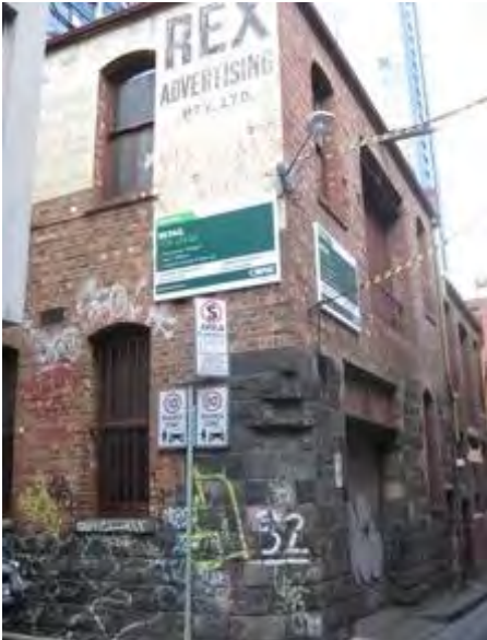
Figure 4. 32-34 Guildford Lane constructed 1908, with first floor added c1920.
