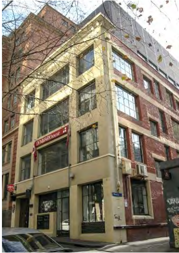
Figure 5. 428-432 Little Bourke Street, built in 1923.
