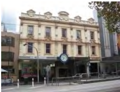
Figure 5. Bourke Mews, 32-38 Bourke Street constructed in 1892. (Source: Butler 2011)
