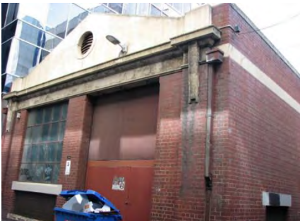
Figure 8. Substation, 10-14 Park Street constructed 1928. (Source: Context 2017)
