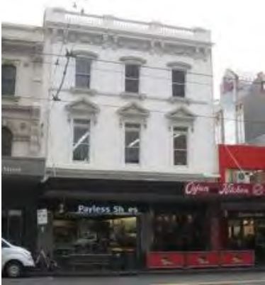
Figure 3. 136-140 Elizabeth Street, constructed in the mid-Victorian era.
