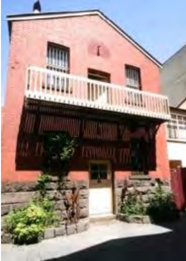
Figure 9. West wing of Currie & Richards showrooms & warehouses constructed c1900 (Source: Butler 2011:221).
