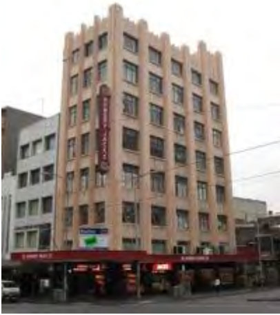
Figure 6. Norman's Corner Stores, 180-182 Bourke Street constructed 1932.
