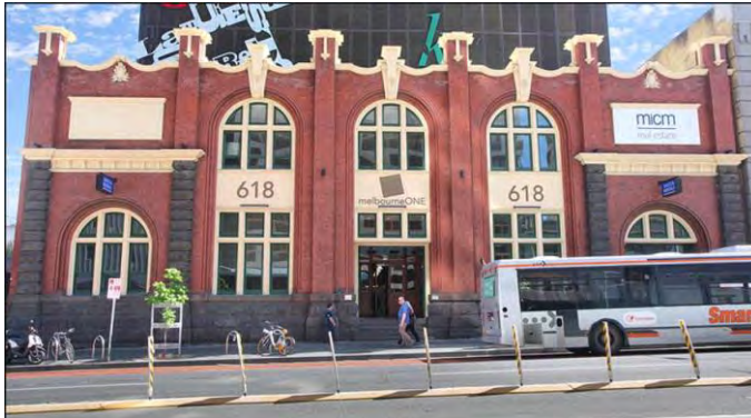
Figure 5. 612-620 Lonsdale Street, built in 1911. (Source: Gogle 2019)
