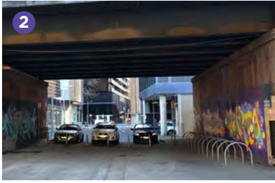
Image 9. The area beneath the viaducts is overshadowed, noisy and feels unsafe.
