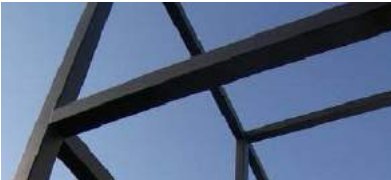
PRODUCT: ‘MONUMENT’ PAINTED STEEL FRAME WITH UNIVERSAL BEAMS AND SQUARE HOLLOW SECTION COLUMNS LOCATION: SUPPORTING CONTAINERS, PV’S AND OUTDOOR DINING CANOPIES
