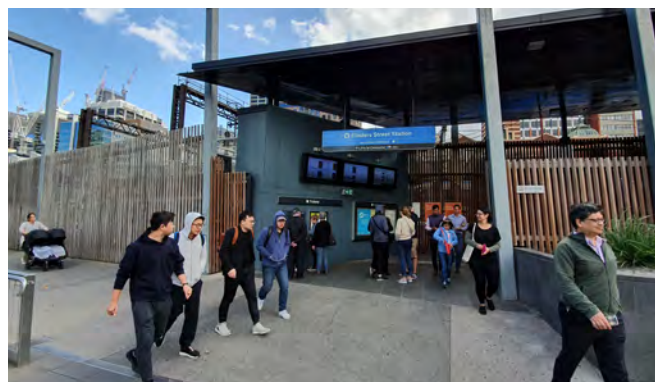
Image 27. Flinders Walk entry Flinders Street Station.
