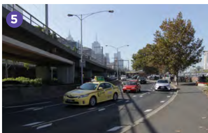
Image 13. Vehicular oriented infrastructure. A barrier to movement.
