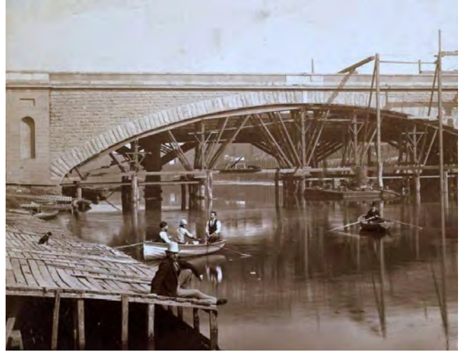
Image 52. First Princes Bridge construction 1884 (State Library of Victoria)
