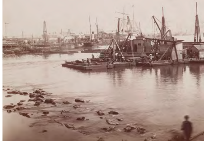
Image 48. Photo of the Falls removal works in 1883 (State Library of Victoria)
