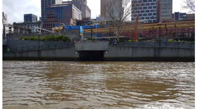
Image 59. Elizabeth Street main drain outlet underneath Flinders Walk
