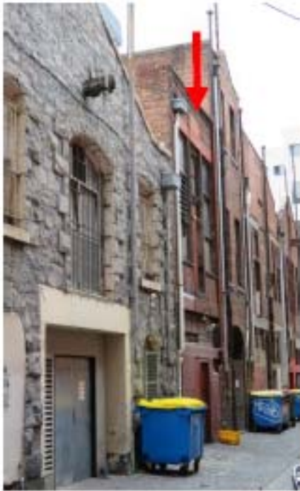
Heape Court with the brick rear elevation of 301 Elizabeth Street indicated
