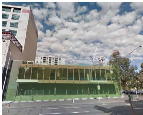
VIEW 3 Looking towards subject site from the edge of Flagstaff Gardens.
