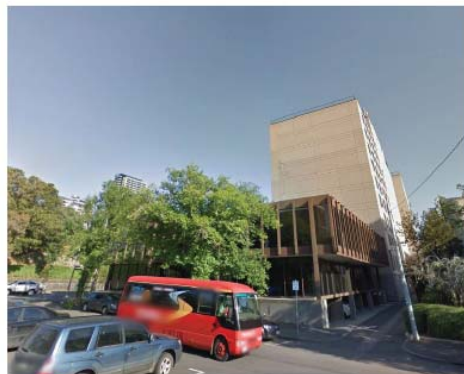
VIEW 5 Looking towards subject site along Batman St.
