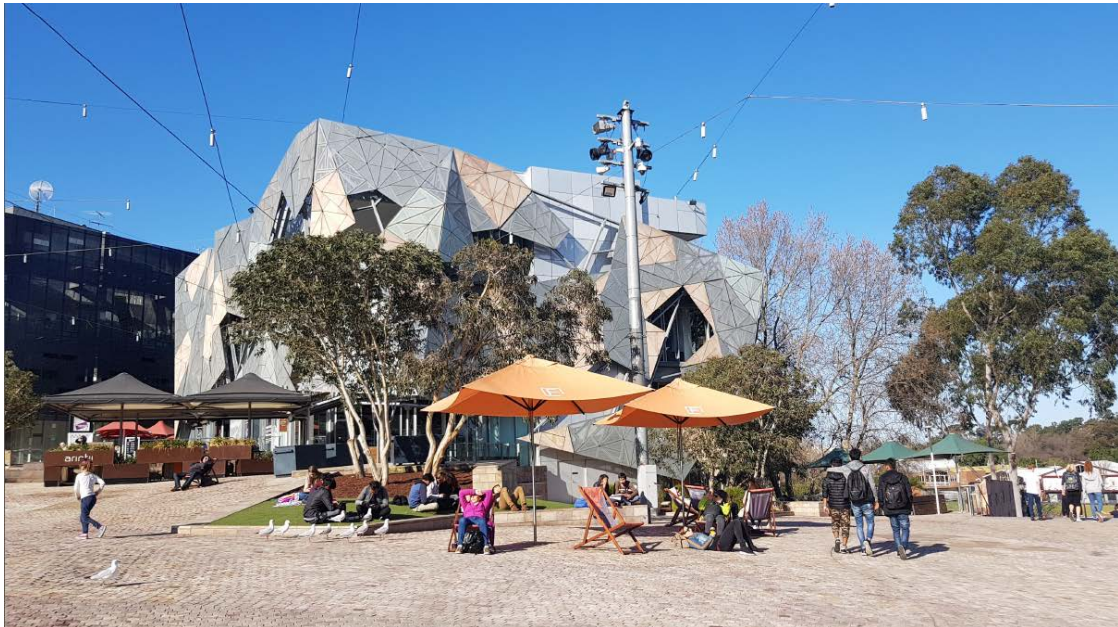
North-west elevations of Yarra building. Photo taken on 14 August 2018
