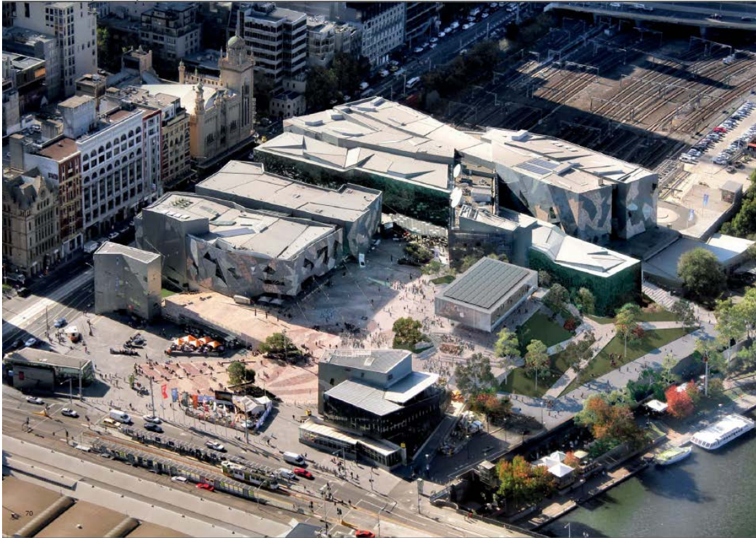
The proposal from the south west Source: Project Core – Federation Square by Foster + Partners
