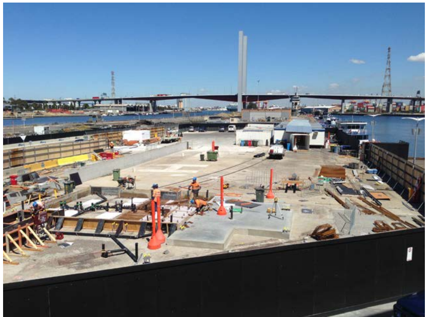
Photo: Construction on-site December 2014
