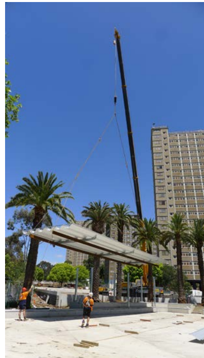
Figure 2 – Installation of basketball court shelter
