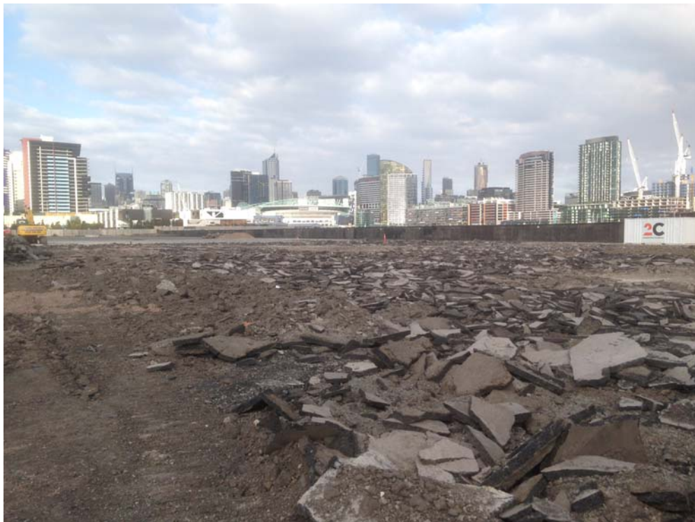
Demolition in progress – view east to Harbour Esplanade
