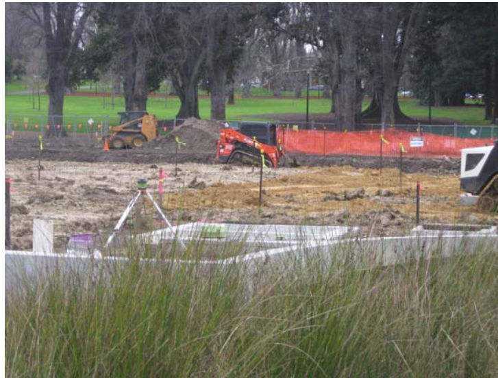
Figure 1: Landscaping Works being carried out by the contractor Delta.
