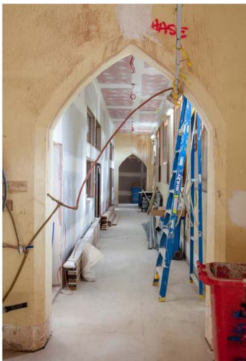
Corridor – Ground Floor
