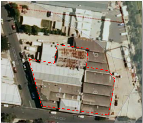
Site of 21-35 Barrett Street with red dash indicating contributory buildings on site including 43 Bruce Street) - rear wing on east has been demolished since this aerial view
