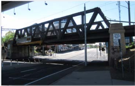
Bridge from west, showing trusses and rendered pylons.
