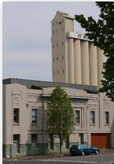
Figure 19 Building 5, silos with distinctive corrugated iron clad roofed wing on south
