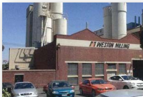
Figure 9 Building 3- Munster Terrace with earlier wall
