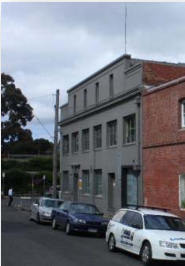
Figure 25 Building 11- Anderson Street elevations- Smith & Sons later Brockhoff biscuit factory and red brick TB Guest biscuit factory wings adjoining
