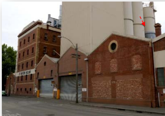
Figure 8 Building 3 -Laurens St, store ('50 Laurens St'), roof forms and chimney
