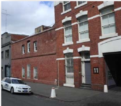
Figure 23 Building 9, 10- Anderson Street elevations, TB Guest biscuit factory wings
