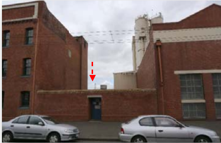
Figure 16 Building 3 - Victorian-era brick wall in Munster Terrace (arrowed) with new opening, Victorian-era, - rear of Building 3.
