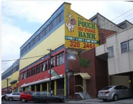
East end of complex, 1940 wing
