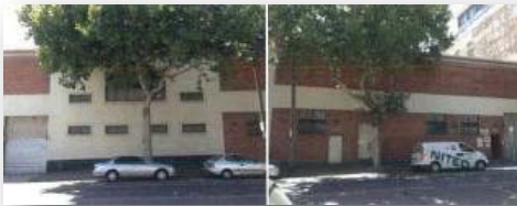
Figure 4 Laurens St Building 1
