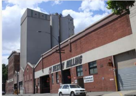
Brunton sections above- as 3 gabled stores, 5 level mill and another gabled store
