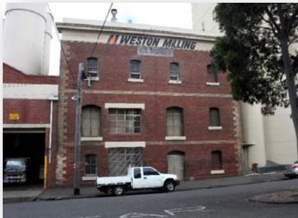
Figure 17 Building 4-Munster Terrace
