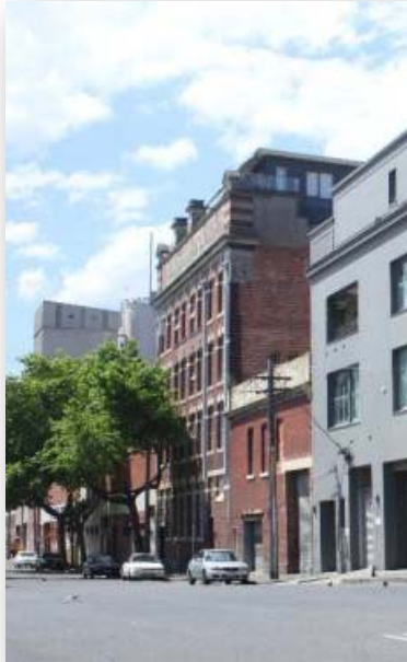
Figure 22 Building 9, 10, Laurens St
