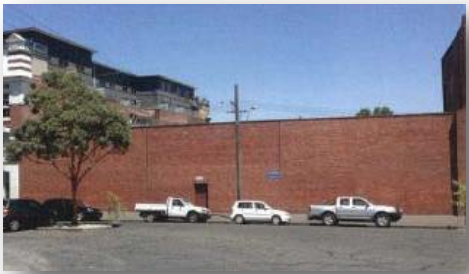
Figure 5 Anderson St, Building 1- recent wall, not contributory,
