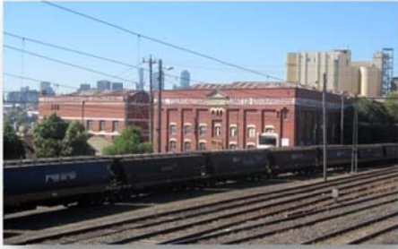
Stores 2, 1 from north
