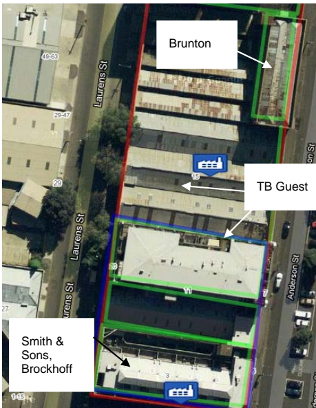
South end of precinct (red line), with key elements outlined in green, including parts of Brunton's Australian Roller Flour Mill and TB Guest biscuit factory centre while at south end is part TB Guest and former Brockhoff biscuit factories included
