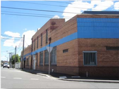
View of complex from south end, Richard Butler design extended up by Morsby.
