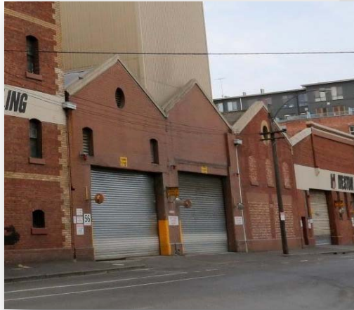
Figure 7 Building 3 -Laurens St Building 3 2013, publicly visible roofs
