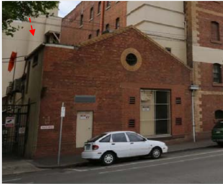
Building 7 (part Brunton's Australian Roller Flour Mills as gabled store to Laurens St)
