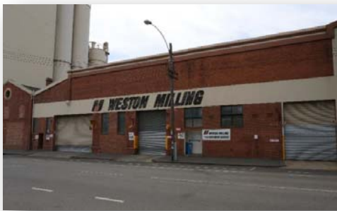
Building 8 (inter-war or later warehouse)
