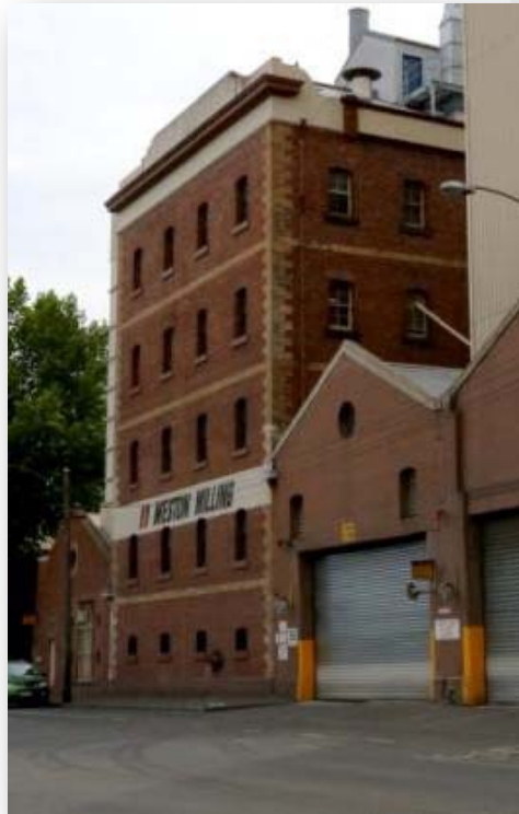
Figure 18 Building 4- Laurens St
