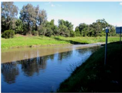
North section of Moonee Ponds Creek in overlay area, in naturalised form but with some stone pitchers visible at edge
