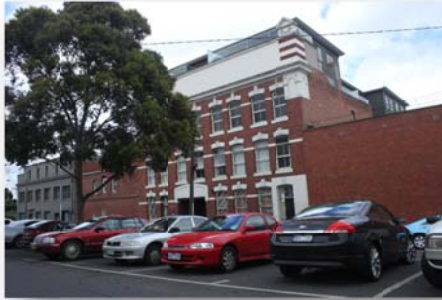
TB Guest biscuit factory, Anderson Street 2011, adjoining former Brockhoff building at the corner.
