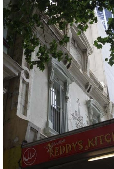
• Figure 119 380 Elizabeth Street upper level
