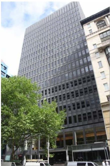
• Figure 79 430-442 Collins Street
