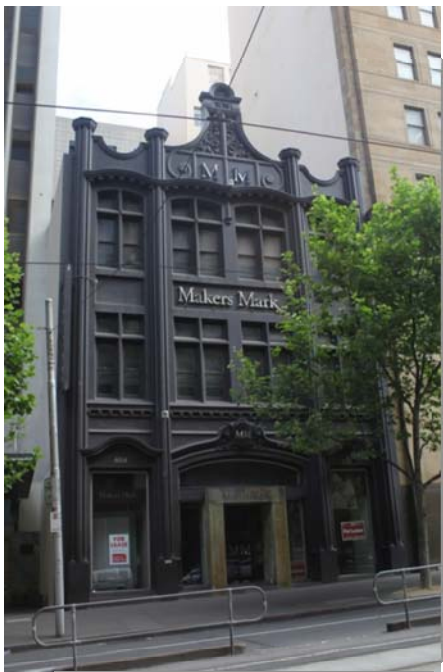
• Figure 86 464-466 Collins Street
