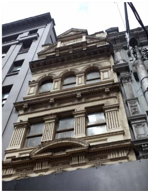
• Figure 98 21-23 Elizabeth Street upper level
