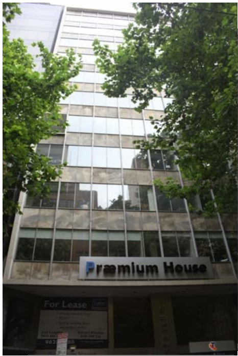
• Figure 71 404-406 Collins Street
