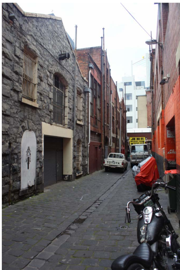
Figure 108 Rear façade and context
