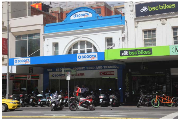
Figure 107 Elizabeth Street facade
