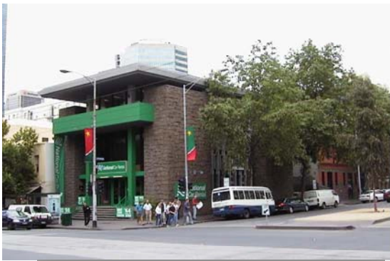
• Figure 131 453-457 Elizabeth Street prior to additions
