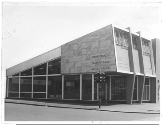
• Figure 135 463-465 Elizabeth Street as built (Commonwealth Banking Corporation archives)
