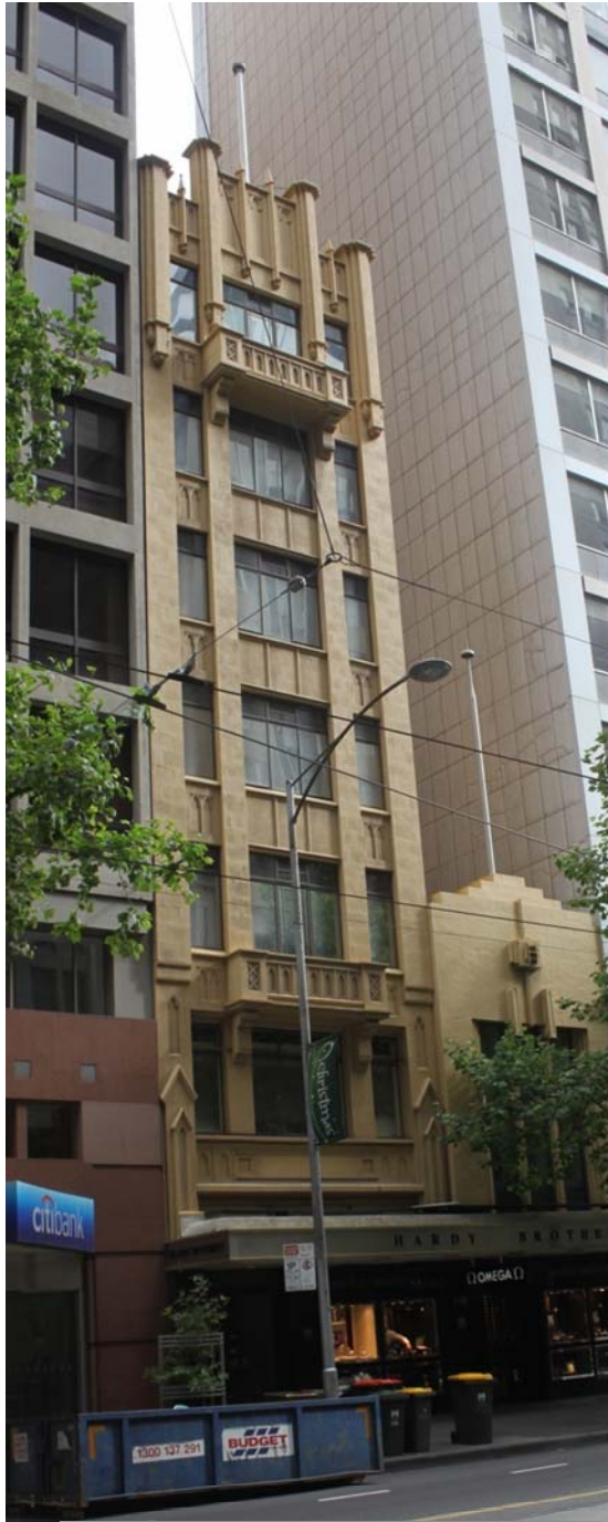
• Figure 68 342 Collins Street
