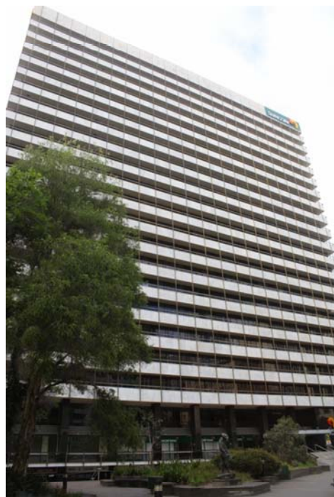
• Figure 82 435-455 Collins Street from north
