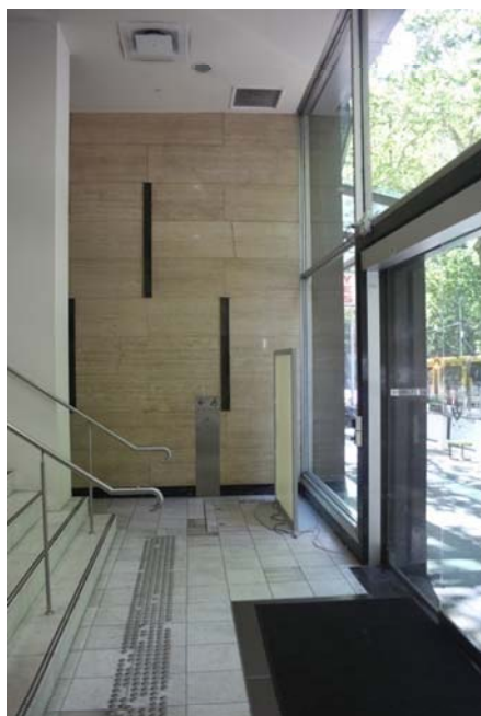
• Figure 62 Travertine, white and green marble in lobby, stainless steel handrails.
