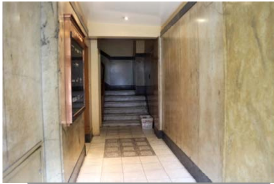
• Figure 113 Australian marble cladding in lobby.
