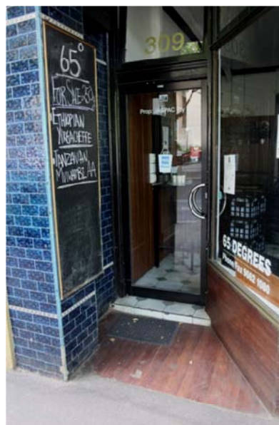
• Figure 160 309 Exhibition Street, part shopfront with tiles and entry recess (tiles covered/removed at plinth)
