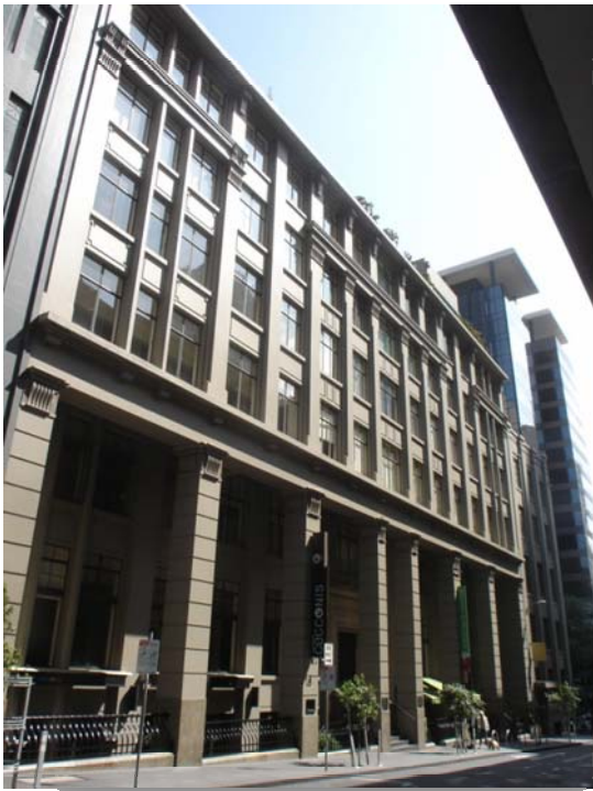
• Figure 162 61-73 Flinders Lane (NTA)
