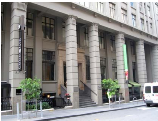
• Figure 163 61-73 Flinders Lane, ground level colonnade.
