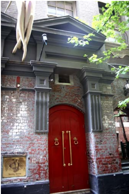
• Figure 94 9-13 Drewery Lane, entry
