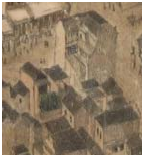
• Figure 25 DeGruchy & Leigh 1866: 3 storey building at corner (State Library of Victoria)
