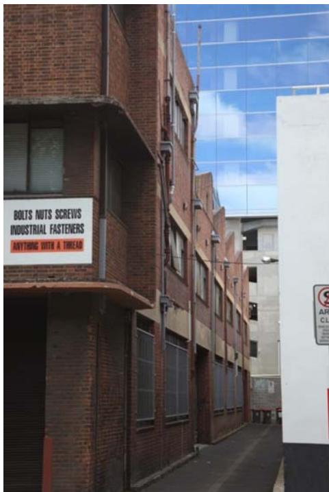
• Figure 10 sawtooth workshop wing behind
