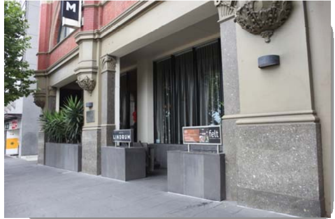
• Figure 180 26-30 Flinders Street, ground level
