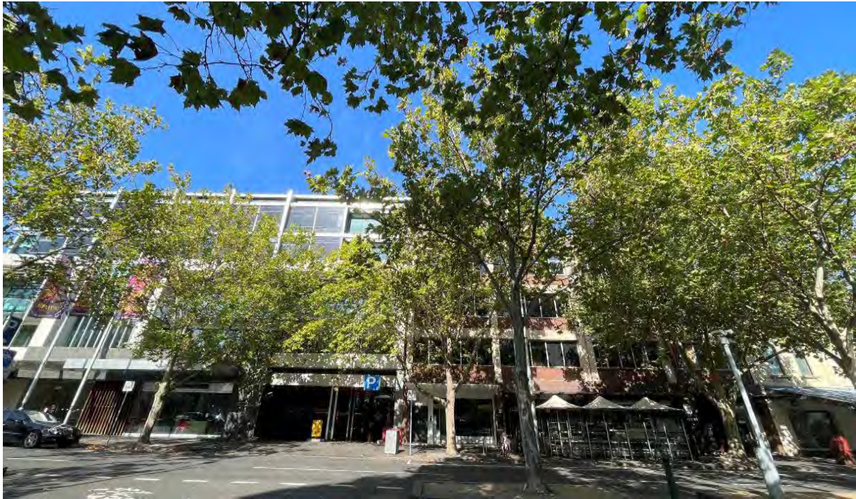
Figure 11 - Nos. 200 and 2004-218 Lygon Street to the north. Taken on 3 March 2023
