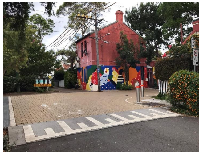
Raised intersection, Camden Street, Newtown, NSW
