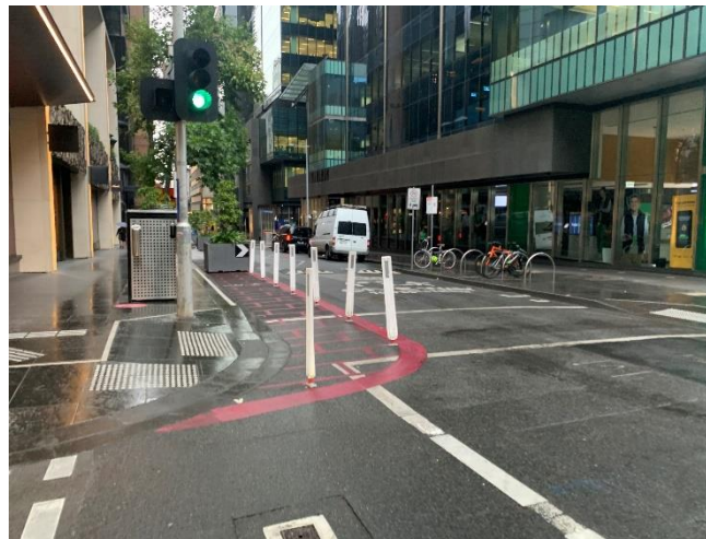
Footpath extension with paint and bollards, Little Collins Street
