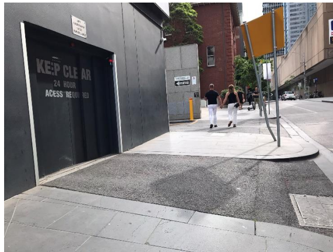
Example of tight kerb geometry (Flinders Lane, Exhibition to Spring)
