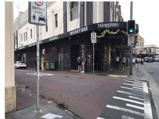
Raised threshold and surface colour and texture change at entry to shared zone, Newtown, NSW
