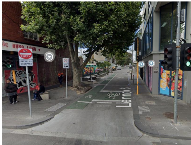
Signalised contraflow bike lane, Lennox Street, Richmond
