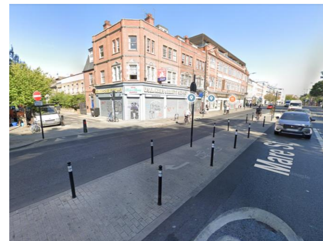
A median preventing some car movements from a one-way street, St Thomas's Square, London, UK
