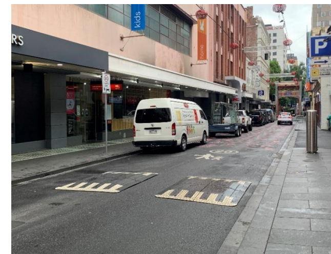
Example of mid-block treatment (Little Bourke Street, Swanston to Russell)
