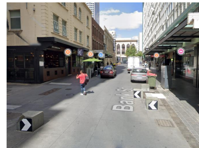
Chicanes to introduce horizontal deflection and create space for loading, Bank Street, Adelaide, SA
