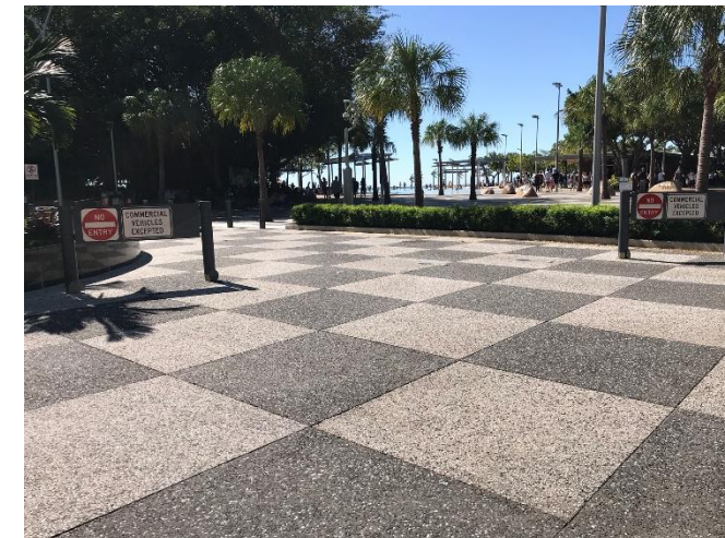
Raised intersection with contrasting surface colour and texture, Cairns, QLD
