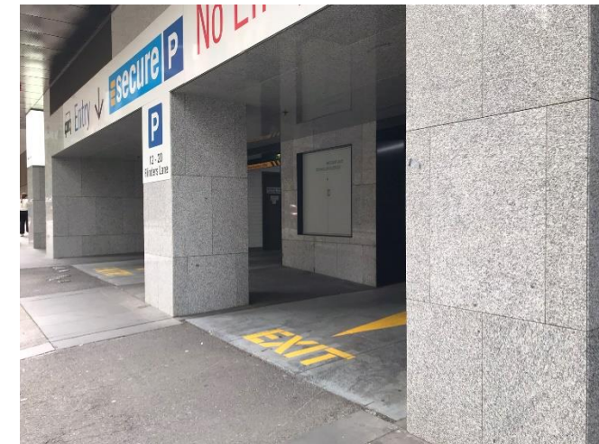
Example of column restricting visibility (Flinders Lane, Exhibition to Spring)
