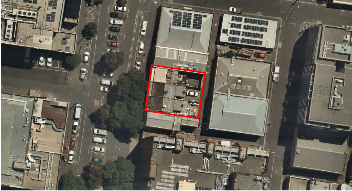
Figure 4 Recent aerial photograph of the subject site Source: Nearmap, January 2019
