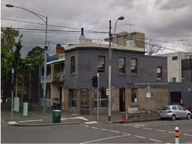
Figure 15 332 Cardigan Street, Carlton (HO1) Source: Google Streetview
