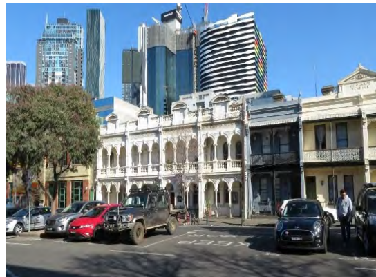
Figure 11 51-65 Cardigan Street, Carlton (HO27) Source: Lovell Chen
