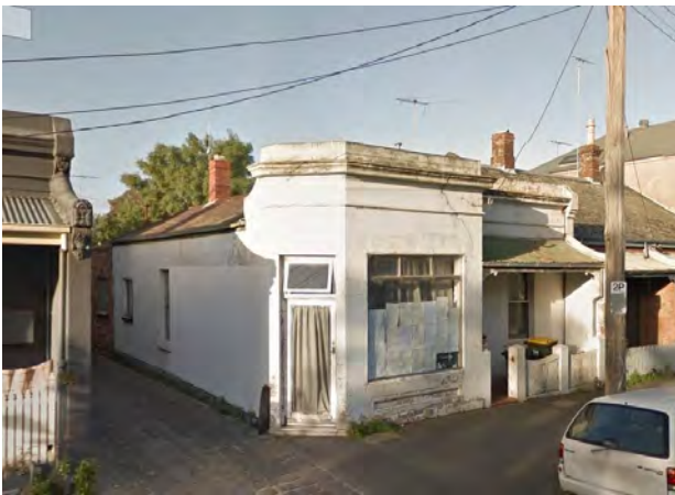
Figure 11 76 Palmerston Street, Carlton (HO1) Source: Google Streetview
