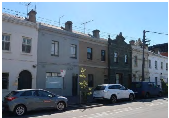
Figure 11 101-111 Cardigan Street, Carlton (H030) Source: Lovell Chen
