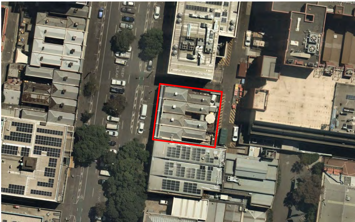
Figure 4 Recent aerial photograph of the subject site Source: Nearmap, January 2019
