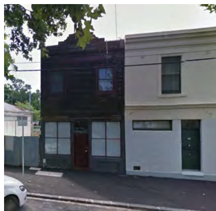
Figure 14 68 Barkly Street, Carlton (HO1) Source: Google Streetview
