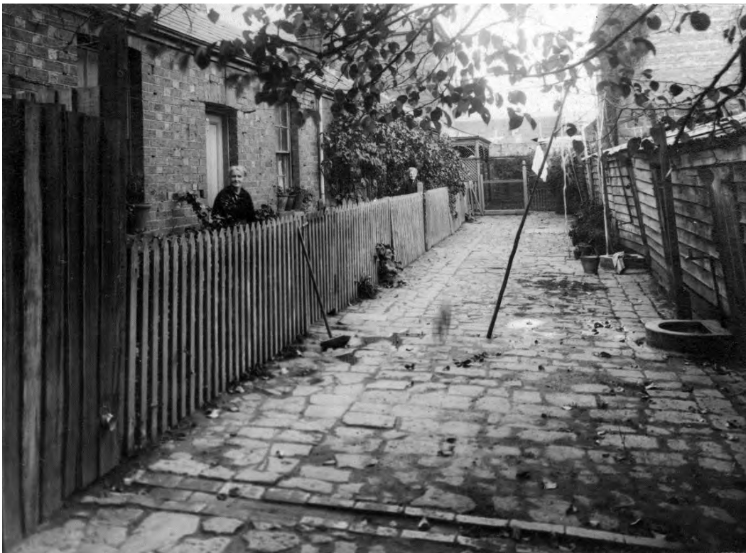
Figure 15 Residences fronting an unidentified laneway, 1934. Note access to water at right of lane and laundry drying at end of laneway Source: F Oswald Barnett collection, H2001.291/7, State Library of Victoria
