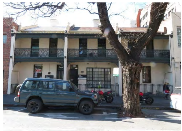
Figure 13 18-22 Cardigan Street, Carlton (HO35) Source: Lovell Chen
