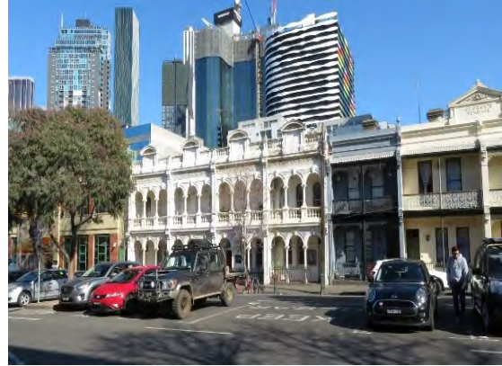
Figure 9 51-65 Cardigan Street, Carlton (HO27) Source: Lovell Chen
