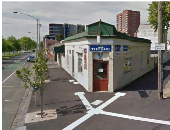
Figure 12 30 Canning Street, Carlton (HO1) Source: Google Streetview
