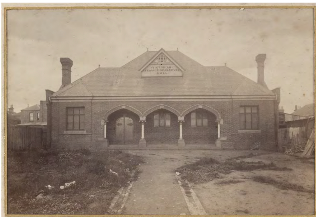
Figure 29 Female Operatives Hall at Trades Hall site, photographed in 1889, since demolished Source: In 'Presentation folder to Lord and Lady Loch from the Trades Hall Council, Melbourne', H40677/D, State Library of Victoria
