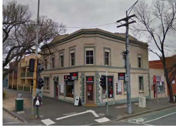
Figure 10 832 Swanston Street, Carlton (HO1) Source: Google Streetview
