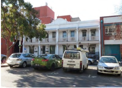
Figure 14 Mary's Terrace, 50-6 Cardigan Street, Carlton (HO36) Source: Lovell Chen
