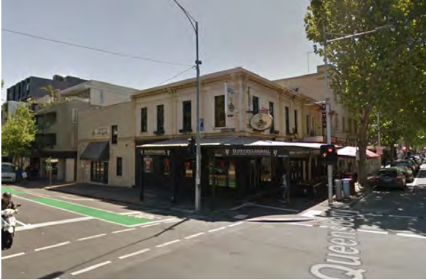
Figure 9 86-92 Queensberry Street, Carlton (HO1) Source: Google Streetview
