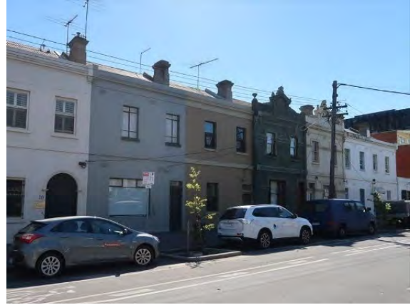
Figure 13 101-111 Cardigan Street, Carlton (HO30) Source: Lovell Chen
