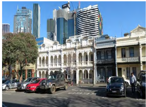
Figure 9 51-65 Cardigan Street, Carlton (HO27) Source: Lovell Chen
