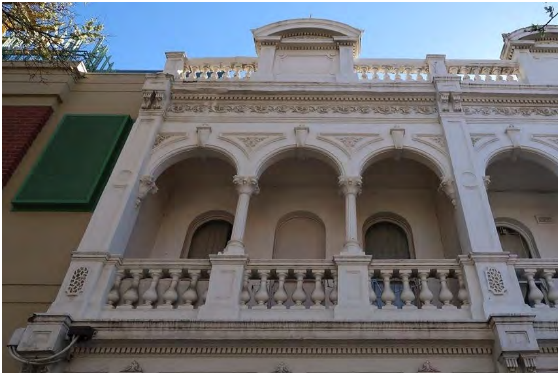
Figure 6 Upper façade, 51 Cardigan Street, Carlton
