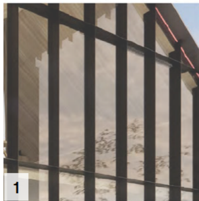
1 Steel window frame and shroud
