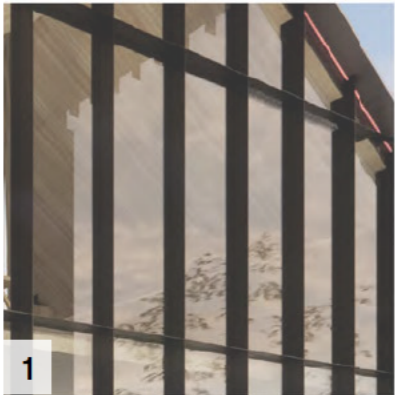
1 Steel window frame and shroud
