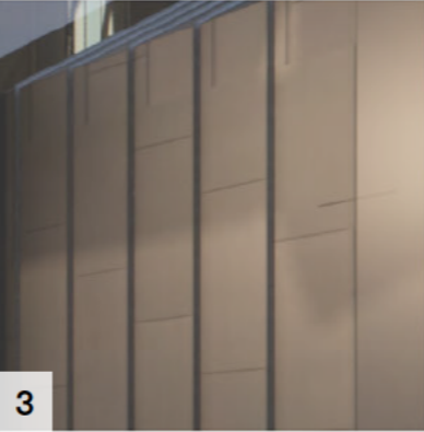
3 Standing seam roof and wall cladding
