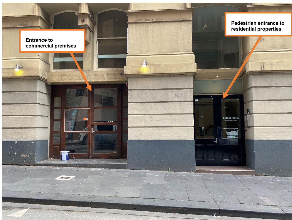
Figure 1: Subject site – entrance to commercial premises and residential properties of Fairfax House (Source: Officer's photo October 2022)
