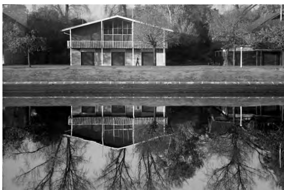
Figure 20. The newly constructed Melbourne Grammar School Boathouse c1950–59. (Source: Mark Strizic c1950-59. State Library Victoria: Mark Strizic collection of photographic negatives, Accession No: H2008.11/2155)
