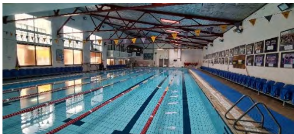
Figure 40. Swimming pool interior showing original 1935 skillion roof structure with exposed trusswork. (Source: GML Heritage 2021)
