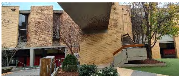
Figure 41. Eastern elevation, intersection of the central and southern section. (Source: GML Heritage 2021)
