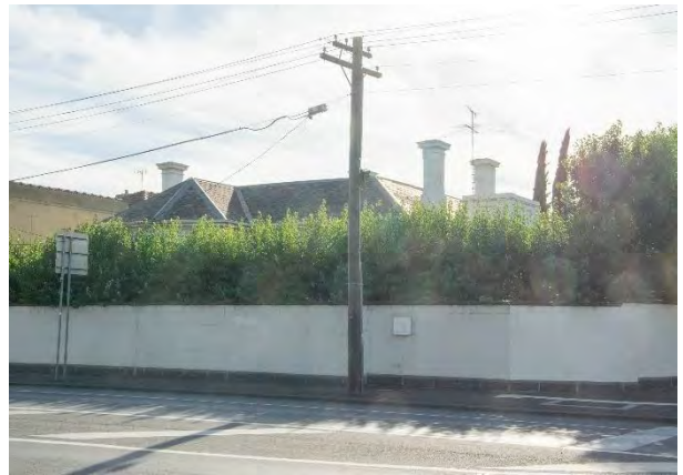
Figure 16. 1–13 Pasley Street North, occupying a corner allotment. (Source: GML Heritage 2021)
