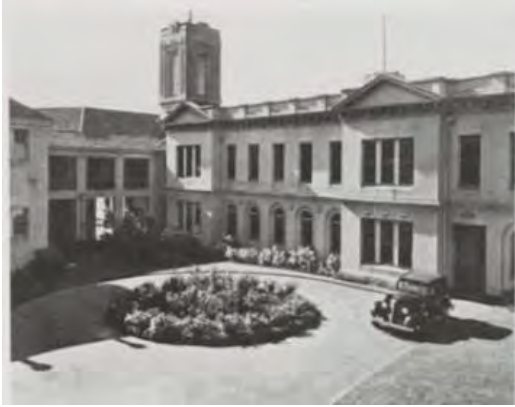
Figure 11. South-western corner of Nye Quadrangle, showing the remodelled West Wing and connecting science block, 1934. (Source: Collections of Wesley College Melbourne, via Lemon 2004:252)
