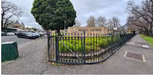
Figure 50. Cast iron picket fence on the corner of St Kilda Road and Moubray Street. (Source: GML Heritage 2021)
