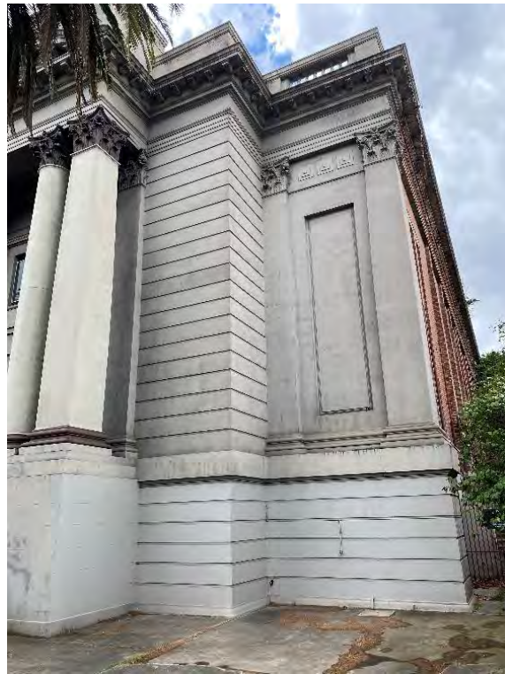
Figure 9. The eastern half of the front elevation, showing the stepped back form of the façade. The ruled render inner step back can be seen, along with the outer step back featuring pilasters. The prominent basement level is also visible underneath. (Source: GML Heritage 2021)
