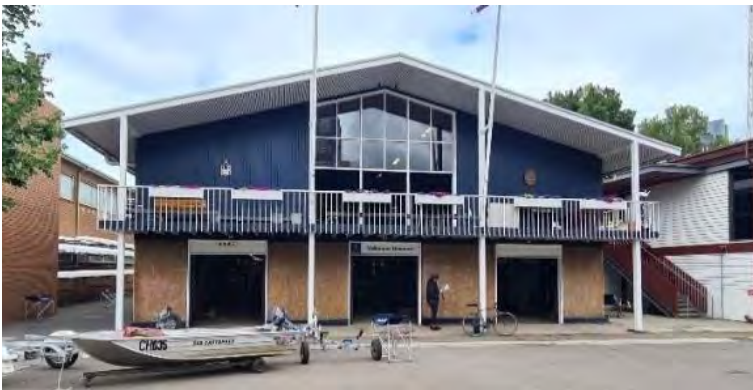
Figure 29. Principal façade of 4 Boathouse Drive, Melbourne. (Source: GML Heritage 2021)
