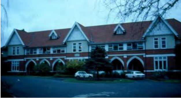
Figure 57. Scotch College, Hawthorn, 1917, established in 1851. (Source: National Trust Vic not dated via Hermes)
