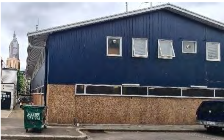
Figure 30. Principal façade of 4 Boathouse Drive, Melbourne. (Source: GML Heritage 2021)
