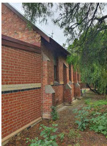
Figure 23. Northern side wall of the former hall, showing part of the extension (left, foreground). (Source: GML Heritage 2021)
