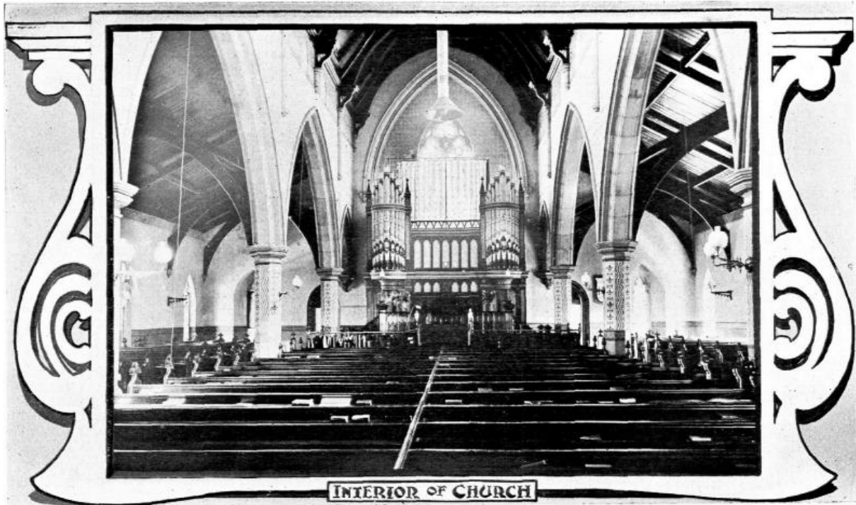
Figure 2. A 1905 view of the 1865 church interior. Note the space comprising central nave and two isles separated by piers and arches. (Source: South Yarra Presbyterian Church 1905:10)
