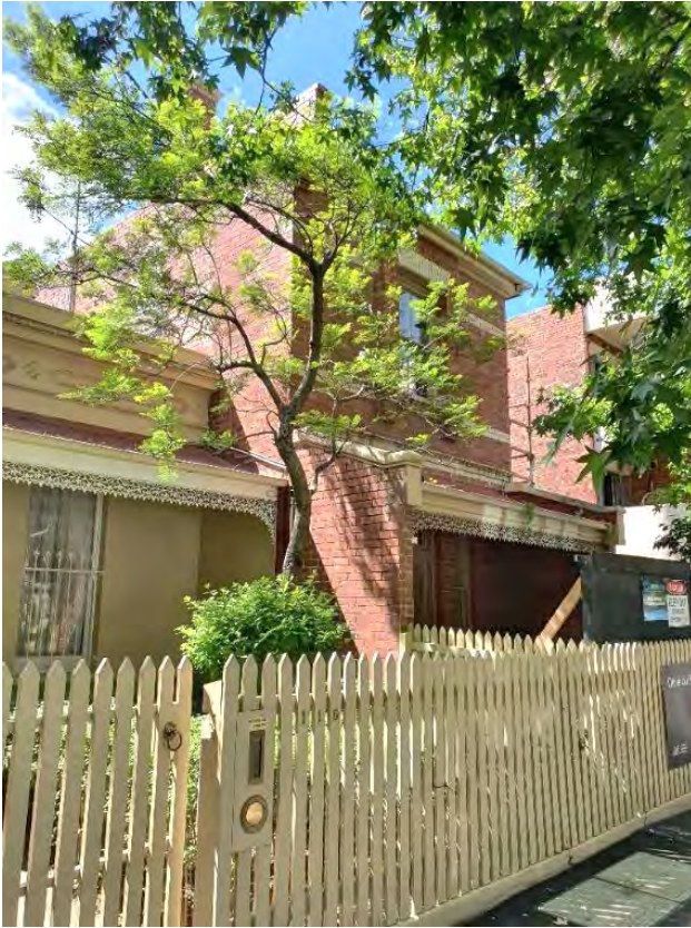
Figure 10. 114 Millswyn Street, with a narrow frontage to Millswyn Street. Note the decorative detailing including verandah with decorative ironwork, and the face red brickwork with cream brick detailing in the contrasting cornices, stringcourses and lintels. (Source: GML Heritage 2021)
