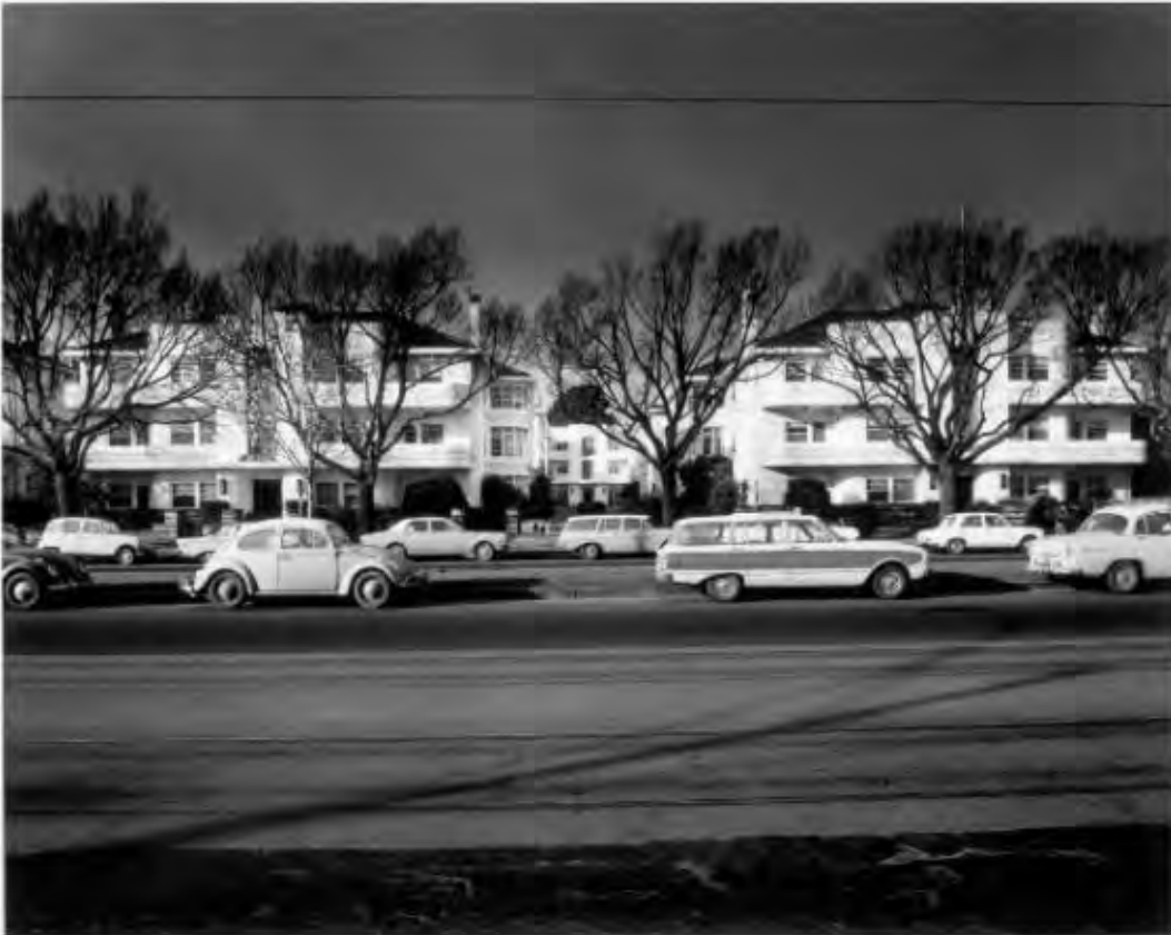
Figure 5. Photograph of the Kia Ora flats from St Kilda Road taken by Wolfgang Sievers in 1959. (Source: Wolfgang Sievers 1968, State Library Victoria: Wolfgang Sievers Collection, Accession No. H2001.40/215)
