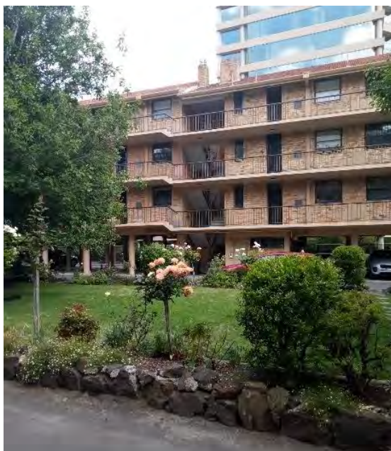
Figure 13. View across the internal courtyard and galleries and stairwell. (Source: GML Heritage 2021)
