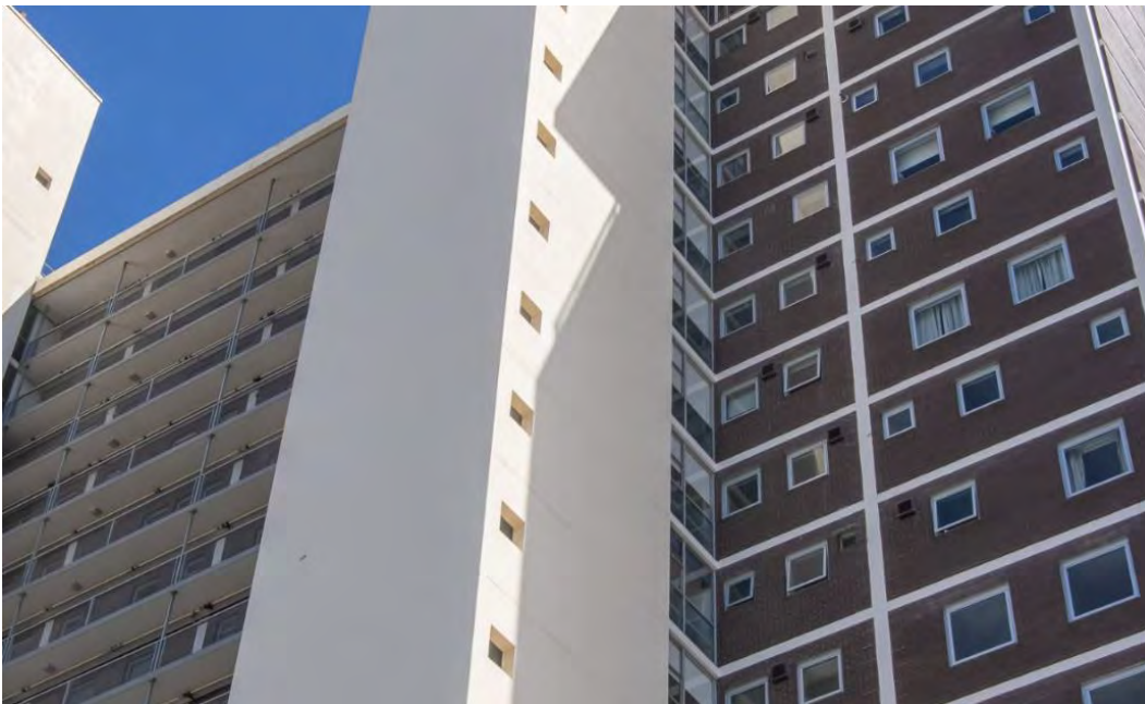
Figure 4. View of the rear elevation. Note the smaller openings on this elevation, openings on the fire staircase and the open service balconies between the service towers. (Source: GML Heritage 2021)
