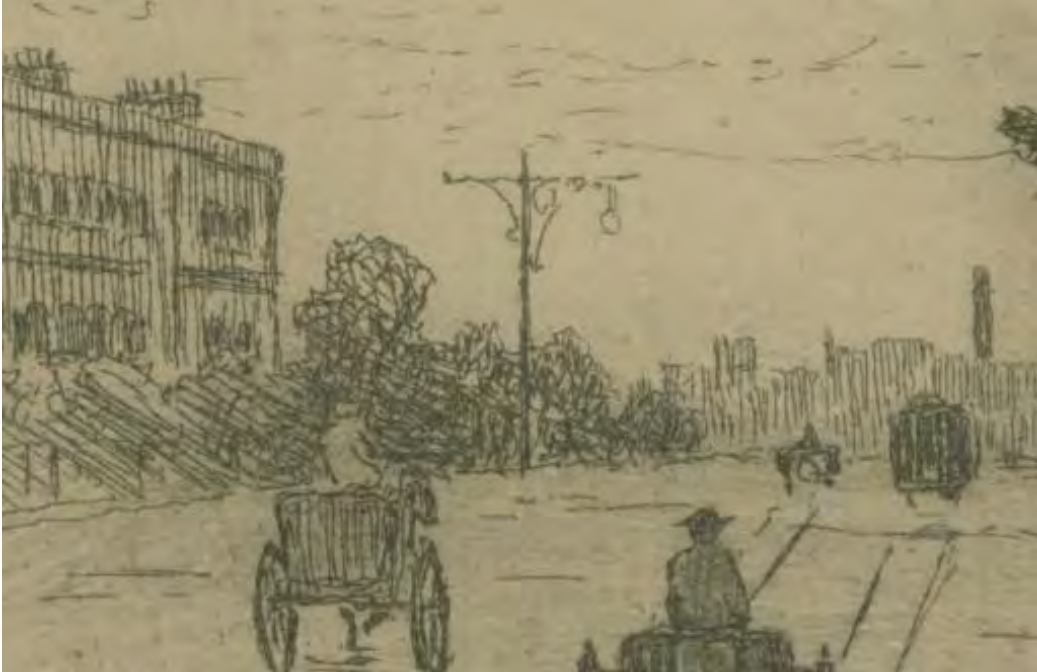
Figure 3.65 Detail from a sketch of Toorak Road West, showing a decorative gas lamp on the north side of the road, c.1890–1910. (Source: State Library Victoria)
