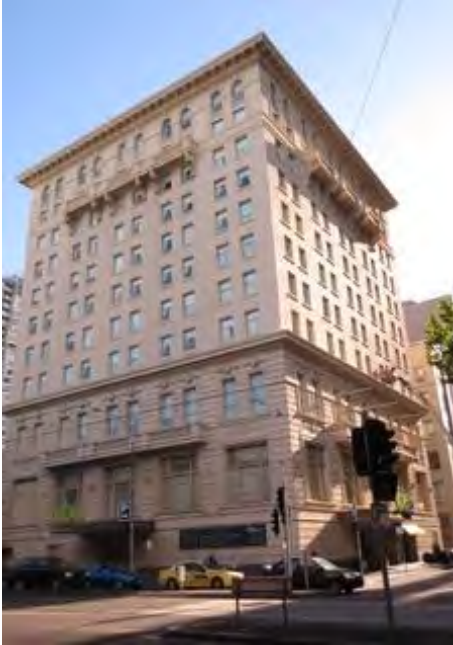
Figure 12. 630 Little Collins Street, Melbourne, built in 1928–29. (Source: CoMMaps)
