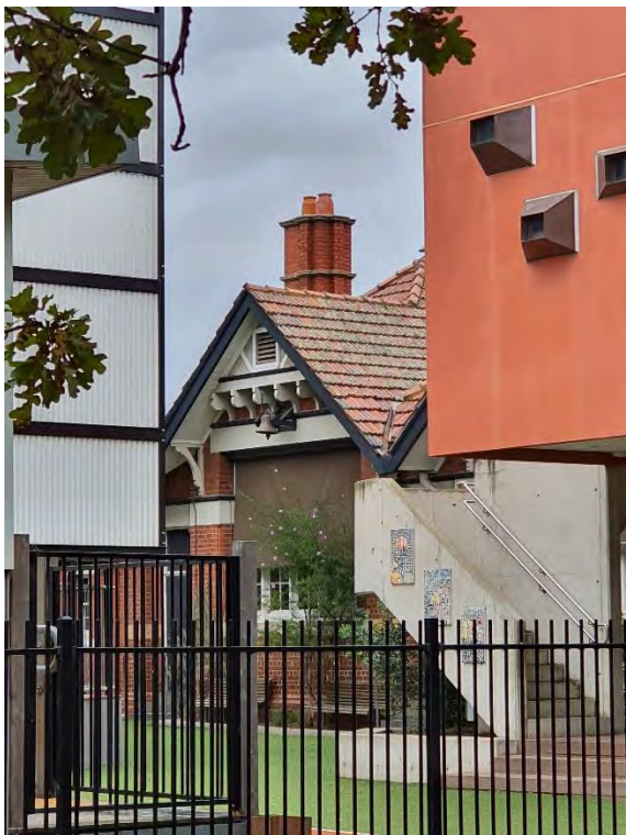
Figure 13. Rear of the infants' school building viewed from Fawkner Park showing the school bell. (Source: GML Heritage 2021)
