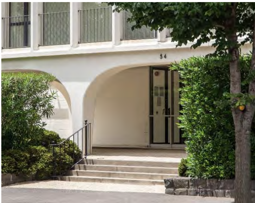
Figure 2. Concrete steps to the entry portico. Note the intact arched pilotis, modular frames and metal balustrading. (Source: GML Heritage 2021)
