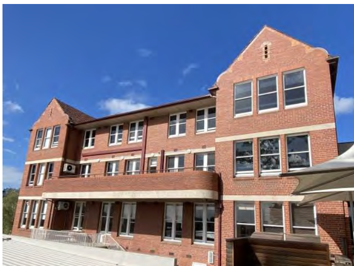
Figure 19. Principal elevation of Gilman Jones Hall, facing north. (Source: GML Heritage 2021)
