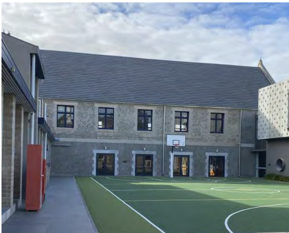
Figure 12. The western façade of the Memorial Hall building, showing how ground floor openings have been altered to accommodate doors. Modern school buildings can be seen either side of the hall in this image. (Source: GML Heritage 2021)
