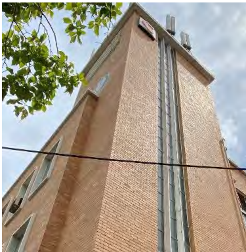
Figure 5. Detail showing the glazed detailing on the eastern elevation. (Source: GML Heritage 2021)
