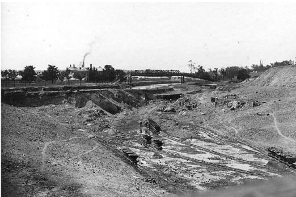
Figure 3.12 Work on the realignment of the Yarra River 1898. (Source: University of Melbourne Archives; copyright restrictions may apply)
