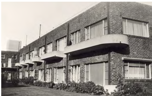
Figure 26. 98 Nicholson Street, Fitzroy, viewed from Hanover Street, built in 1935–36. (Source: Hermes)
