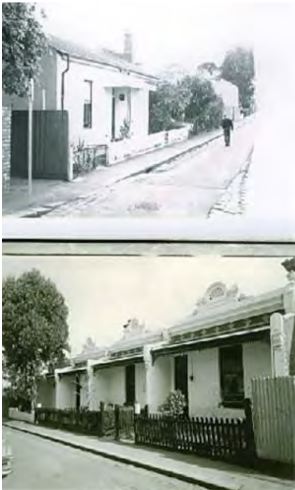
Figure 3.39 and 3.40 Workers' cottages in the Review area. (Source: Victorian Heritage Database)
