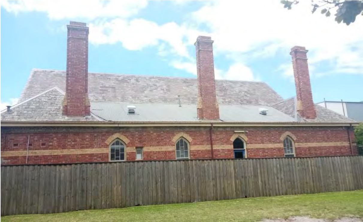
Figure 10. View of the 1884 Sunday school building from Fawkes Park (Figure 7: Number 4). Note the original elements including the chimneys and pointed arched openings. (Source: GML Heritage 2021)
