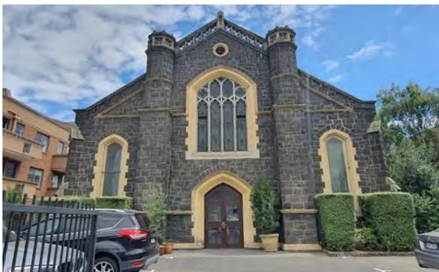
Figure 5. The primary (east) elevation of the former Wesleyan Church at 431–439 Punt Road. Note the use of side pointed arches and the intact Perpendicular Gothic style tracery with stained glass by Ferguson and Urie. (Source: GML Heritage 2021)
