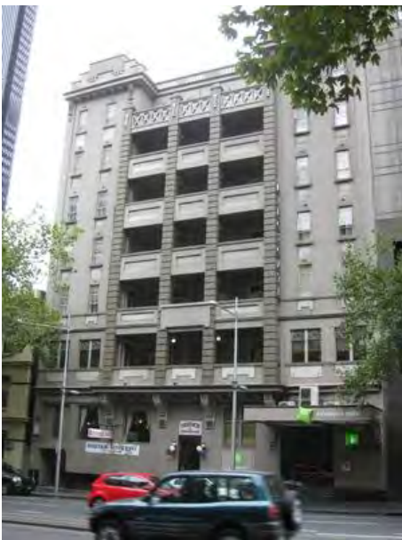
Figure 13. 131–135 King Street, Melbourne, built in 1926. (Source: CoMMap)
