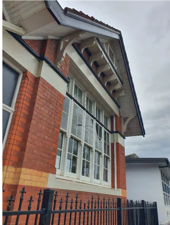
Figure 12. Eastern projecting gable of the infants' school and window detail showing timber brackets and set of five double-hung timber-framed sash windows with transom windows. (Source: GML Heritage 2021)
