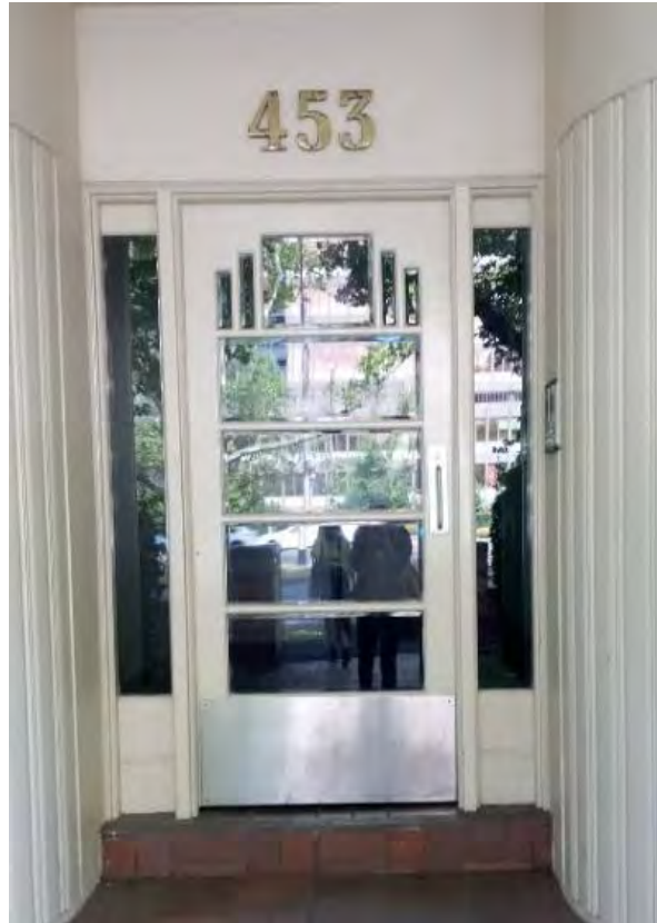
Figure 19. Decorative Moderne motif within the door. (Source: GML Heritage 2021)
