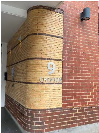
Figure 10. The formal entry of the 1934 portion fronting Commercial Road, finished with brown and red bricks with decorative cream and brown roman bricks. (Source: GML Heritage 2021)
