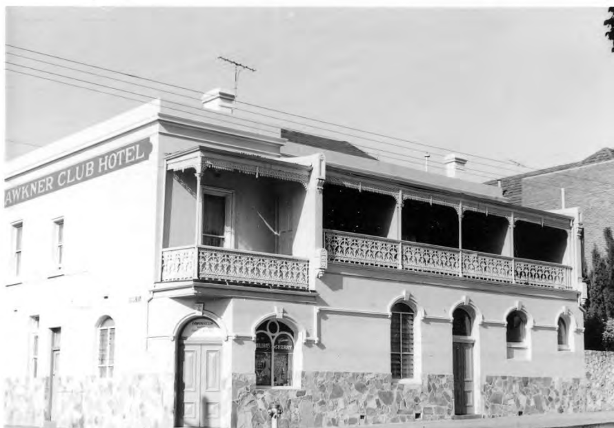
Figure 5. Fawkner Club Hotel, photographed by John T Collins in 1965. The stone cladding at ground level was later removed. Note that there are only four window openings and one door opening on the southern elevation. The door shown in the east end of the principal façade has been altered to form a window. (Source: John T Collins Collection, State Library Victoria, Accession No. H98.251/941)
