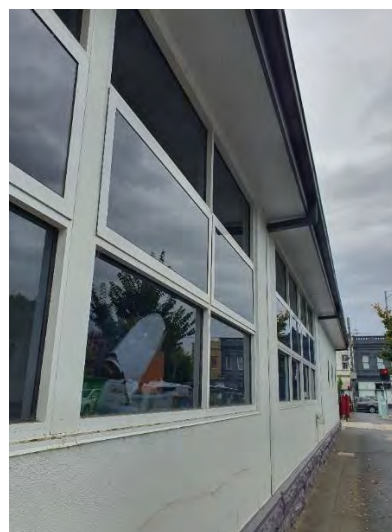
Figure 16. Aluminium-framed windows abutting Pasley Street North. (Source: GML Heritage 2021)
