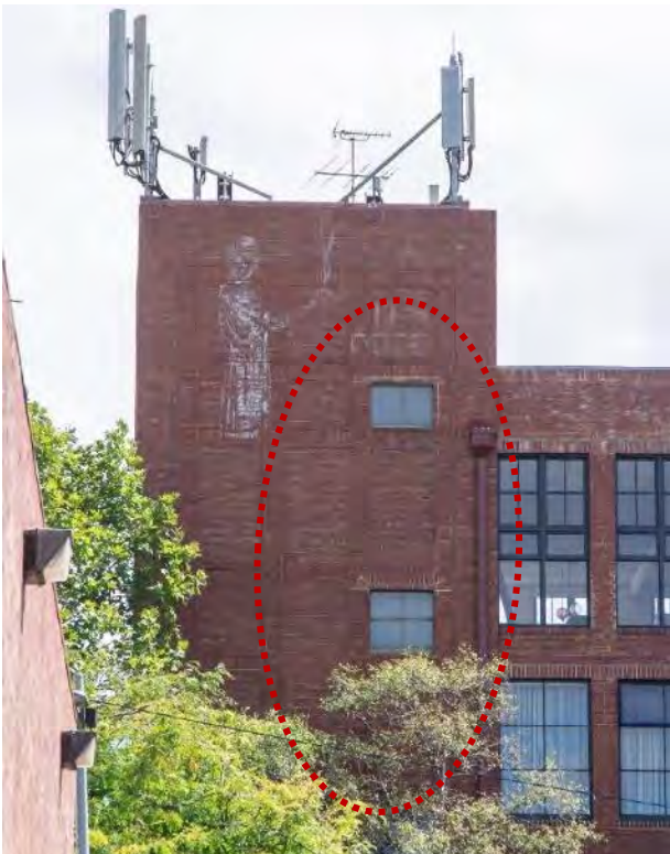
Figure 16. Stairwell on the west elevation of the 1922 former storage building with decorative brick detailing and remnant mural. The openings on the stairwell shown in dashed lines are original. (Source: GML Heritage 2021)
