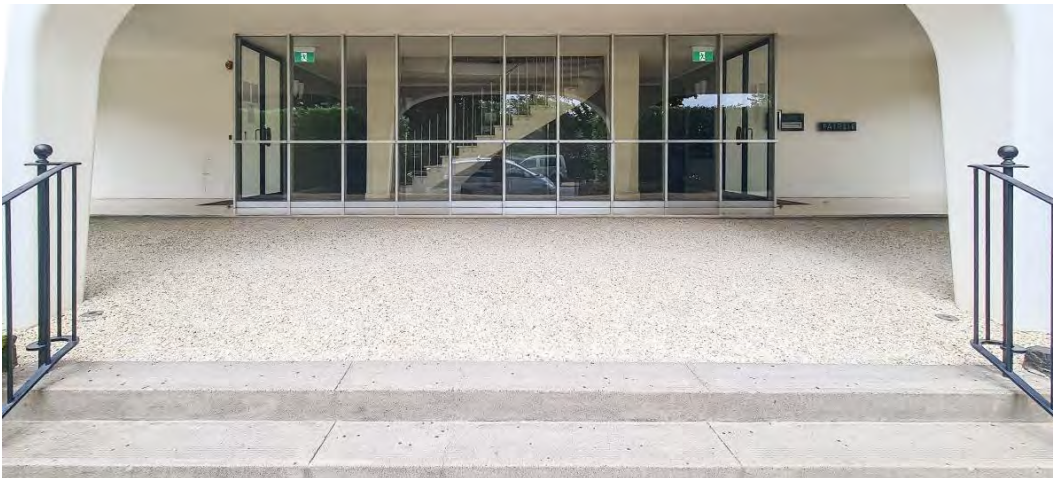
Figure 4. View of the portico and lobby enclosed by the fully glazed walls. The entrances are provided on both sides. (Source: GML Heritage 2021)
