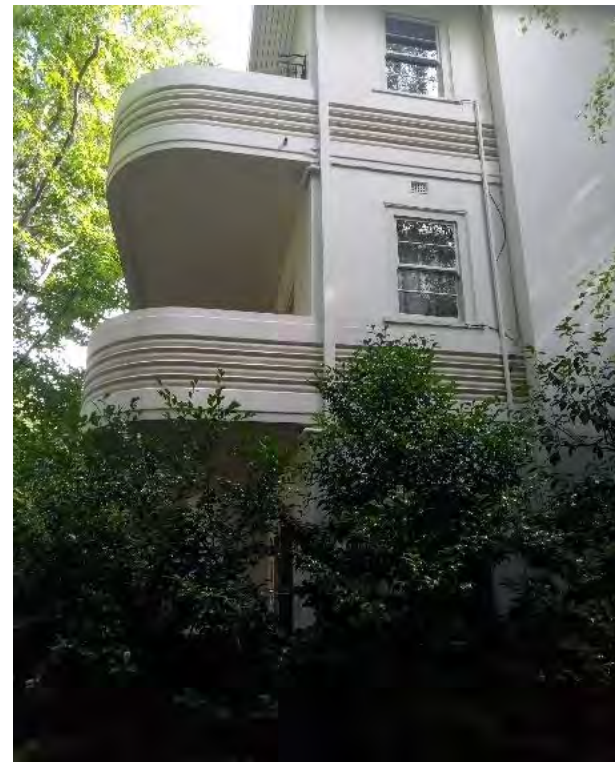
Figure 12. Curved balconies on the second and third floors with string course moulding matching the columns of the portico. (Source: GML Heritage 2021)
