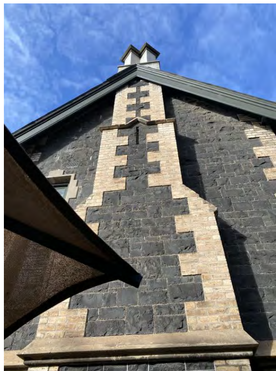
Figure 8. The chimney stack with quoining on the northern elevation of the vicarage. (Source: GML Heritage 2021)
