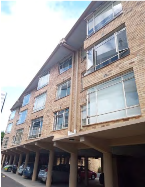
Figure 9. Windows along the serrated southern sides. (Source: GML Heritage 2021)
