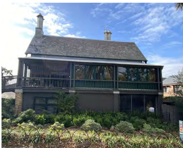
Figure 6. The principal (western) elevation of the vicarage with verandah. (Source: GML Heritage 2021)
