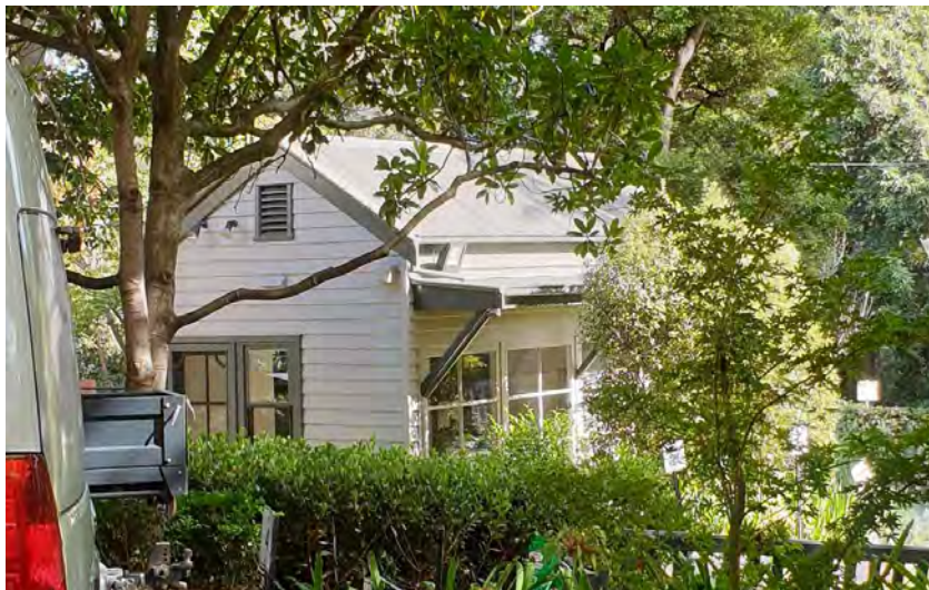
Figure 20. Former nursery. (Source: GML Heritage 2021)
