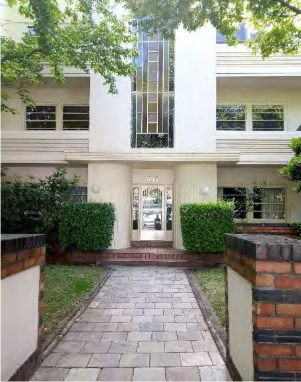
Figure 9. Entrance to number 453 from outside the St Kilda Road fence. (Source: GML Heritage 2021)
