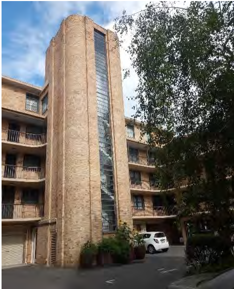
Figure 14. Stairwell at the western end extending above the main building and housing a lift. (Source: GML Heritage 2021)
