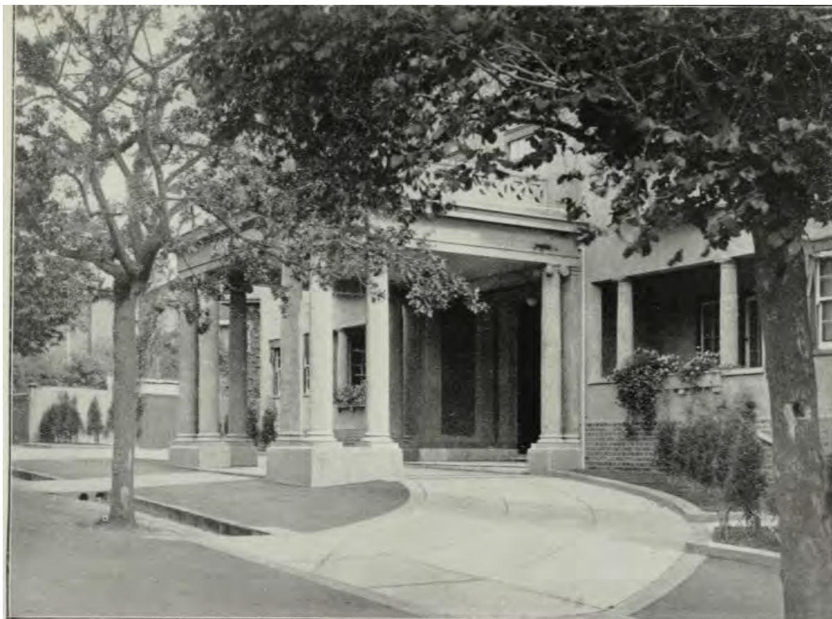
The porte cochère of Amesbury House, South Yarra. Square-set, spacious, dignified, its massive, yet graceful, proportions are consistent with the architectural character of the house itself. The triple groups of columns support a balcony enclosed by a decorative railing.
