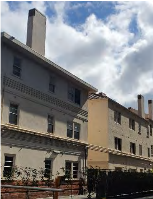
Figure 20. Southern side of the building showing the back of the building painted cream without render. (Source: GML Heritage 2021)
