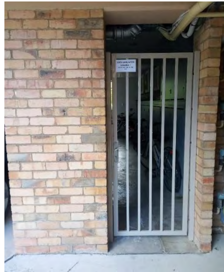
Figure 17. Doorway to bike room. (Source: GML Heritage 2021)
