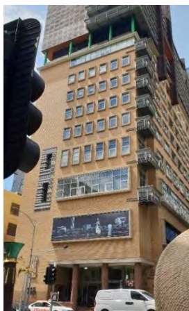
Figure 6. 114–120 Russell Street, built in 1948–1954. (Source: Context 2020)
