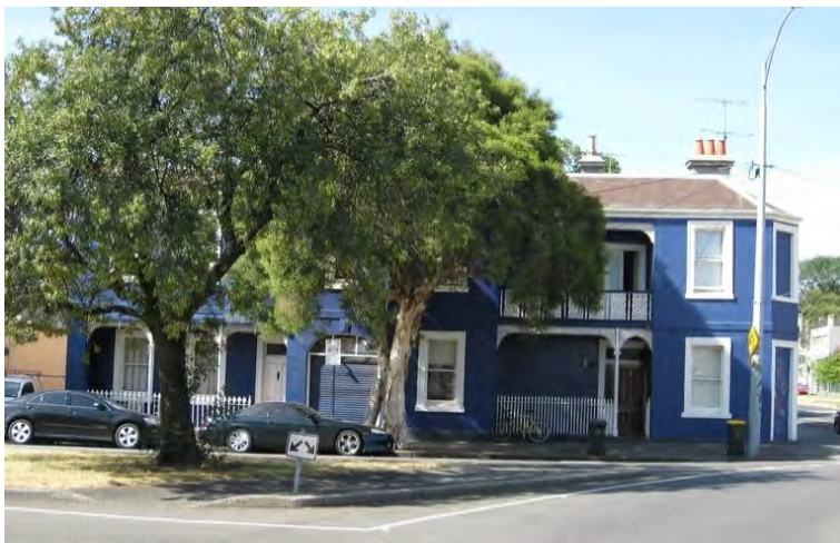
Figure 12. Former Dove Hotel, 55–61 Faraday Street, Carlton, built in 1867. (Source: CoMMaps)
