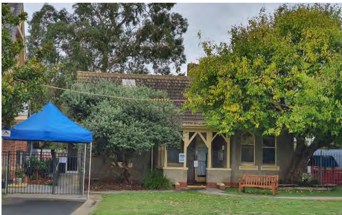
Figure 13. Former caretaker's cottage (Figure 7: Number 6) built in 1925. Note the decorative timberwork to the front porch and the pointed arched windows on the projecting wing on the right-hand side. (Source: GML Heritage 2021)
