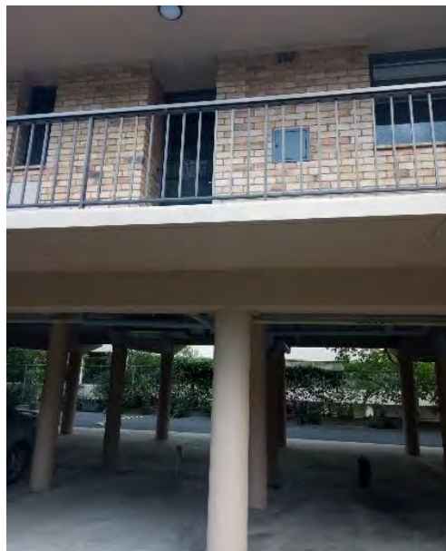
Figure 12. Metal balustrade to galleries above pillar to first floor base. (Source: GML Heritage 2021)
