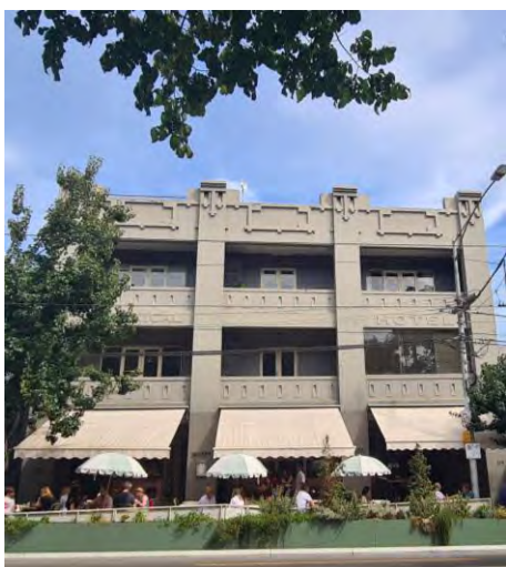
Figure 16. 161–173 Domain Road, South Yarra, built in 1924. (Source: GML Heritage 2021)
