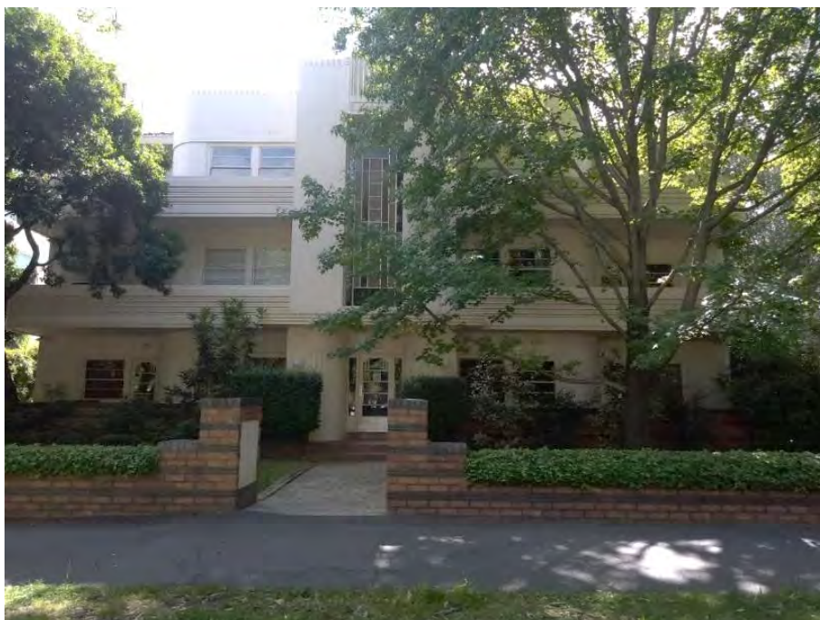
Figure 8. Western façade, facing St Kilda Road, showing front fence with contrasting face brickwork with horizontal stripe patterning. (Source: GML Heritage 2021)
