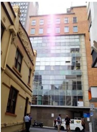
Figure 8. 376–382 Flinders Lane, built in 1956. (Source: Context and GJM 2020)
