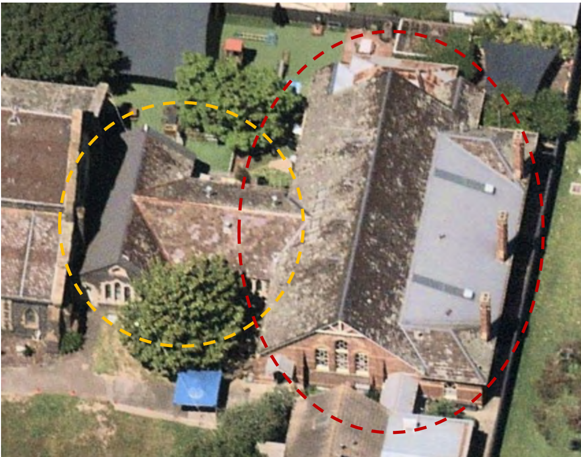
Figure 9. Bird's-eye view of the 1874 vestry and school wing built of bluestone (outlined in yellow, Figure 7: Number 3) and the 1884 Sunday school building built of brick (outlined in red, Figure 7: Number 4). (Source: Nearmap 2020)
