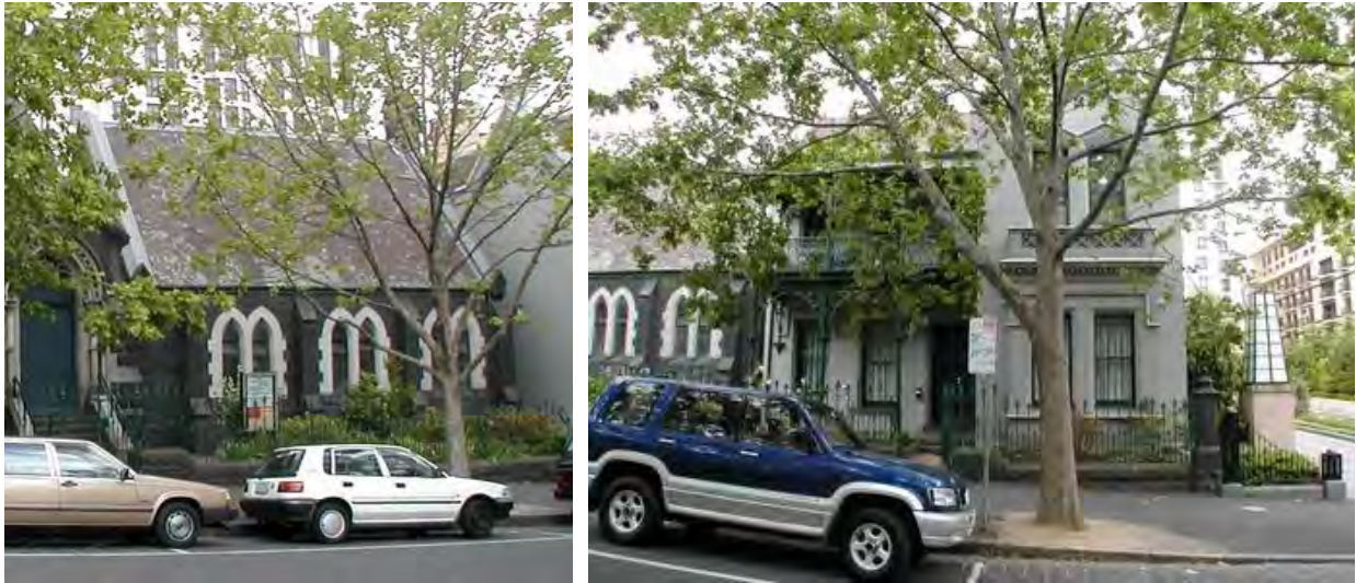
Figure 14. Lutheran Trinity Church Hall, built in 1864 (left), and vicarage, built in 1890 (right). (Source: CoMMaps)
