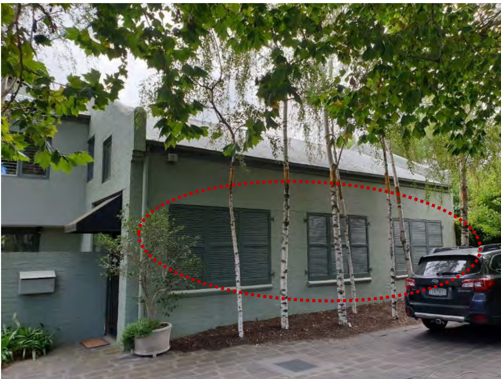
Figure 20. The former engineers workshop, built in 1923, retains its overall industrial form and original window openings (outlined in red) on the east elevation. Other openings appear altered. (Source: GML Heritage 2021)
