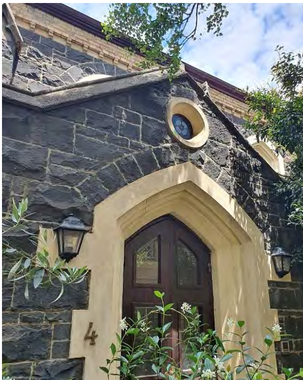
Figure 8. Bluestone porch on the north elevation, featuring a secondary entrance with four centred arch and a rosette window above. (Source: GML Heritage 2021)
