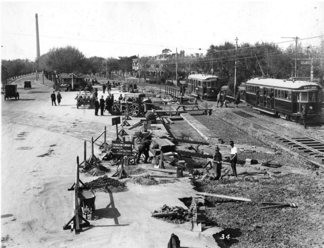
Figure 3.66 Electric tramlines being installed on St Kilda Road, looking towards the city, c.1925. (Source: State Library Victoria, Accession No. H40275/22)
