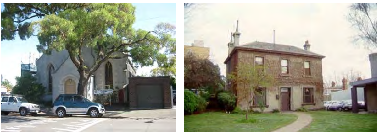
Figure 17. Former Presbyterian Union Memorial Church Complex (North Melbourne) showing hall, built in 1879 (left) and manse, built in 1868 (right). (Source: CoMMaps; Victorian Heritage Database)
