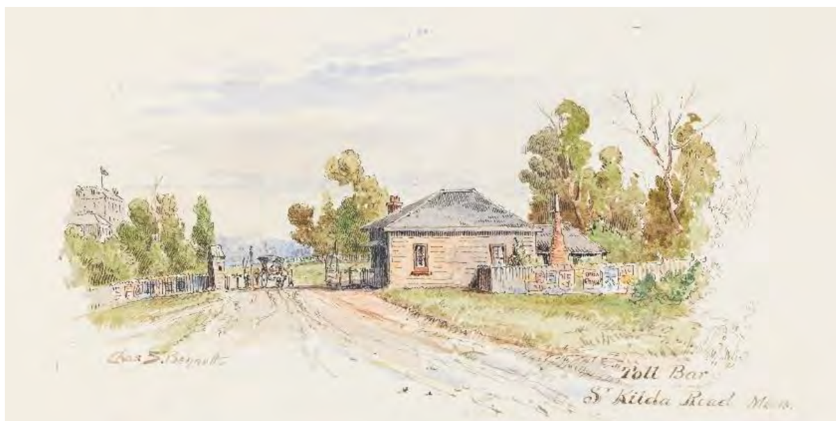
Figure 3.58 Toll booth, St Kilda Road, looking towards town, painted by Charles Bennett, [n.d.], c.1880s. (Source: State Library of New South Wales)
