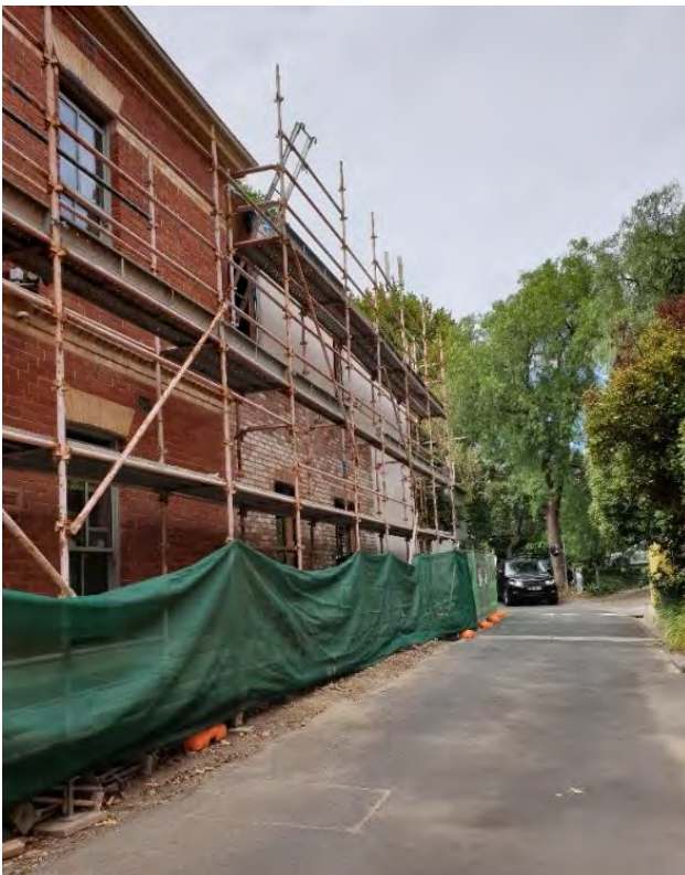
Figure 11. Side elevation of 114 Millswyn Street, with original face brick wall with intact openings (left-hand side) and rear additions being added. (Source: GML Heritage 2021)
