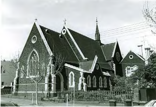
Figure 11. 53–63 Queensberry Street, Carlton, built c1854–65 and altered in 1871 and 1887 to a design by Leonard Terry. (Source: National Trust 1989, via Victorian Heritage Database)
