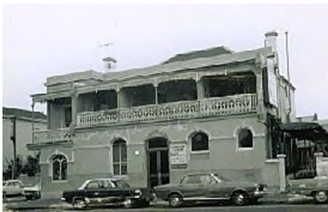
Figure 6. Fawkner Club Hotel (not dated but c1970s). Note that the entrance opening has been widened and the arch form changed to shallower, segmental arch. (Source: National Trust of Australia (Victoria), file B2947)
