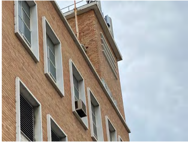
Figure 4. Punt Road façade, detail showing the second floor, tower and moulded grill. (Source: GML Heritage 2021)
