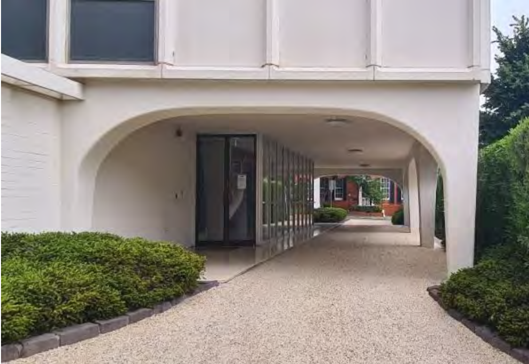
Figure 3. Entry portico. (Source: GML Heritage 2021)
