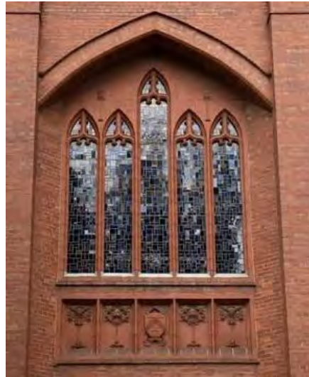
Figure 12. Detail showing stained glass windows, terracotta panelling, and fine brickwork. (Source: GML Heritage 2021)
