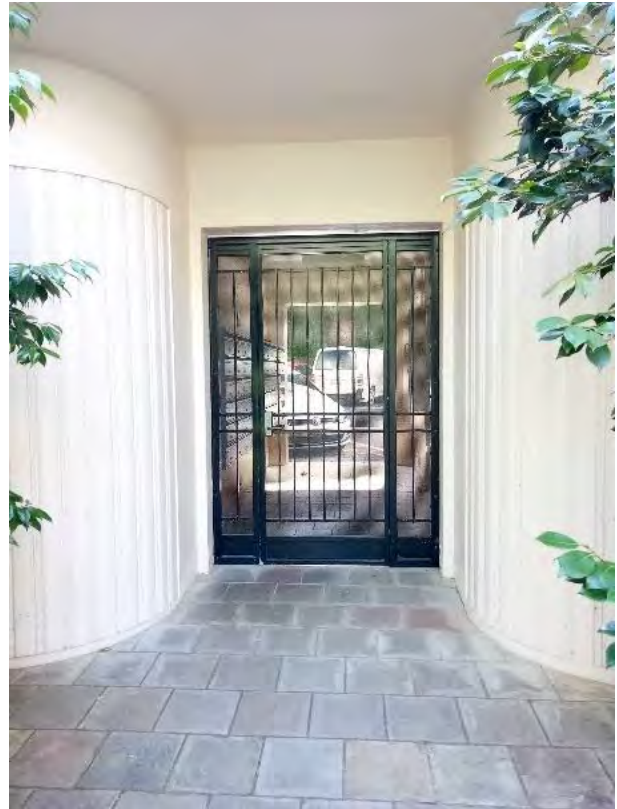
Figure 17. Recessed bay entrance to the carpark with curved walls featuring vertical ribbing. (Source: GML Heritage 2021)
