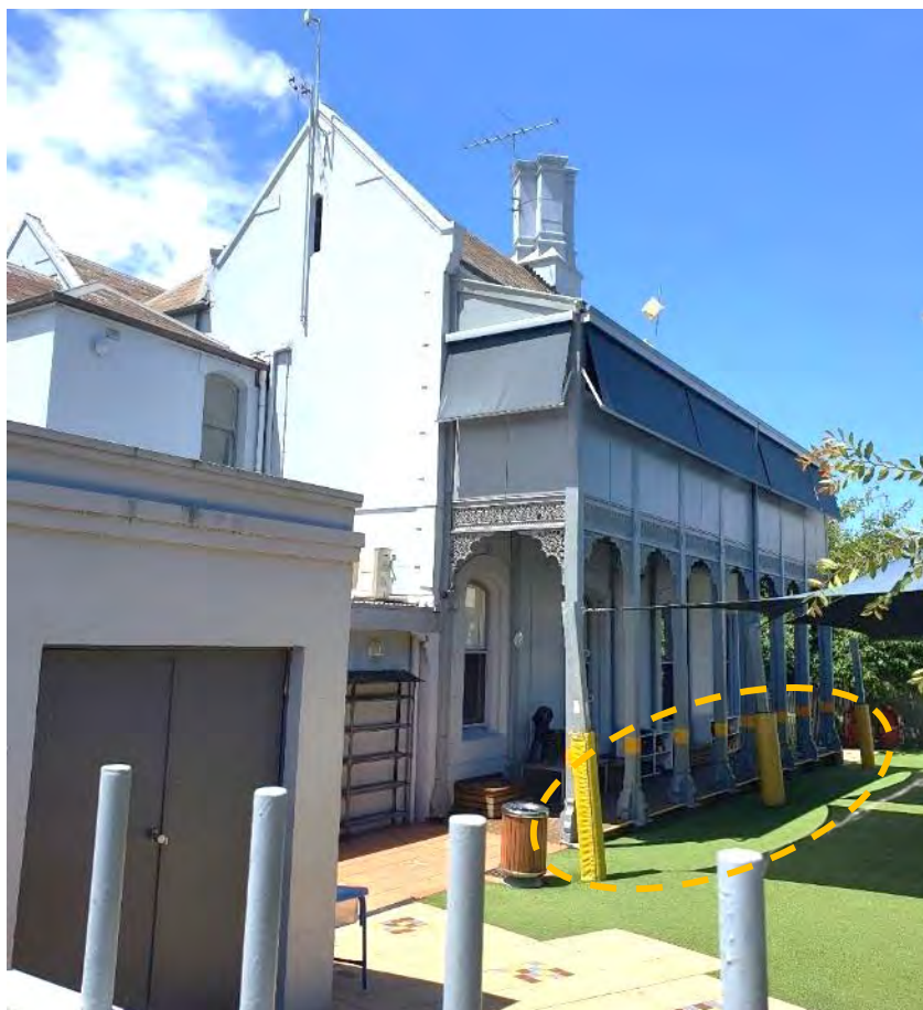
Figure 12. View of the former manse (Figure 7: Number 2) from Park Place. Note the timber verandah with decorative ironwork and base (outlined in yellow). (Source: GML Heritage 2021)
