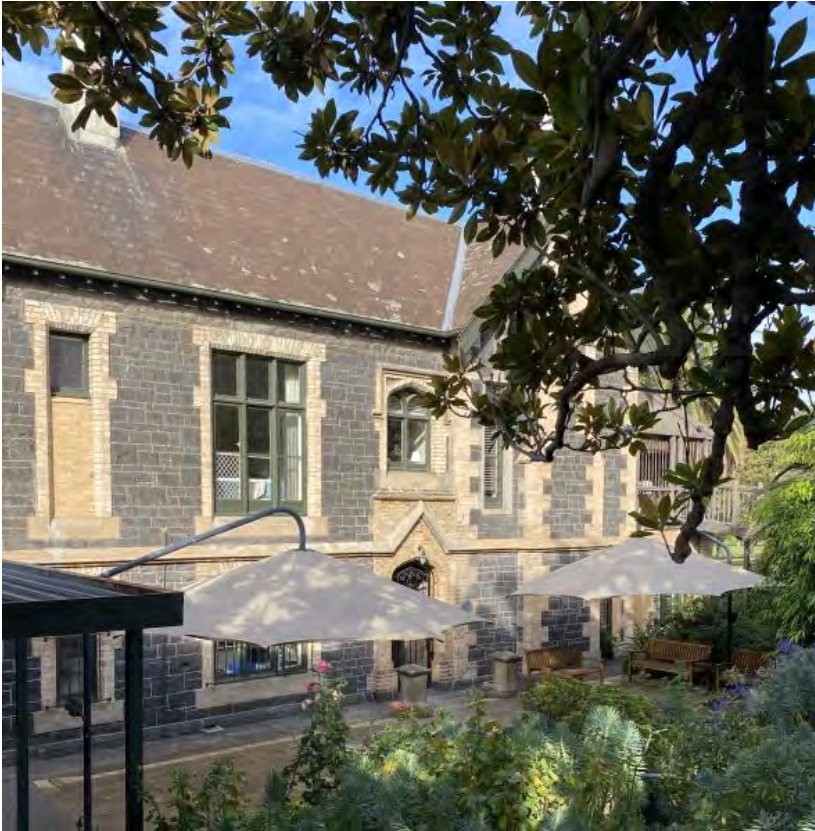
Figure 9. A view of the northern elevation of the Vicarage. The height of the first floor against the ground floor is evident. Note the bricked up window to the left. (Source: GML Heritage 2021)
