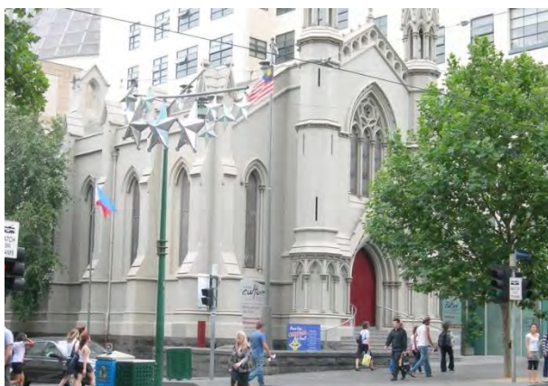
Figure 13. 327–333 Swanston Street, Melbourne, built in 1863 to a design by Charles Webb. (Source: Victorian Heritage Database)
