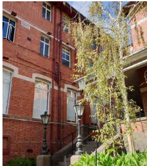
Figure 18. Phelia Grimwade House extension, side elevation facing west. (Source: GML Heritage 2021)
