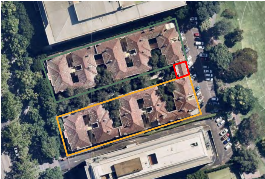
Figure 7. Aerial image of the building in 2020 showing block 447 (outlined in orange), block 453 (blue) and the interconnecting element at the rear (red). (Source: Nearmap 2020 with GML overlay)
