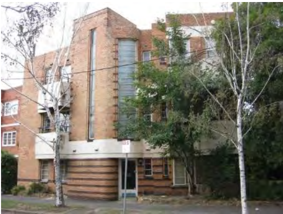
Figure 24. 2–4 Garden Avenue, East Melbourne, built in 1930. (Source: CoMMaps)
