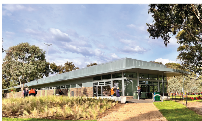
Landscaping in front of the pavilion is complete
