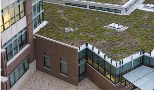
Figure 21. William A. Jones III building, Joint Base Andrews, Maryland, USA can reduce runoff by 65% and cool roof by 35–40%.
